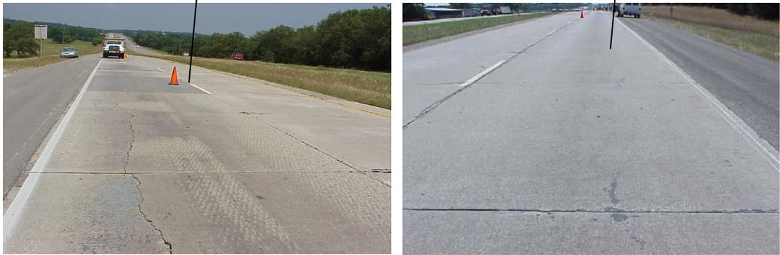
b) Pavement condition in the distressed and non distressed area
