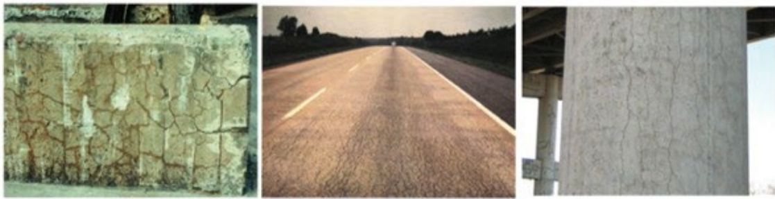
Figure 11.4: Concrete Structures Affected by ASR [2]
