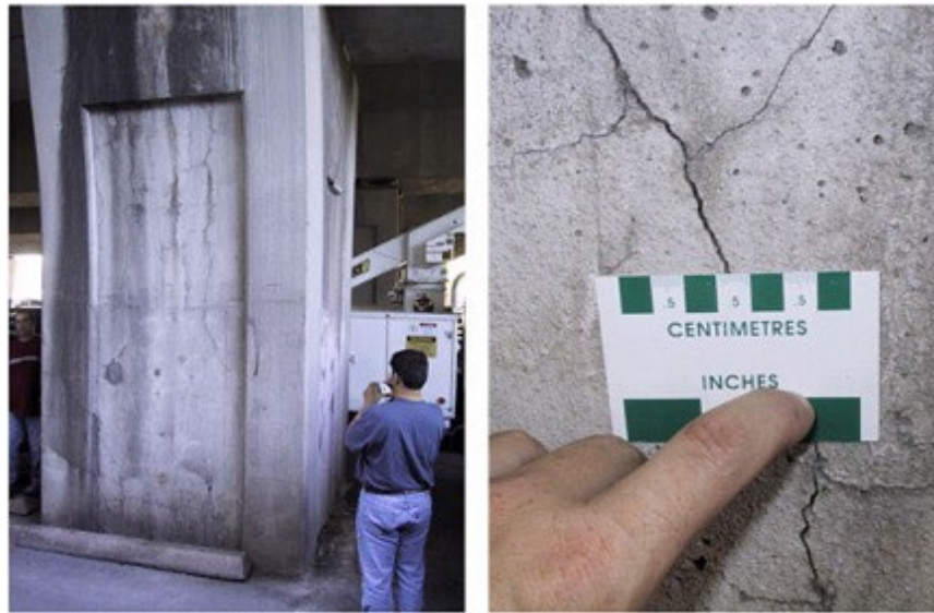
Figure 11.5: Concrete Structures Affected by DEF. [12]
