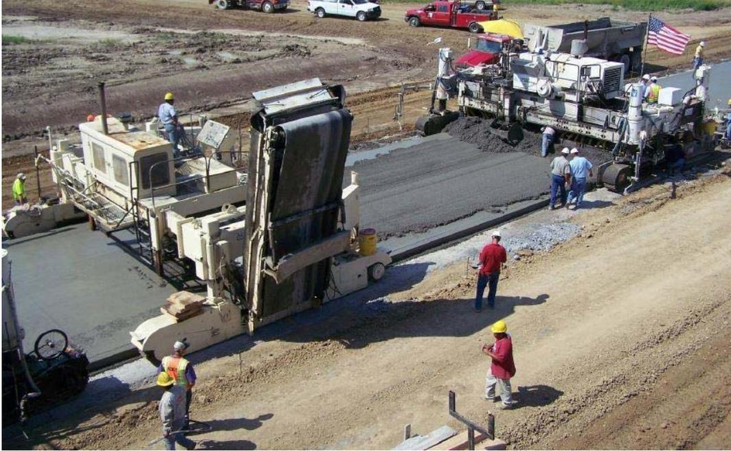
**Figure 20. 2LCP construction in Kansas I-70 Project (Gerhardt 2013).**
