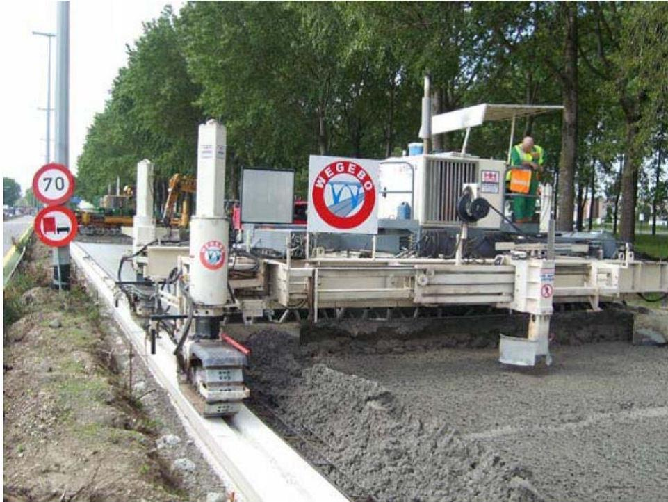
**Figure 19. CRCP Construction in E34 Motorway Construction (Ren 2008).**
