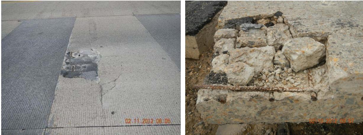
**Figure 8. Two-Lift Pavement Delamination on I-30 at Sulphur Springs, TX
