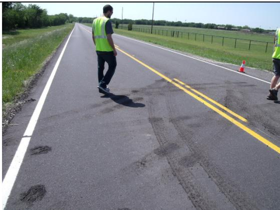
Tear marks (bottom left) from power to rear tires damaging the microsurfacing. The microsurfacing was still slightly soft when visited 5-6 months after construction. Demonstrates importance of creating an adequate mix design to ensure proper curing.
