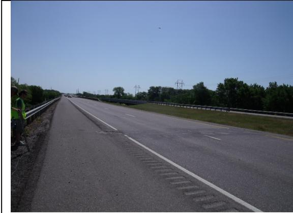
One of only two significant distresses in the microsurfacing. Occurred at the beginning of an embankment constructed for a bridge. Settlement of the fill was the obvious cause of failure of the base pavement which reflected through the microsurfacing.
