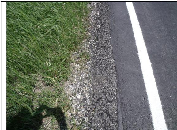
Well constructed edges on pavement with good macro-texture. Microsurfacing had good micro-texture.
