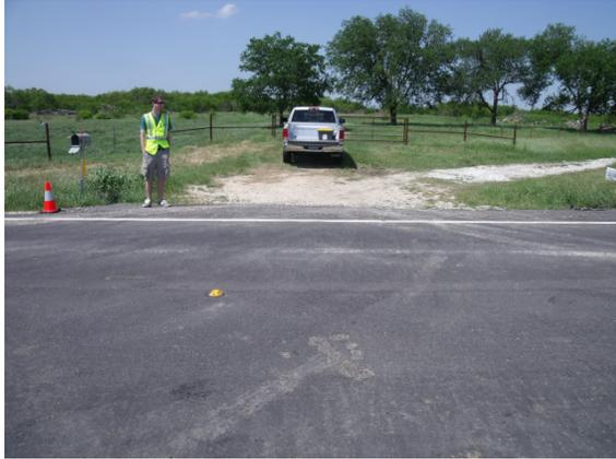
Delamination seen in intersections. In this case, entrance and exit of landowner immediately prior to paving may have introduced dust onto the surface and prevented adequate bonding.
