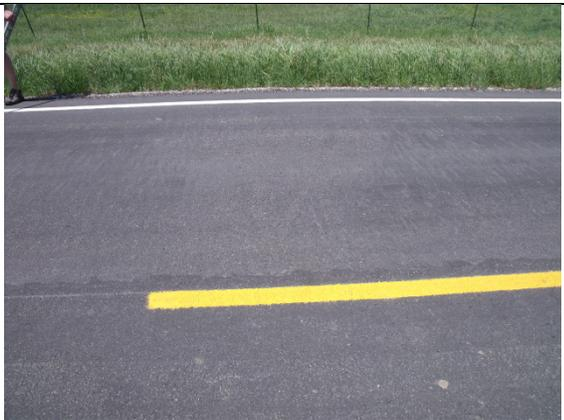
Also present in this project was high frequency, low amplitude corrugation as seen on the left of the top lane. Rough pavement underneath reflecting through or causing the rear strikeoff to “jump” is the most likely cause of this. Demonstrates importance of meeting the requirements in Table 4-1.
