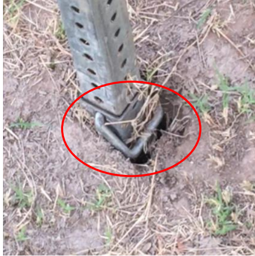
a. The hole (the gap between the metal post and the earth) caused by the constant traffic sign trembling
