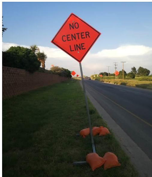
(b) Sign 1003: H-base Single Upright with Leg PSST Skid Sign
