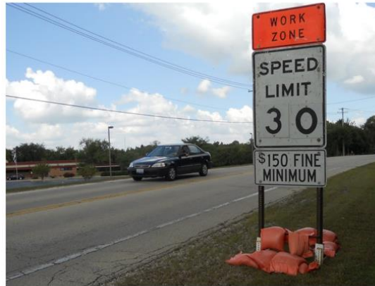
Figure 14. Sandbags on skid as ballast to resist high speed wind forces
