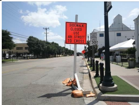
(a) Sign 1000: Wooden Skid with 2 Wooden Legs Sign
