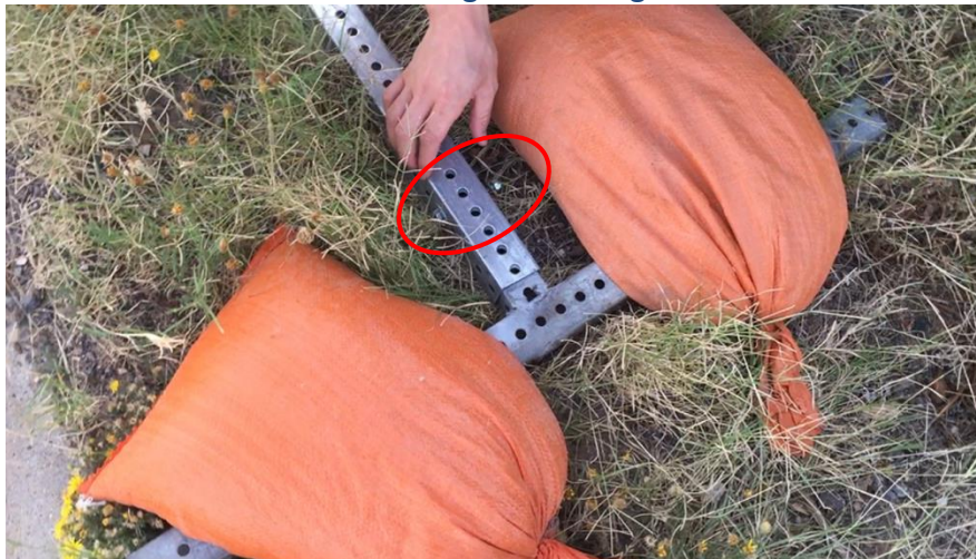
b. The loosened nut resulted from the constant trembling of the supported traffic sign Figure 50. Performance Checks of Traffic Signs in Midland, TX
