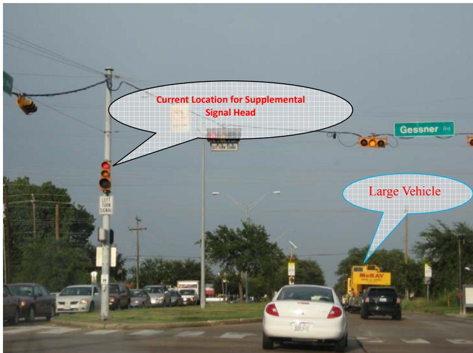
**Figure 15** Current Supplemental Left-Turn Signal Head for Intersection at Bellaire Blvd & S Gessner Rd in Houston, Texas.
