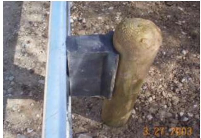
**Figure 4 Tire Rubber Guardrail Spacer**
