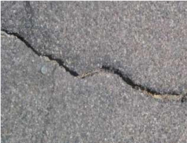
**Figure 12 Typical Thermal Crack**
