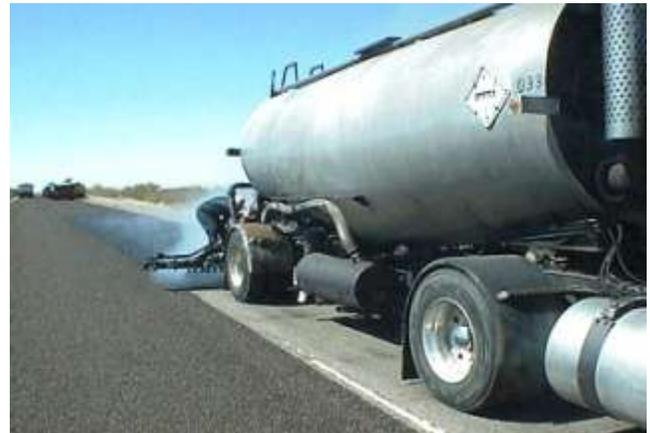
**Figure 13 Agitating Spreader Truck**
