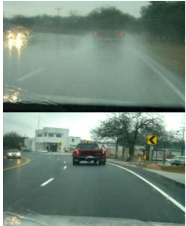
Figure 7 Wet Weather Conditions Before and After A-R Overlay
