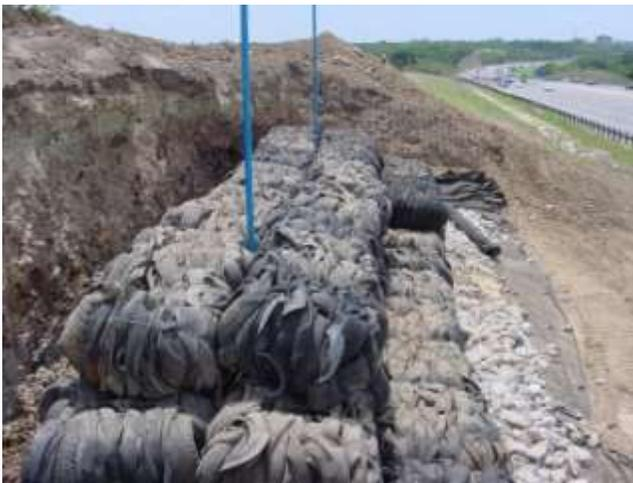
**Figure 3 Tire Rubber Roadside Embankment**
