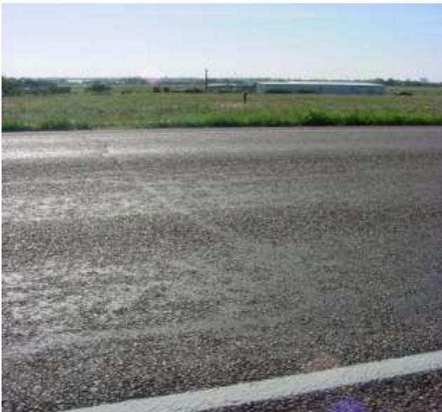
**Figure 10 Seal Coat with Stress Absorbing Layer in Foreground - without Layer in Background**
