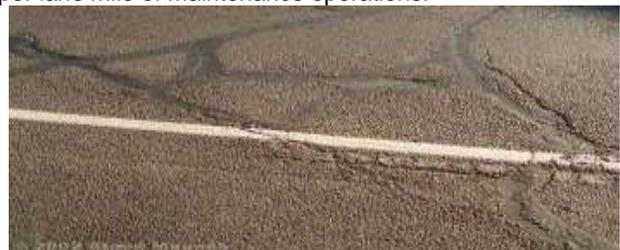
**Figure 9 Crack Seal**
