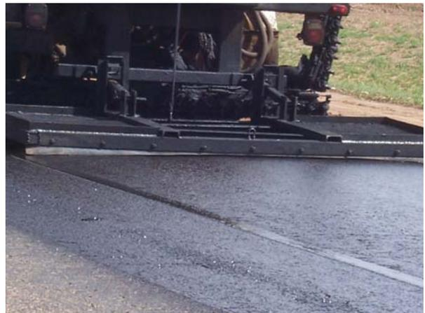
The material's relatively quick curing time, within an hour to an hour and a half in the West Texas wind and heat, allows traffic to be put back on the roadway fairly quickly. Though this method is not nearly as effective as
