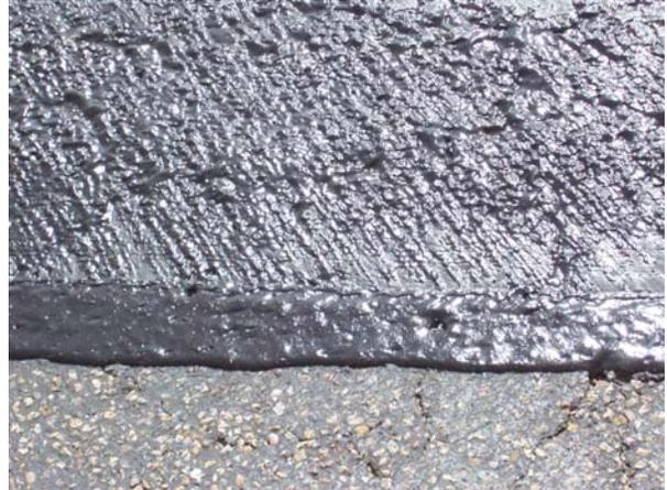
A tire rubber modified surface sealer, which contains 10 percent tire rubber emulsion, is being used on a project in the Lubbock District's Crosby County to pre-treat a 12-mile section of FM 207.
