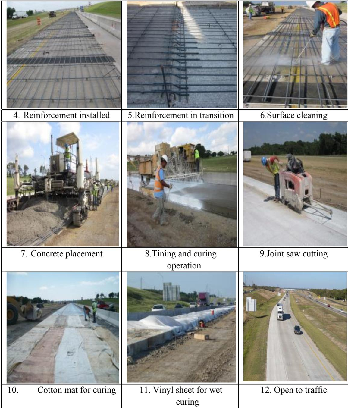
Figure 3.1 Construction sequence of CRCP BCO
