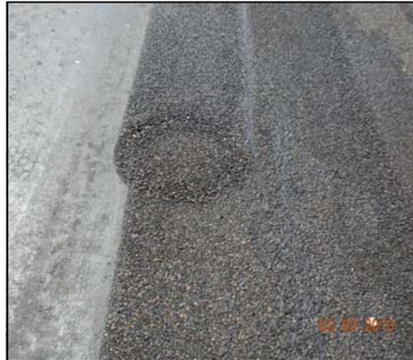
**FIG 38.** Pavement damage due to stationary spray-bar rotation.
