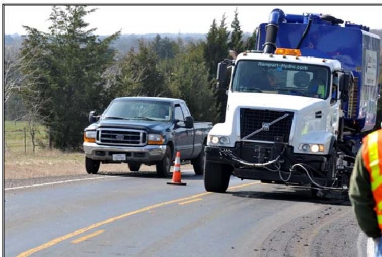
**FIG 30.** UHP Water Cutting in the Outside Wheel Path on Two-Lane Roads Requires A Full Lane Closure. *Image courtesy TTI Visual Media.*
