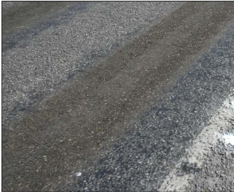
**FIG 39.** Inadequate treatment in the middle of the wheel paths, resulting from a non-uniform pavement surface (rutting).
