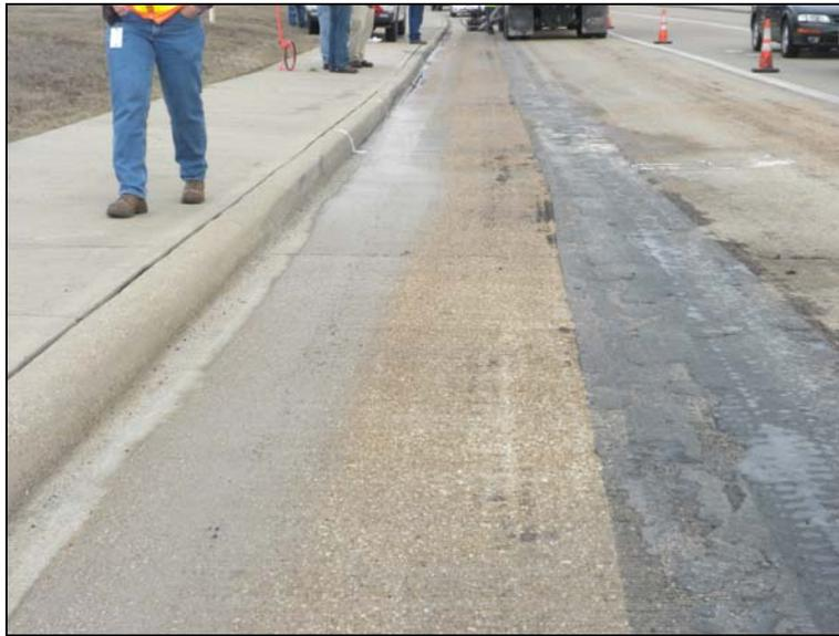
**FIG 25.** UHP water cutting can be used to remove tracked asphalt from concrete pavement.
