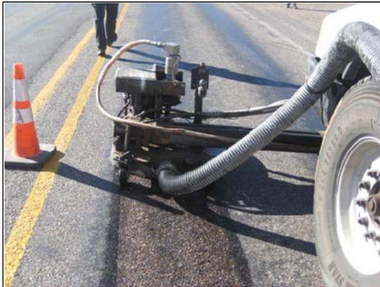
**FIG 23.** Restoration of texture to flushed pavements with a seal coat or surface treatment is the primary maintenance application for UHP water cutting.
