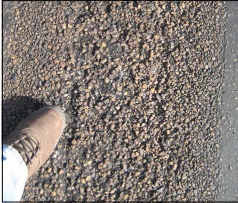
Figure 37 shows damage to the pavement surface associated with an overly aggressive nozzle configuration.
