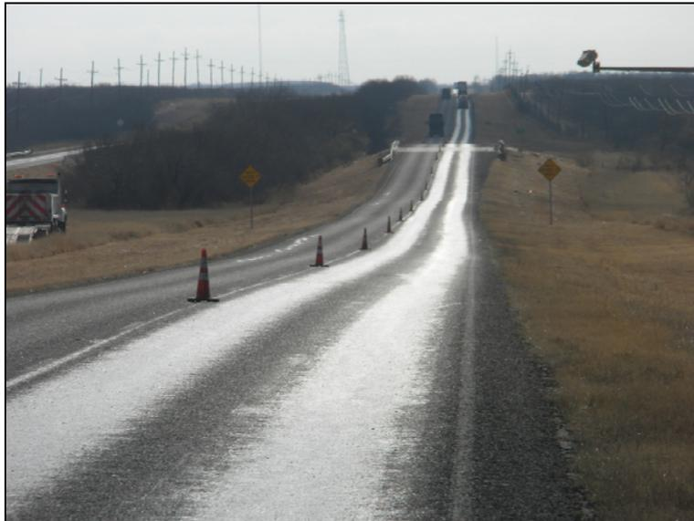
**FIG 6.** This heavily-flushed FM road in Webb County, TX was treated using the UHP water cutting process.
