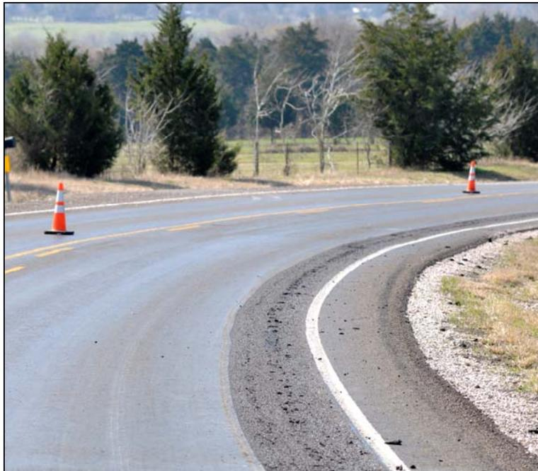
**FIG 24.** UHP water cutting can be used to treat heavily flushed roads in advance of a scheduled seal coat. *Image courtesy TTI Visual Media.*
