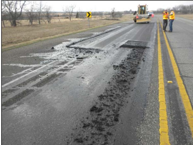
**FIG 35.** Waste debris and water remaining on the pavement surface when the vacuum system is not functioning properly.
