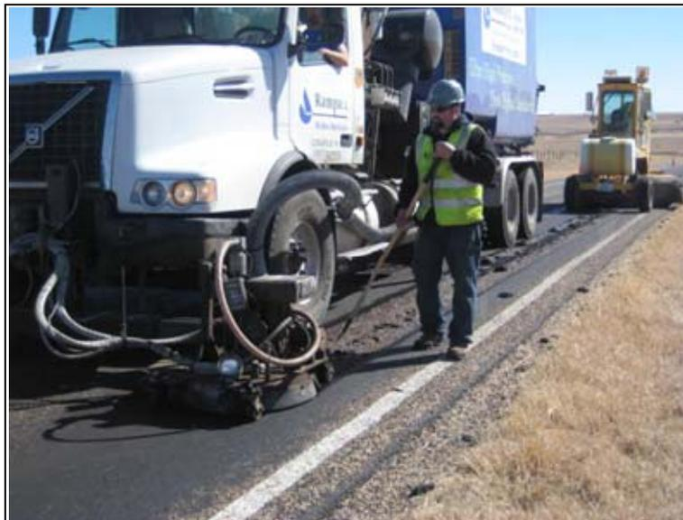
**FIG 36.** Hand-scraping of excess asphalt lumps, cut but not vacuumed from the pavement surface.
