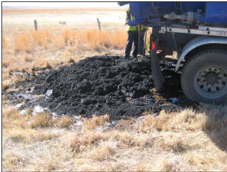
**FIG 15.** Temporary dumping of UHP water cutter waste debris along the roadside for later pickup and removal.
