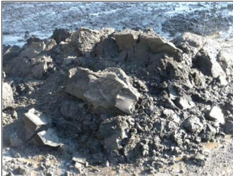
**FIG 14.** The UHP water cutting operation removes both solids and water from the road surface.
