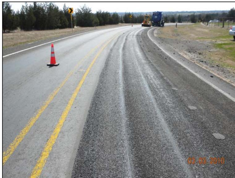
**FIG 2.** UHP water cutting, multiple passes for continuous treatment of the lane, Bryan demonstration project, March 2010.
