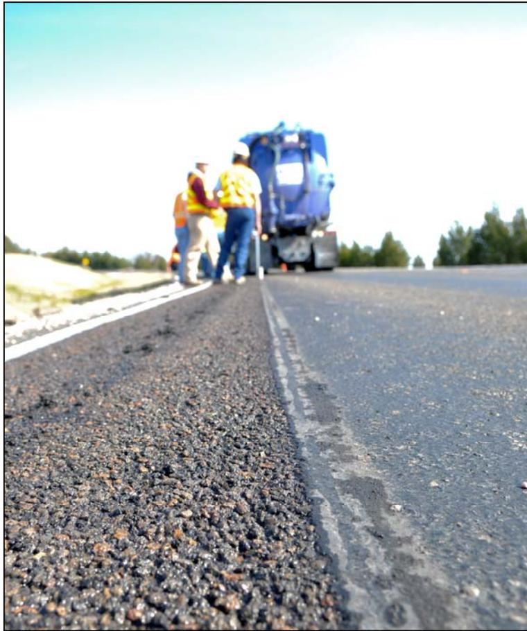
**FIG 29.** UHP water cutting is a promising maintenance tool for treatment of flushed pavements. *Image courtesy TTI Visual Media.*
