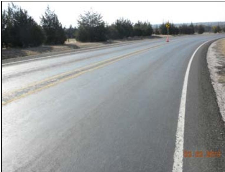
**FIG 1.** Flushed pavement, UHP demonstration project, Grimes County, TX (Bryan District).
