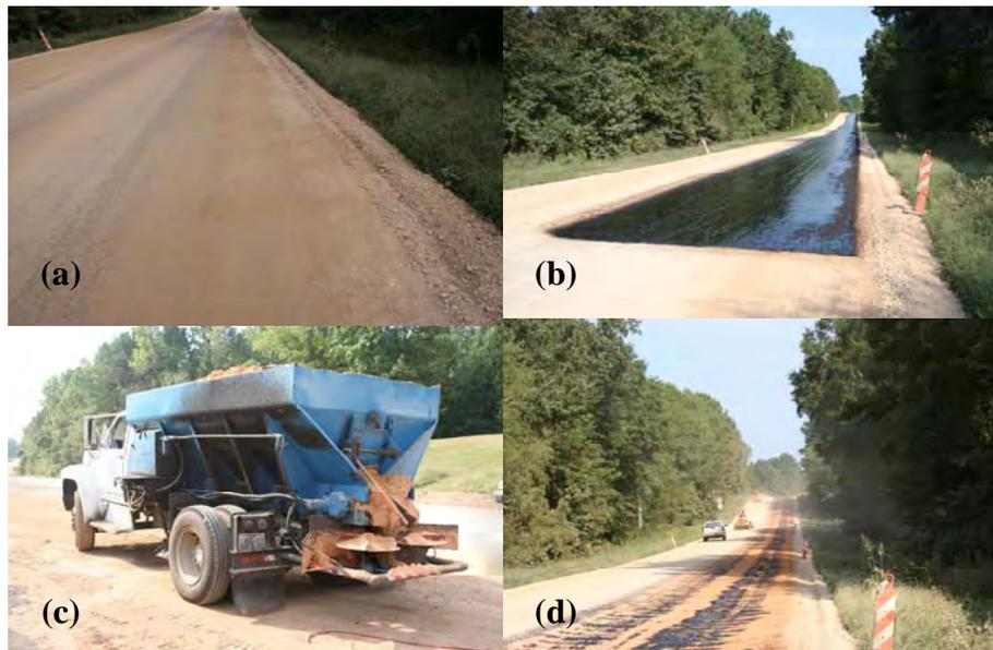
**Figure 5.3** Spraying Prime on Limestone Flexible Base (a) Finished With IRI of 112, (b) Spray Prime Applied (c) Fertilizer Spreader Used to Spread Field Sand for Blotting, and (d) Brooming of Blotting Sand to Finished Lane
