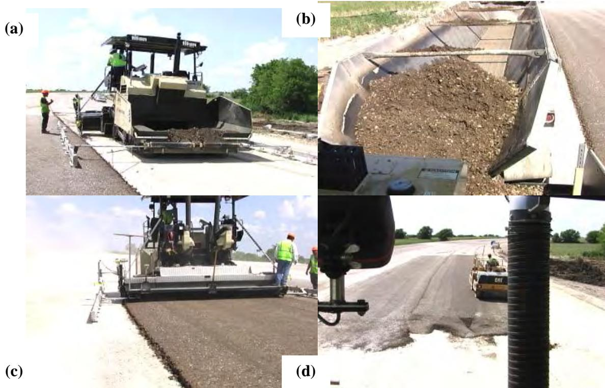
**Figure 5.10** Base Lay-Down Machine in Operation (a) Lay-down Machine and its Conveyor – Driven Hopper (b) Mixed Base Material Transported from Pugmill to Lay-Down Machine Hopper (c) Lay-Down of Emulsified Asphalt Base in Progress (d) Rolling of Laid-Down Base
