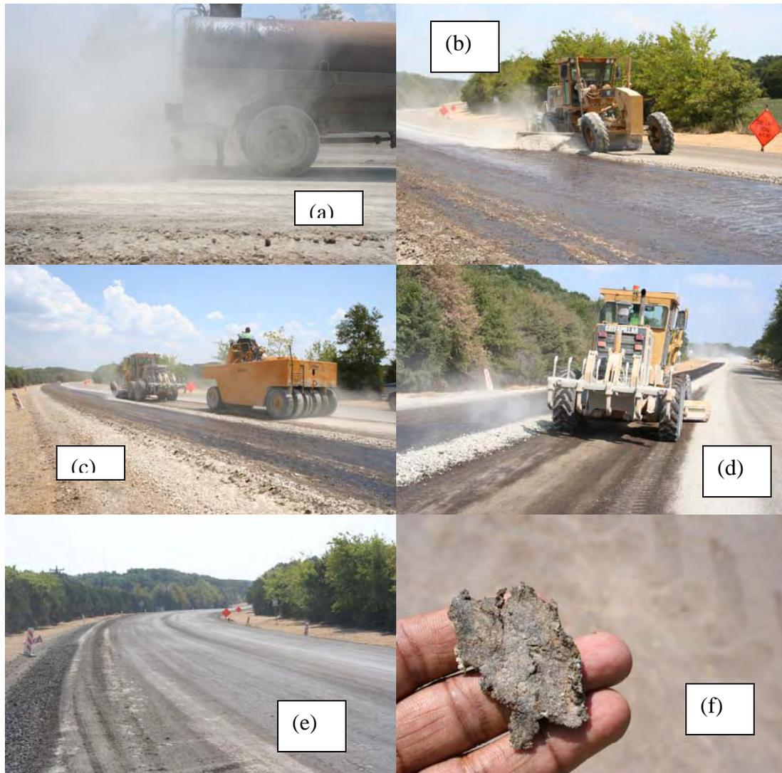
**Figure 5.8** Construction of Two-Course Surface Treatment in East Texas (a) Spraying Diluted SS-1 Emulsion Prime (b) Working-in Base Fines from Windrow (c) Rolling of Fines into the Diluted Emulsion using Medium Pneumatic Roller (d) Application of Second Coat of Prime (e) ‘Painted’ Primed Base Ready for First Course of Surface Treatment (f) Flake of Asphalt-Sand Prime Coat
