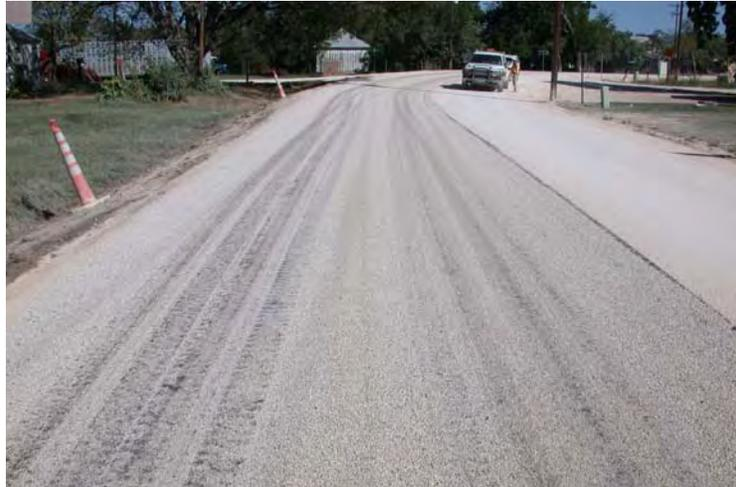
**Figure 4.8** Covered (Or Inverted) Prime Using RC-250 and Grade 5 Rock
