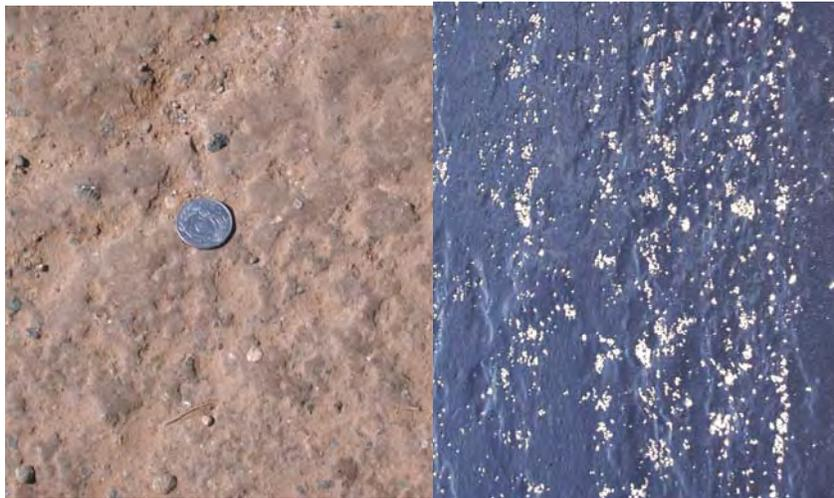
**Figure 4.17** Freckling of Asphalt Applied on Dusty Base
