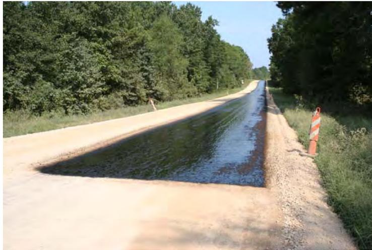
**Figure 4.6** Sprayed Prime Coat on Limestone Base
