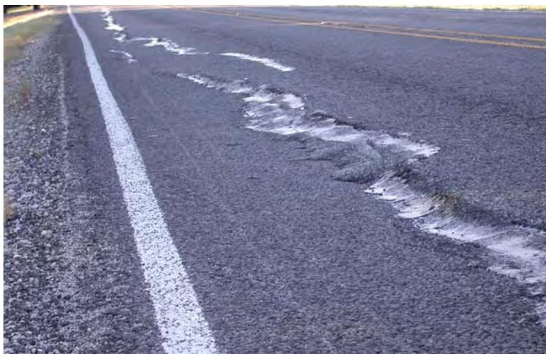
**Figure 4.4** Severe Cracking of Surface Course in a Pavement Built on Expansive Soil
