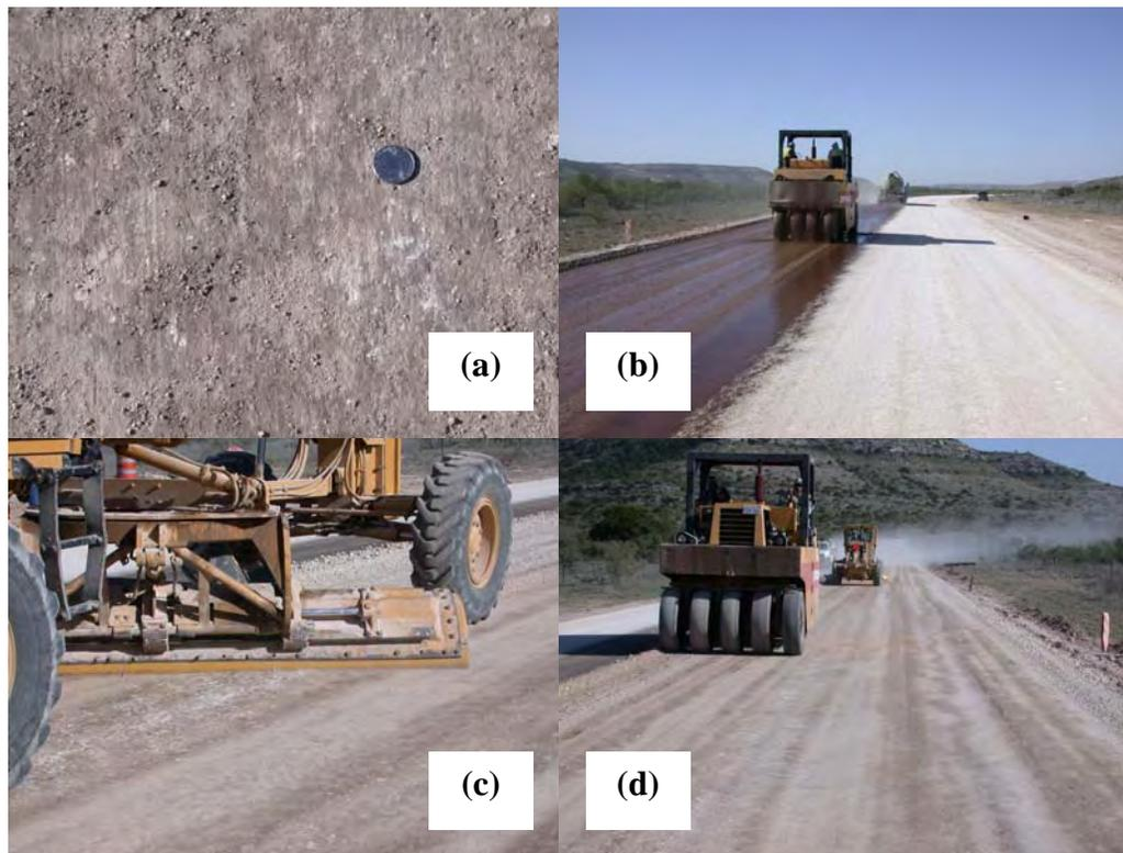
**Figure 5.5** Construction of Two-Course Surface Treatment in West Texas (a) Finished Base Surface before Priming (b) MS-2 Prime Diluted 5% Emulsion/95% Water on Finished Base (c) Base Material Spread over Prime (d) Rolling with Pneumatic Roller
