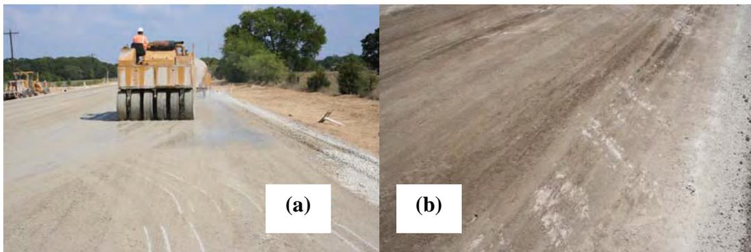
**Figure 5.7** Construction of Two-Course Surface Treatment in East Texas (a) Slush Rolling (b) Bladed Surface Ready to be Primed
