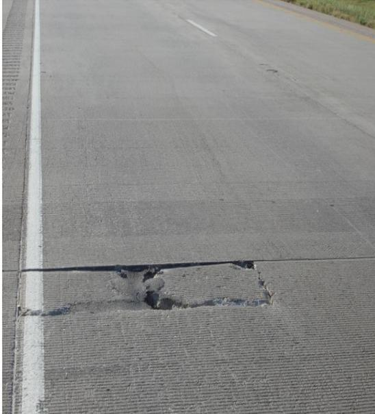
Figure 4-(a) Distress at transverse construction joint
