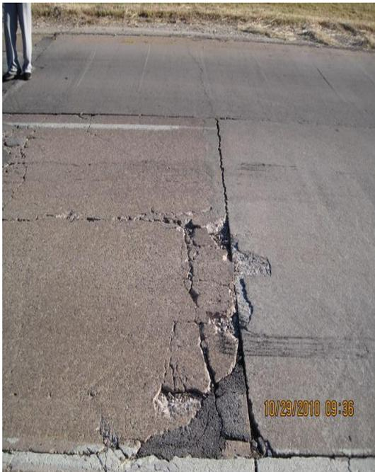
Figure 3-(a) Distress at repair joint
