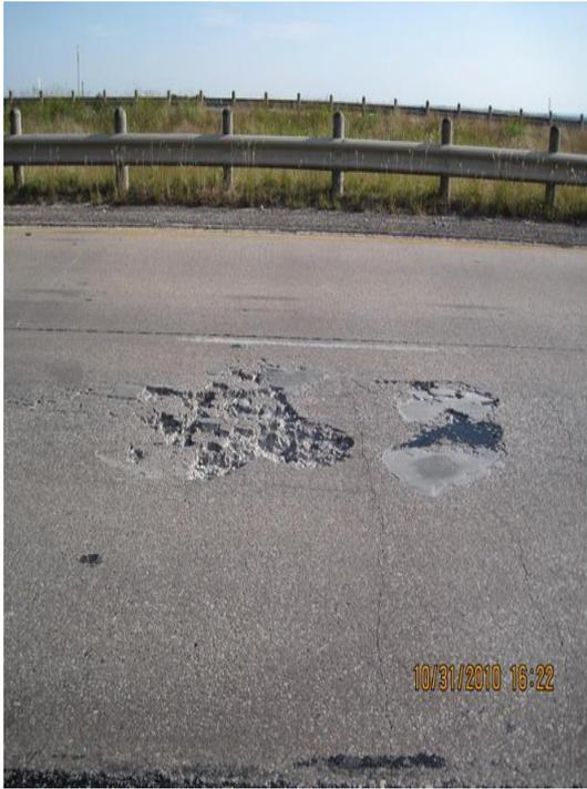
Figure 2-(a) Large surface defect
