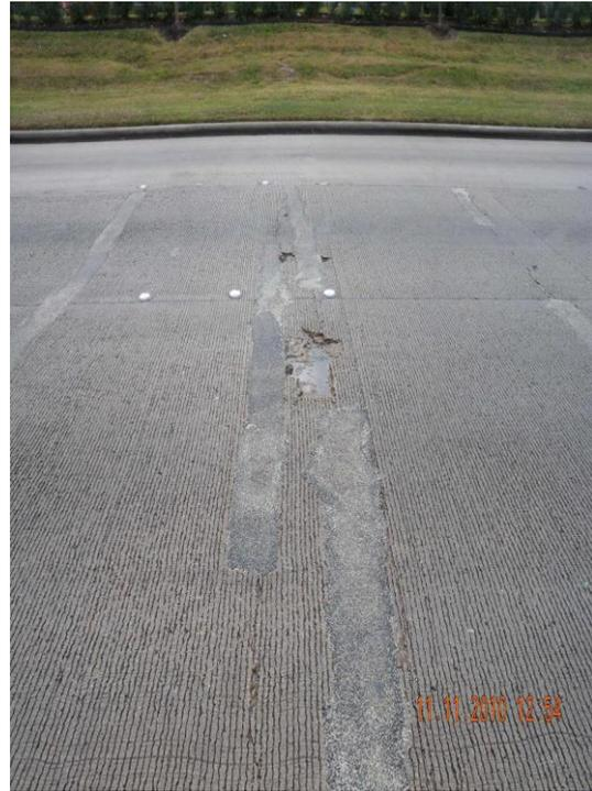
Figure 2-(b) Spalling and repairs
