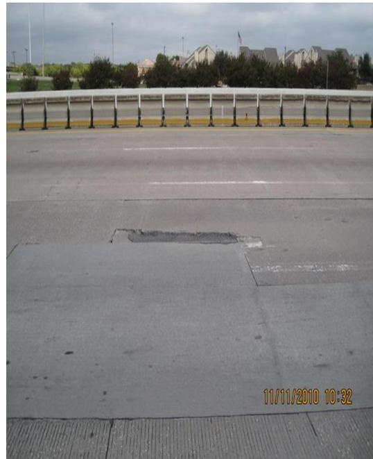
Figure 3-(b) Distress at repair joint
