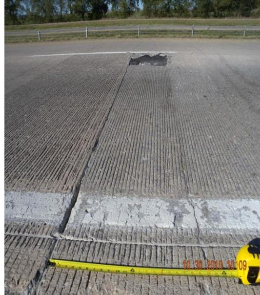
Figure 4-(b) Distress at transverse construction joint
