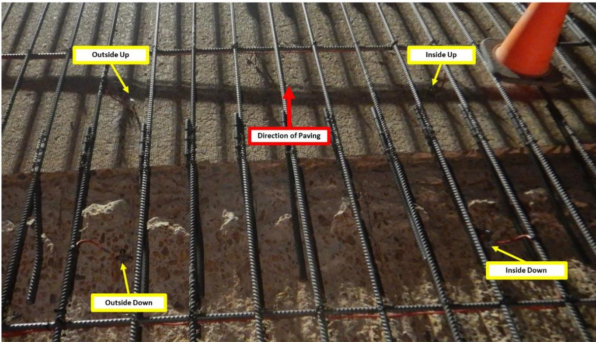
**Figure 41 Field gauge installation of sensors at section 4**
