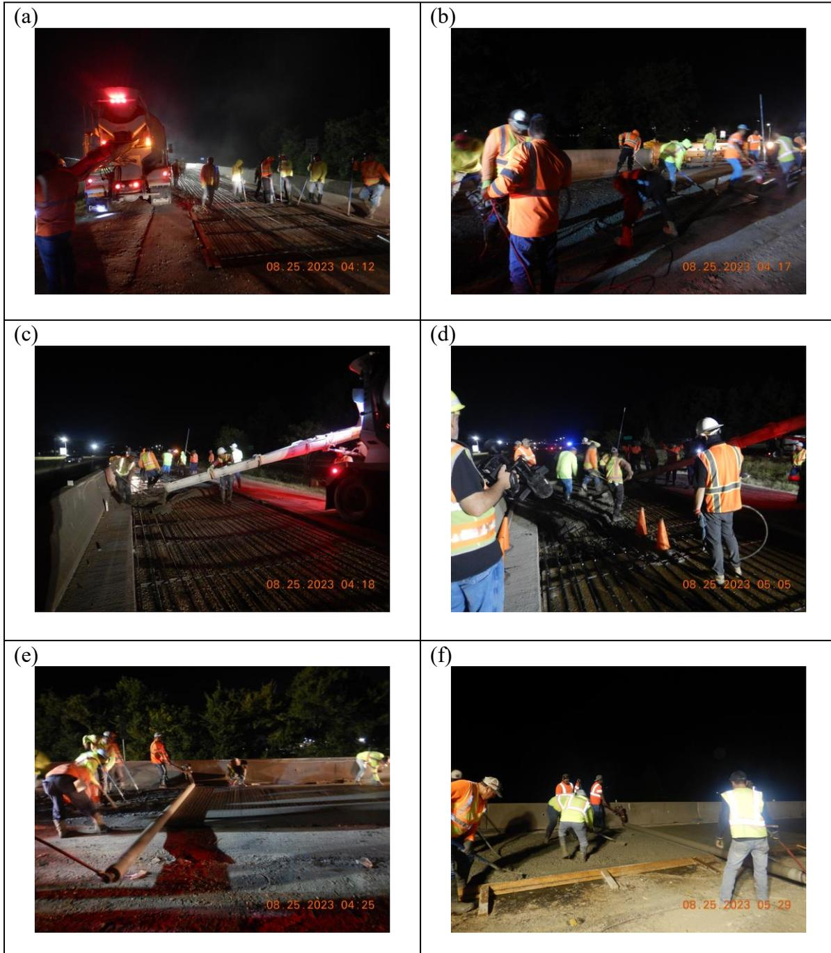
**Figure 48 Concrete placement and consolidation on inside lane**
