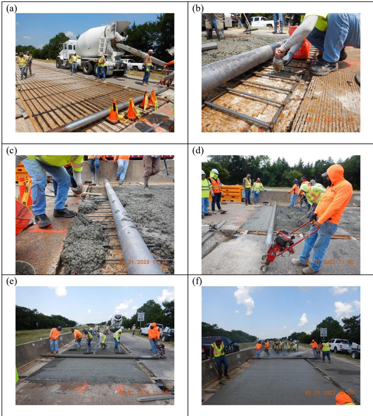
**Figure 43 Concrete placement and consolidation on outside lane.**
