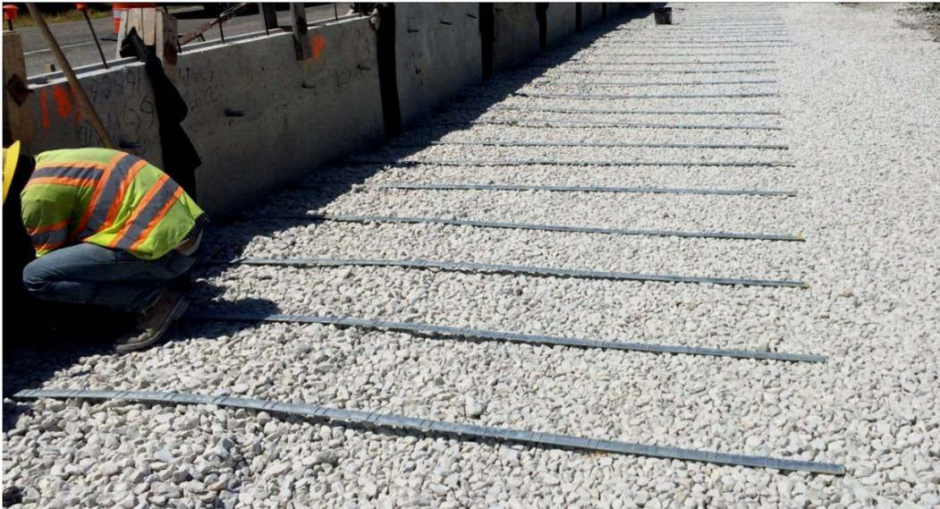
Figure 5.1 Ribbed Strip Reinforcement
