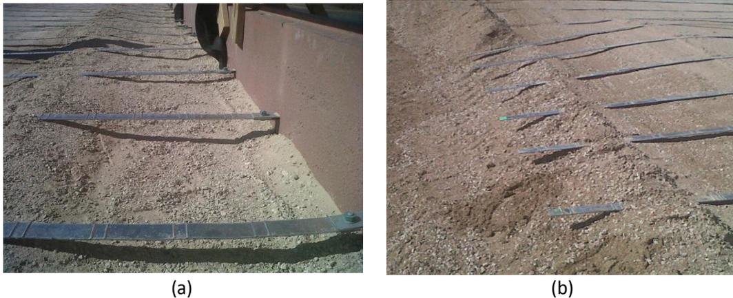
Figure 3.2 Improperly Placed Backfill Providing Non-Uniform Support for Reinforcement
