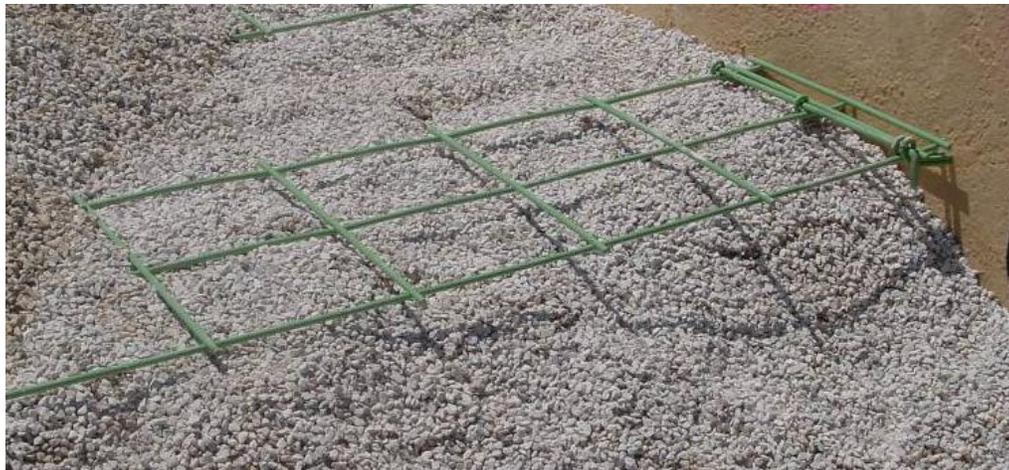
Figure 6.1 3-Wire Grid Reinforcement
