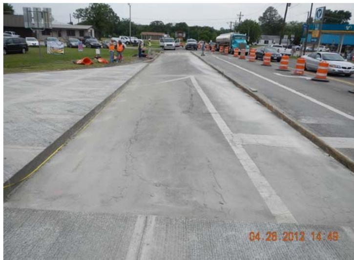
**Figure 3.2 Distress on Existing Asphalt Pavement**
