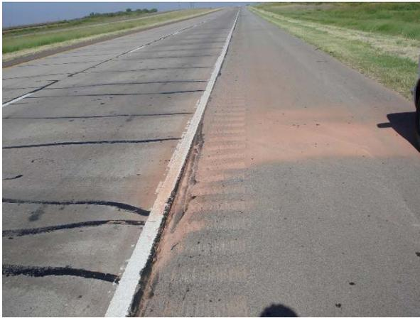
**Figure 4.1 Severe Pumping at The Edge of Pavement with Asphalt Stabilized Base**
