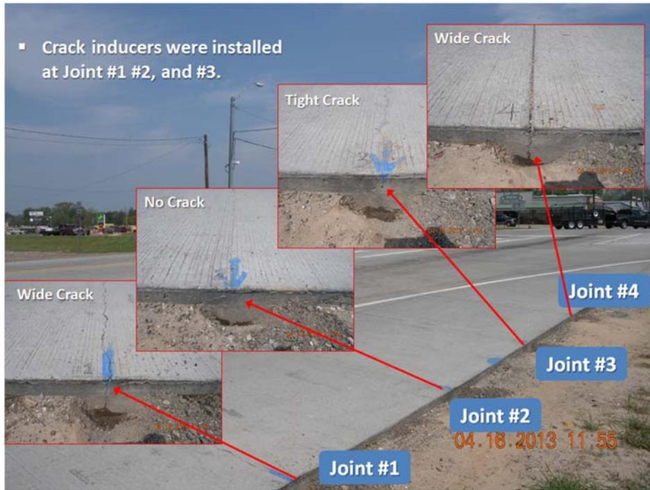
**Figure 3.15 Joints Condition**
