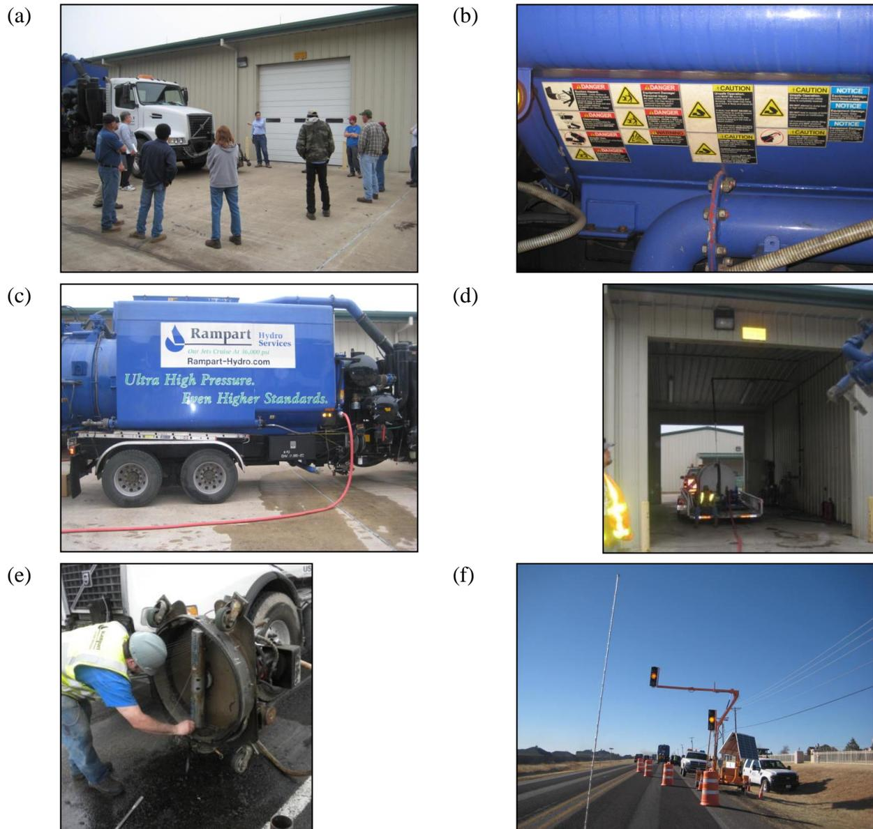
**FIGURE 2.6.** Daily Operations for Ultra High Pressure (UHP) Water Cutter Treatment (a) safety meeting at TxDOT maintenance yard; (b) hazard warnings in the water cutter truck; (c) pumping water into the water cutter truck; (d) getting water to the 4000-gallon water cutter truck - using water trailer when there is insufficient overhead clearance for the truck; (e) adjustment of
