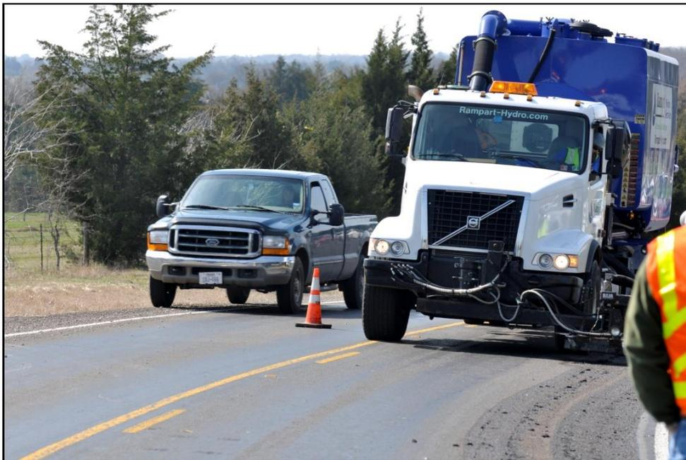
**FIGURE 5.2.** UHP Water Cutting in Outside Wheel Path on Two-Lane Roads Requires Full Lane Closure. *Image courtesy Chris Sasser, TTI Visual Media.*
