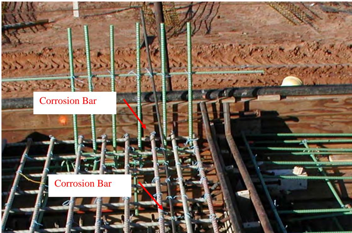
**Figure 3.13** Corrosion Bar at the Sealed Expansion Joint (Discontinuous End) of Span 6, Phase I
