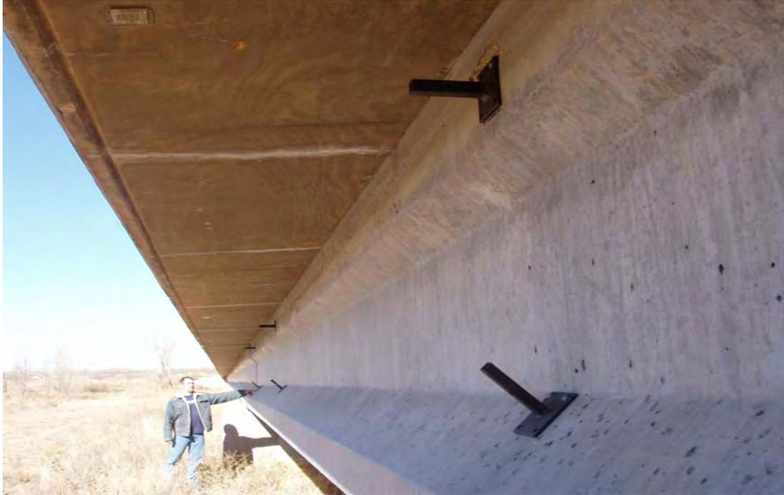
**Figure D.1** LVDT Mounting Brackets on Span 6
