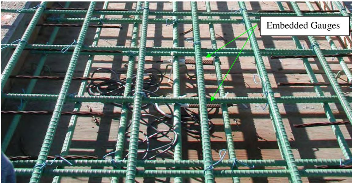
**Figure 3.10** Embedded Gauges in the Controlled Joint Between Spans 1 and 2
