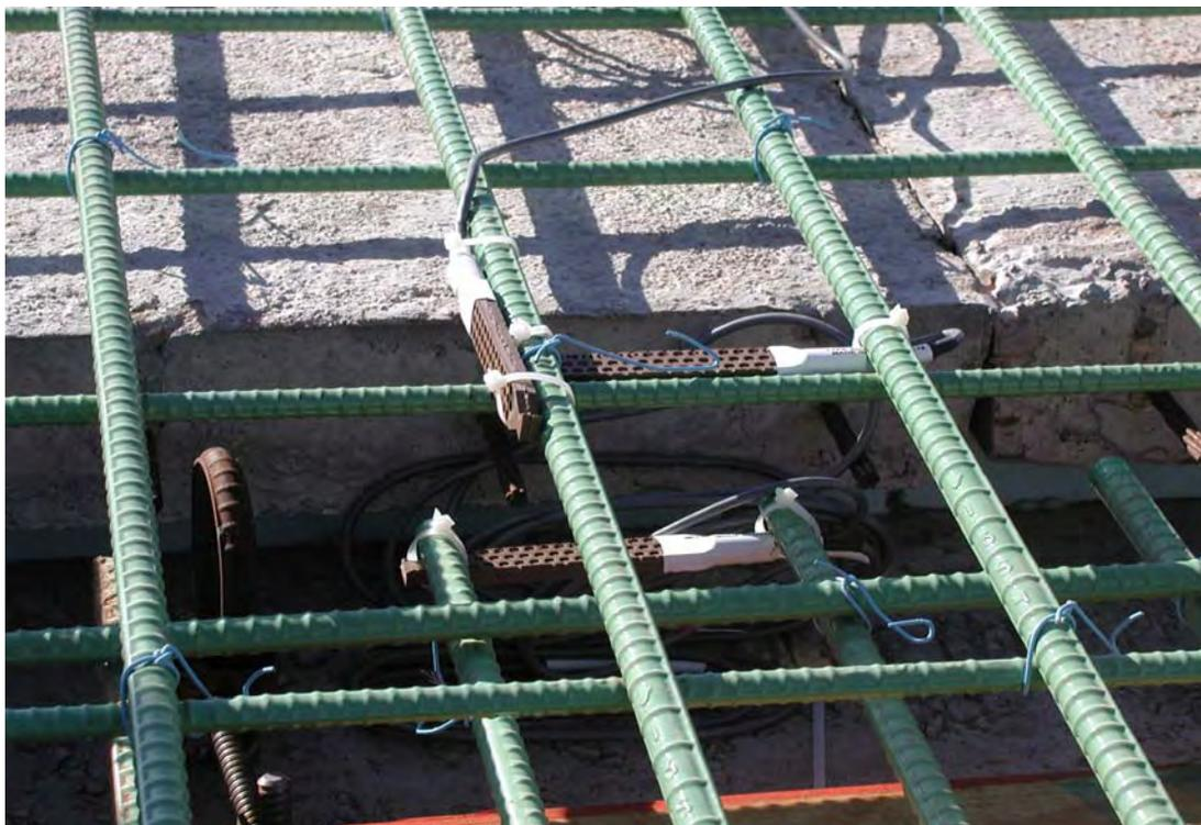
**Figure 3.4.** Embedded Concrete Strain Gauges Over an Interior Beam
