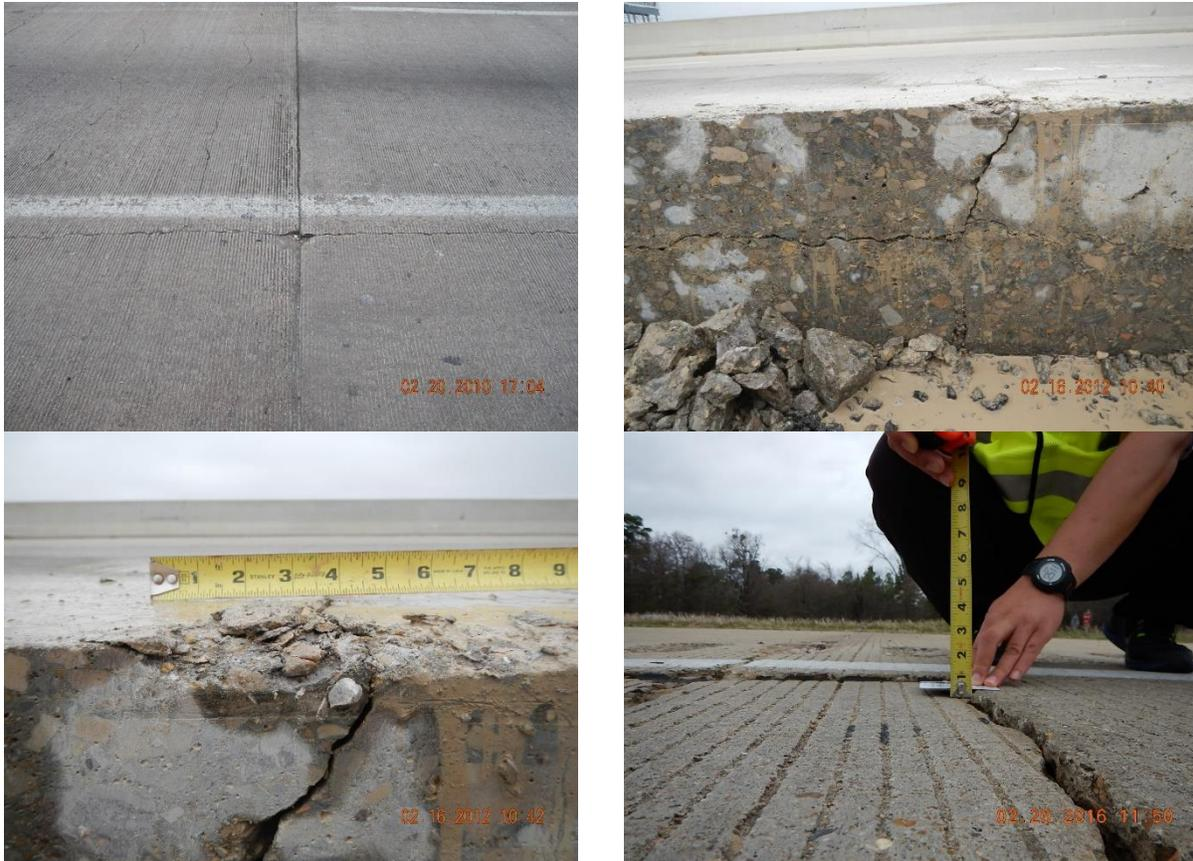
**Figure 5.56** CRCP horizontal cracking observed in IH45 Dallas
