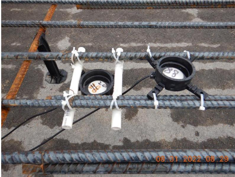
**Figure 5.6** REBEL Sensor and its typical installation
