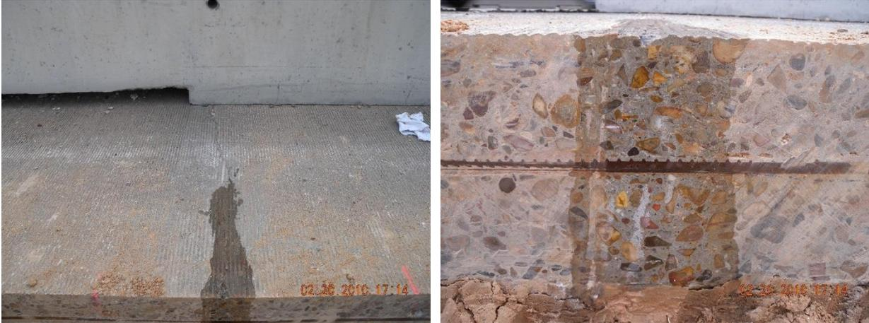
**Figure 2.14-**(a) Wide crack width on the slab surface (left); (b) Transverse crack profile through slab depth (right)
