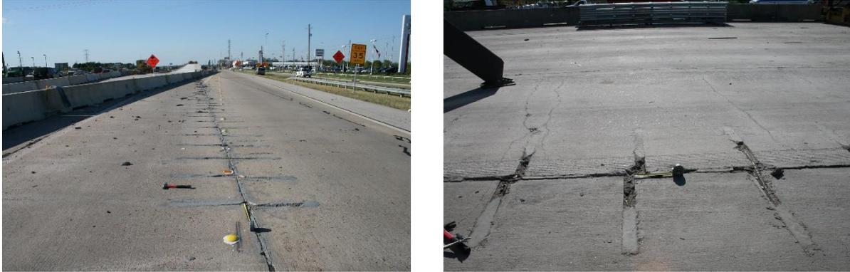
**Figure 5.51** CRCP expansion and resulting stapling failure
