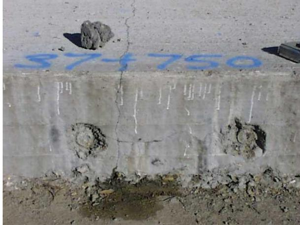
**Figure 3.1** Horizontal cracking in new CRCP
