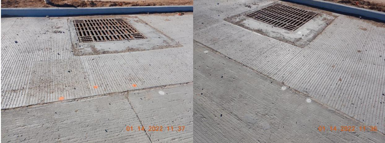
**Figure 5.91** Development of reflection cracking at SC #1 from the drainage manhole
