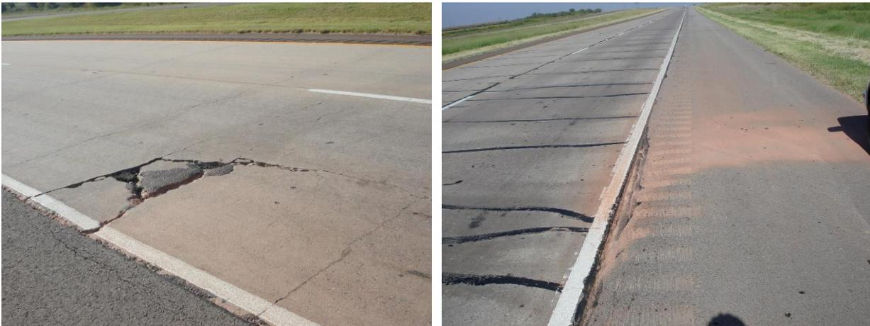
**Figure 2.7-(a)** Punchout distress on US 287 in Harrold (left); (b) Severe pumping on US 287 in Harrold (right)
