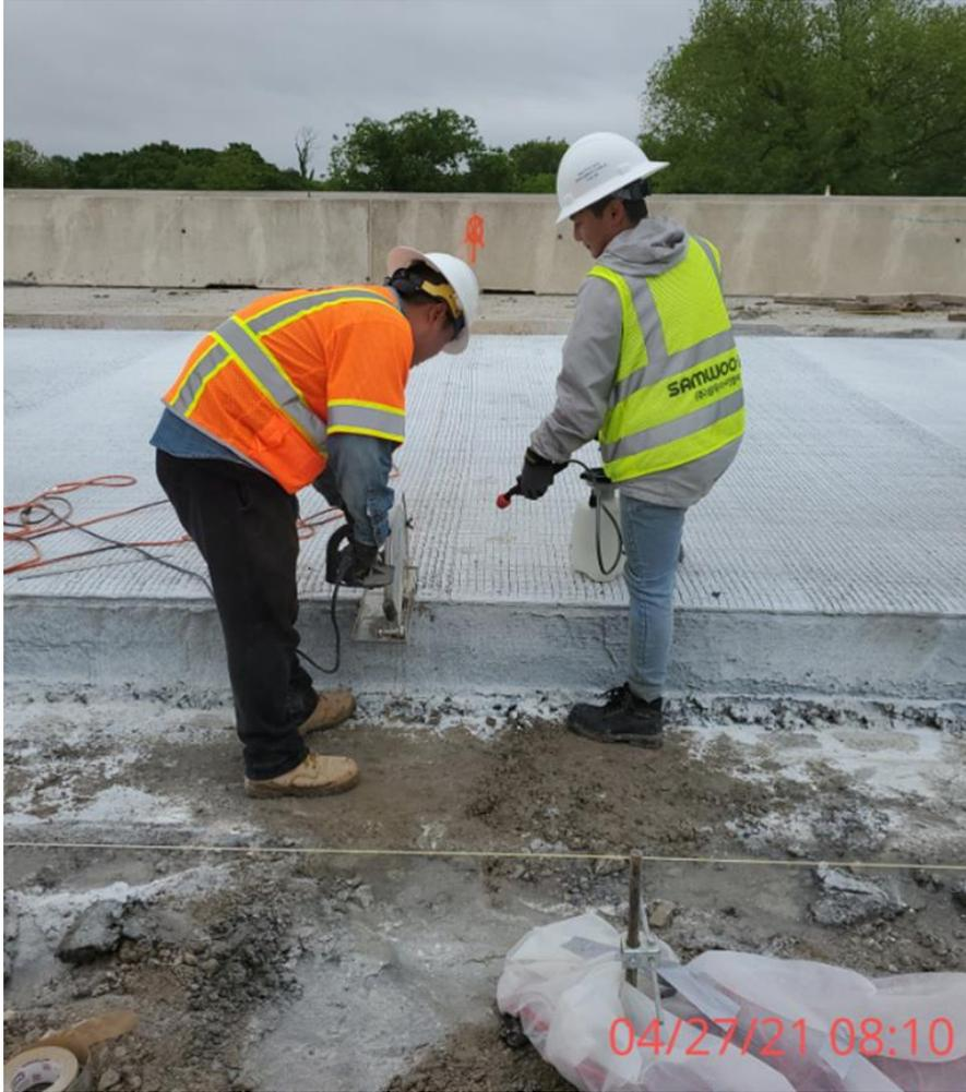
**Figure 5.19** Sawcut operation
