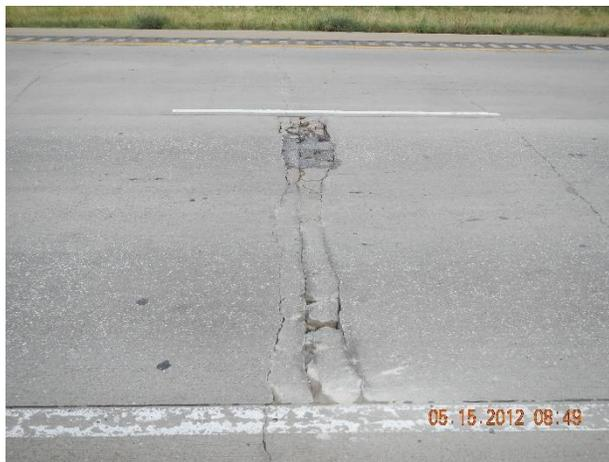
**Figure 3.4** Distress caused by horizontal cracking on IH 35
