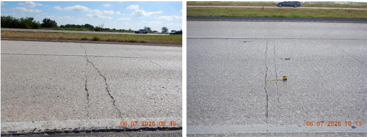
**Figure 2.4-**(a) Y-crack with no distress (left); (b) Short crack spacing (right)
