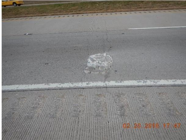
**Figure 3.3** Distress caused by horizontal cracking on IH 20
