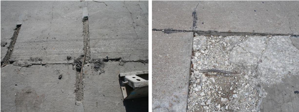
**Figure 2.11-**(a) Stapling failure due to slab expansion (left); (b) Failure of full-depth repair due to slab expansion (right)
