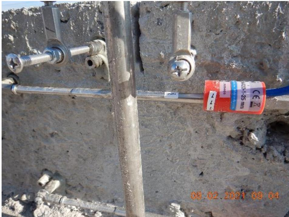
**Figure 5.25** Crack propagation at the upper-depth section (2-2) in US62/180 El Paso
