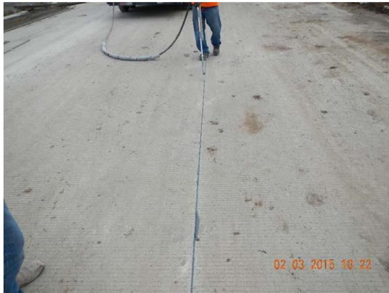
**Figure 2.9 Sealant installation**
