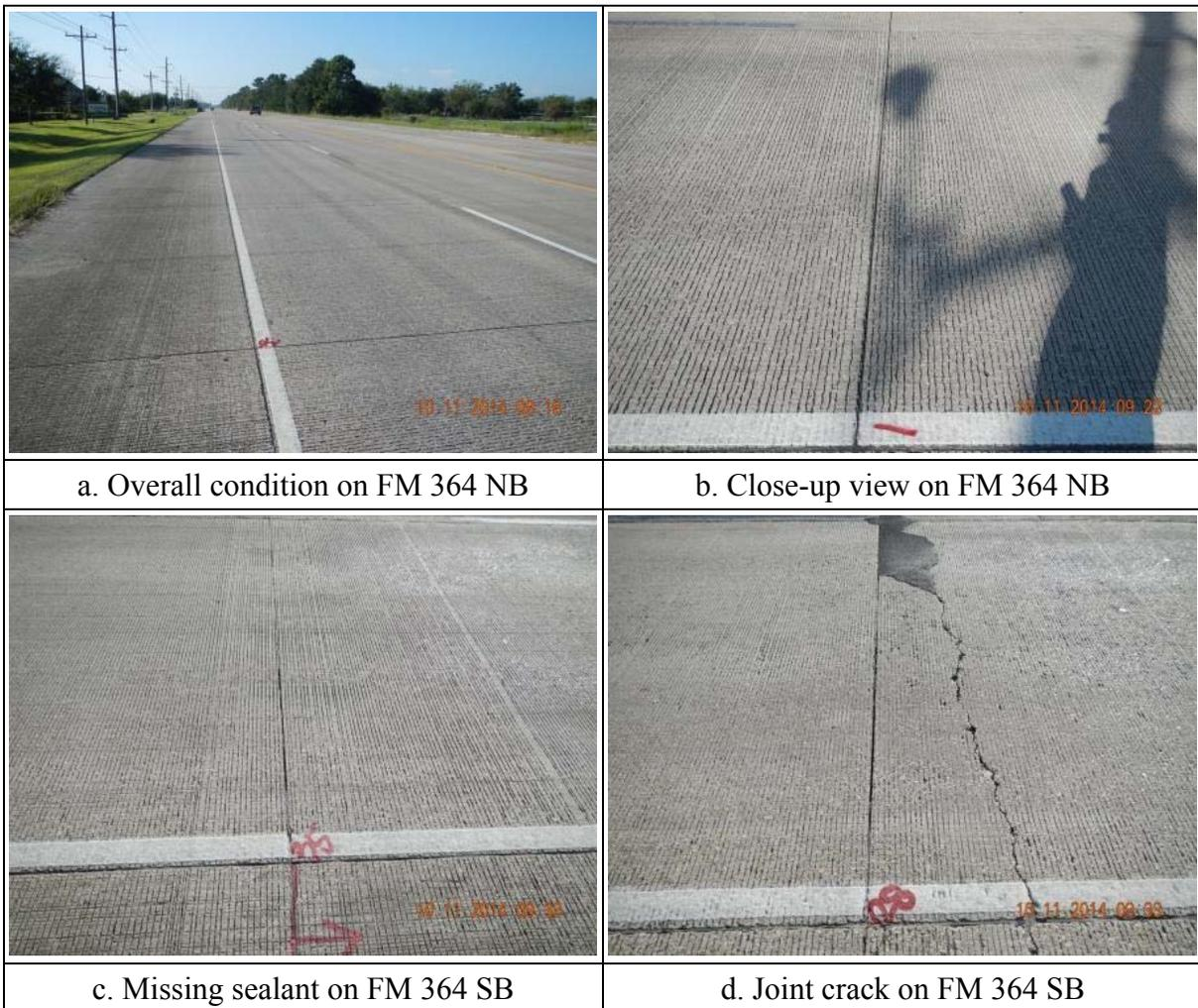
Figure 3.10 Sealant condition on FM 364-BMT [NO. 38]
