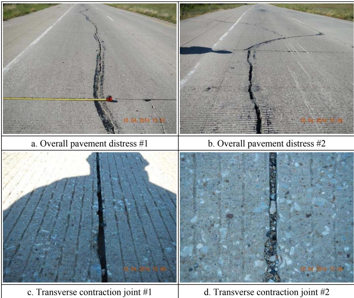
**Figure 3.8 Sealant condition on SL 288-DAL [NO. 47]**
