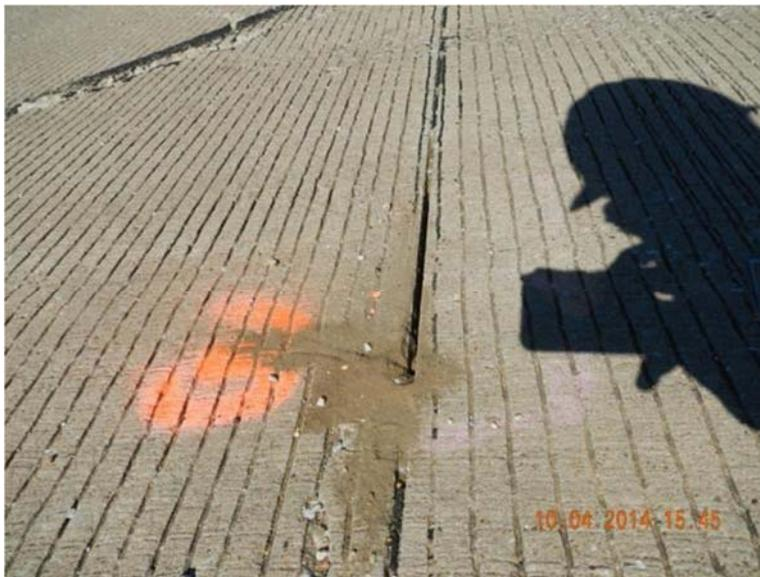
**Figure 2.5 High level of stone intrusion**
