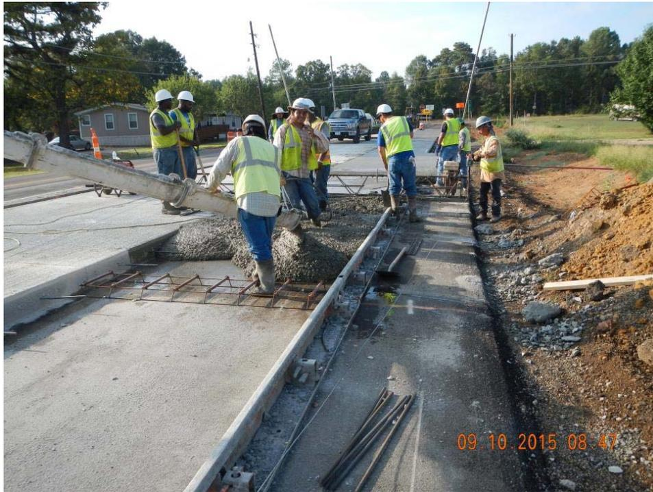
**Figure 4.15 Concrete placement on FM 2253**
