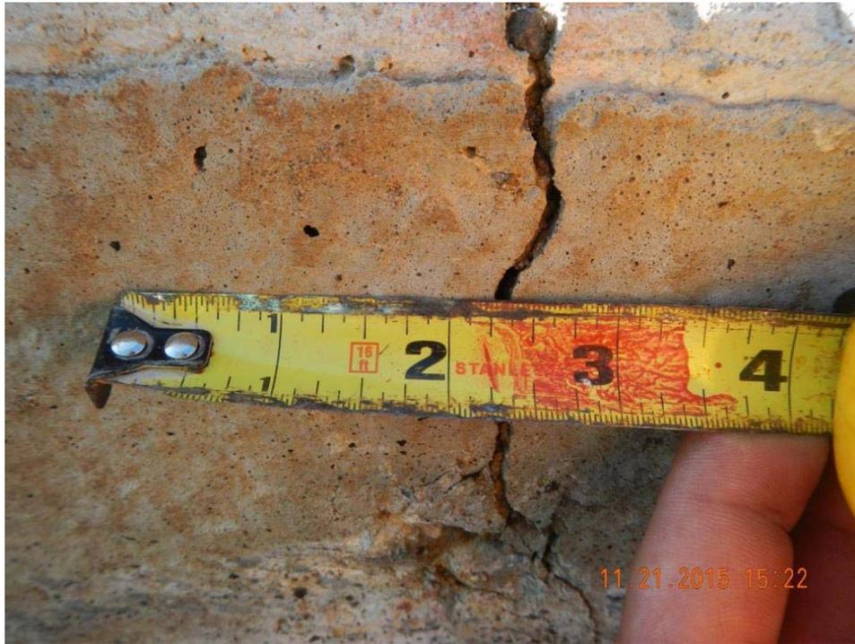
**Figure 4.24 Crack width at Joint on FM 2253**
