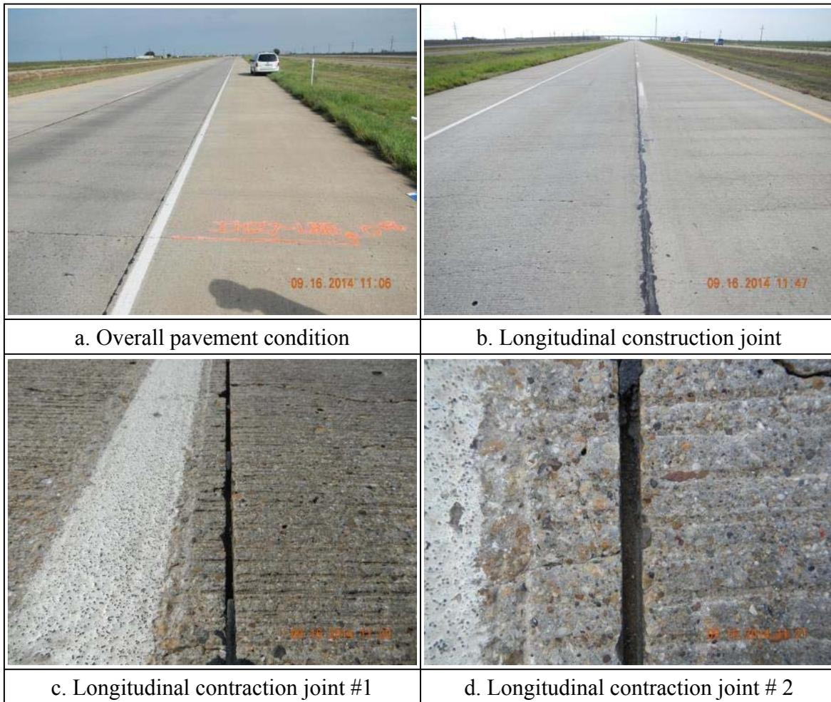
**Figure 3.14 Sealant condition on IH 27-LBB [NO. 46]**
