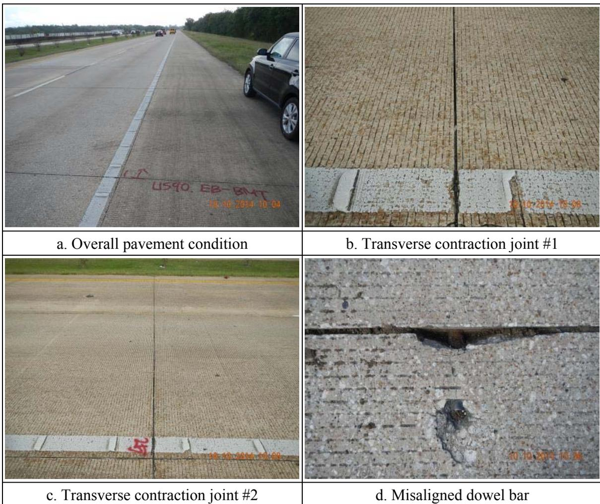
**Figure 3.12 Sealant condition on US 90 EB-BMT [NO. 32]**
