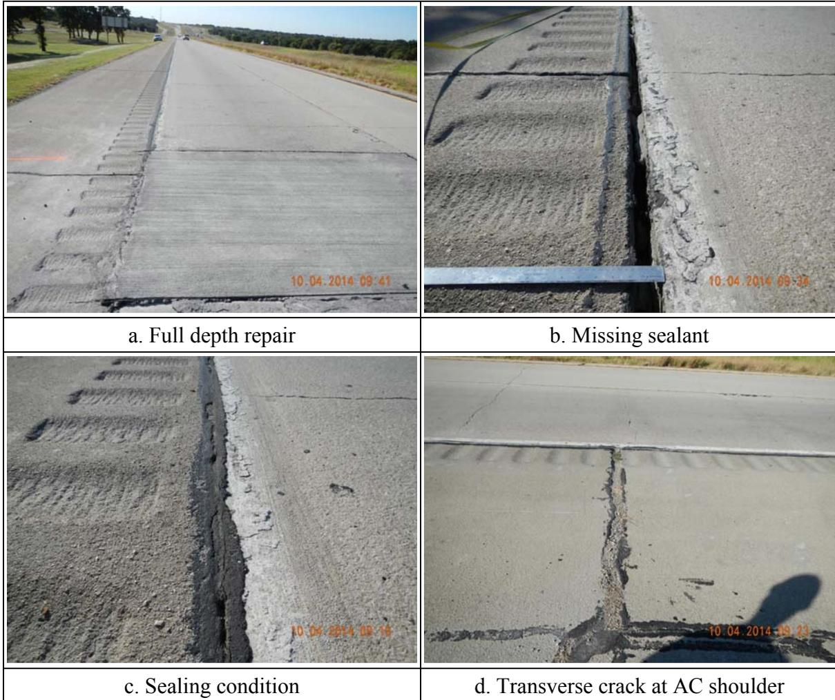
**Figure 3.21 Sealant condition on US 287-WFS [NO. 51]**
