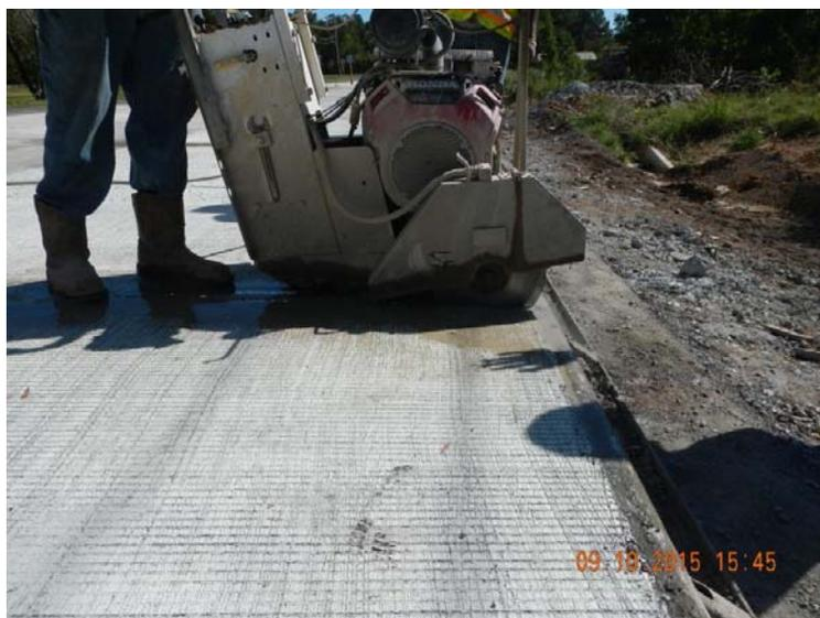
**Figure 4.20 Sawcut at pavement edge**
