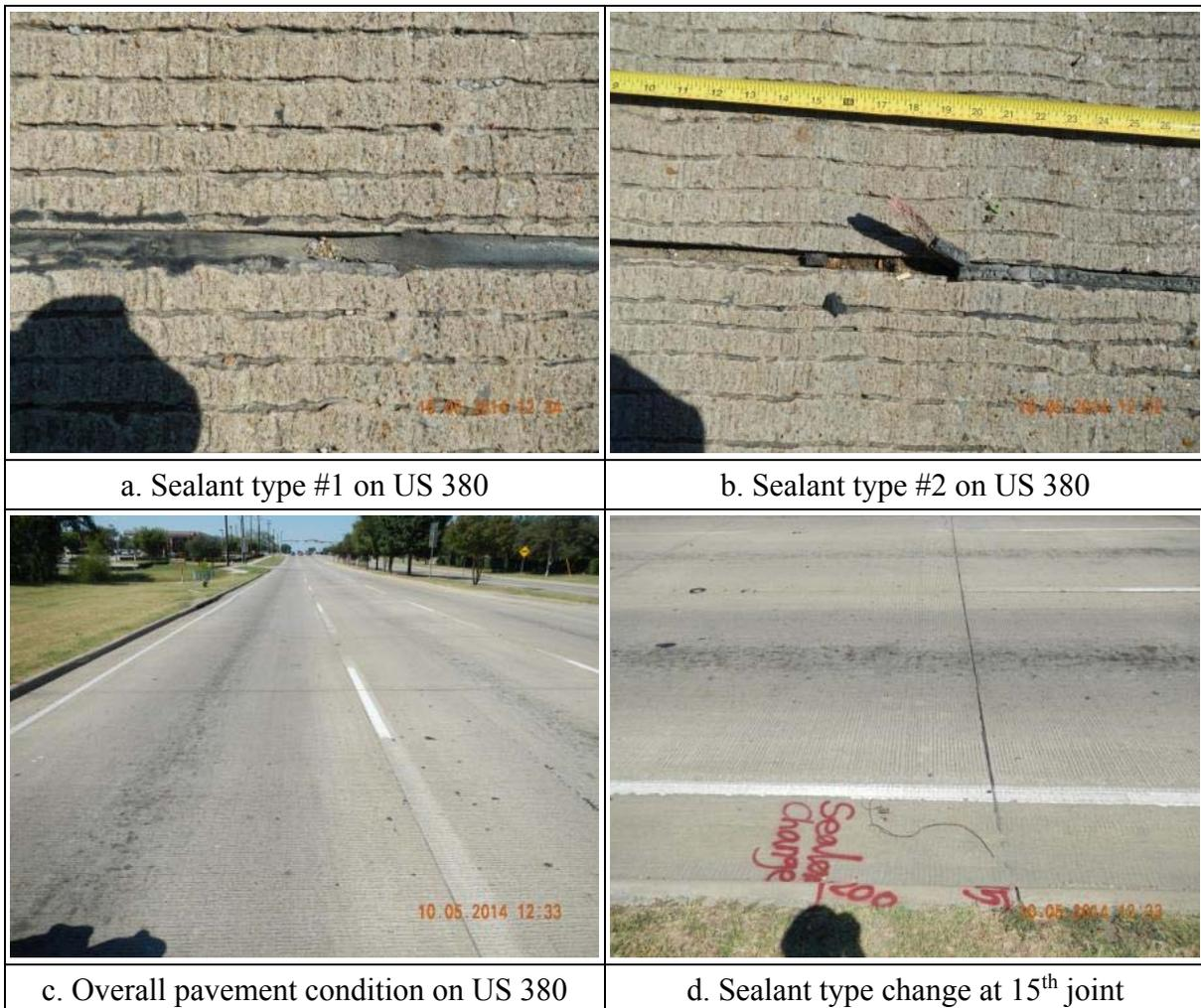
**Figure 3.11 Sealant condition on US 380-DAL [NO. 39]**
