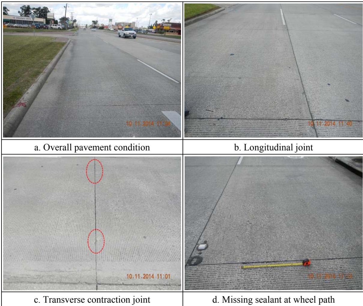
**Figure 3.5 Sealant condition on US 90 BR-BMT [NO. 27]**
