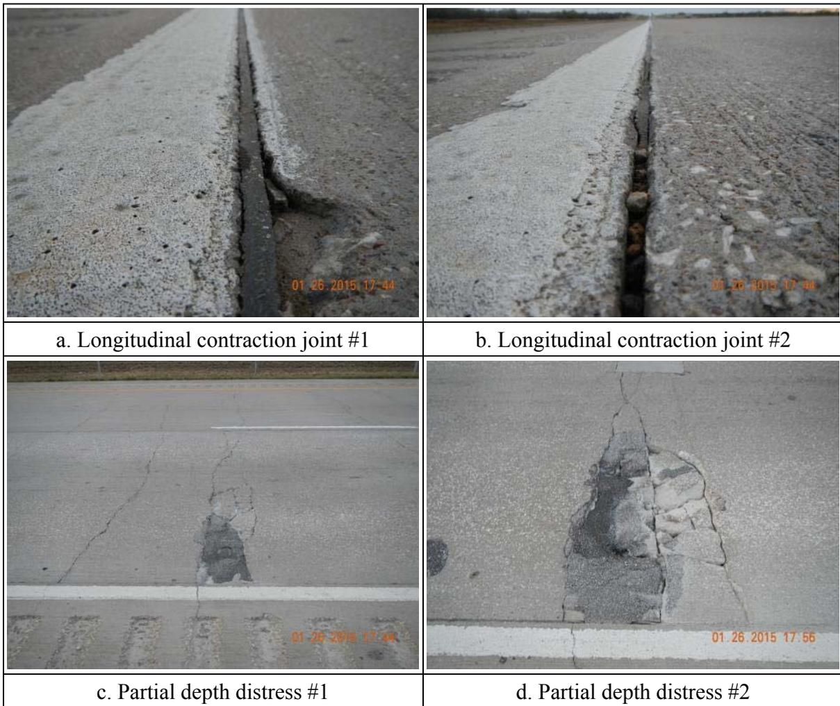
**Figure 3.6 Sealant condition on IH 35-LRD [NO. 42]**
