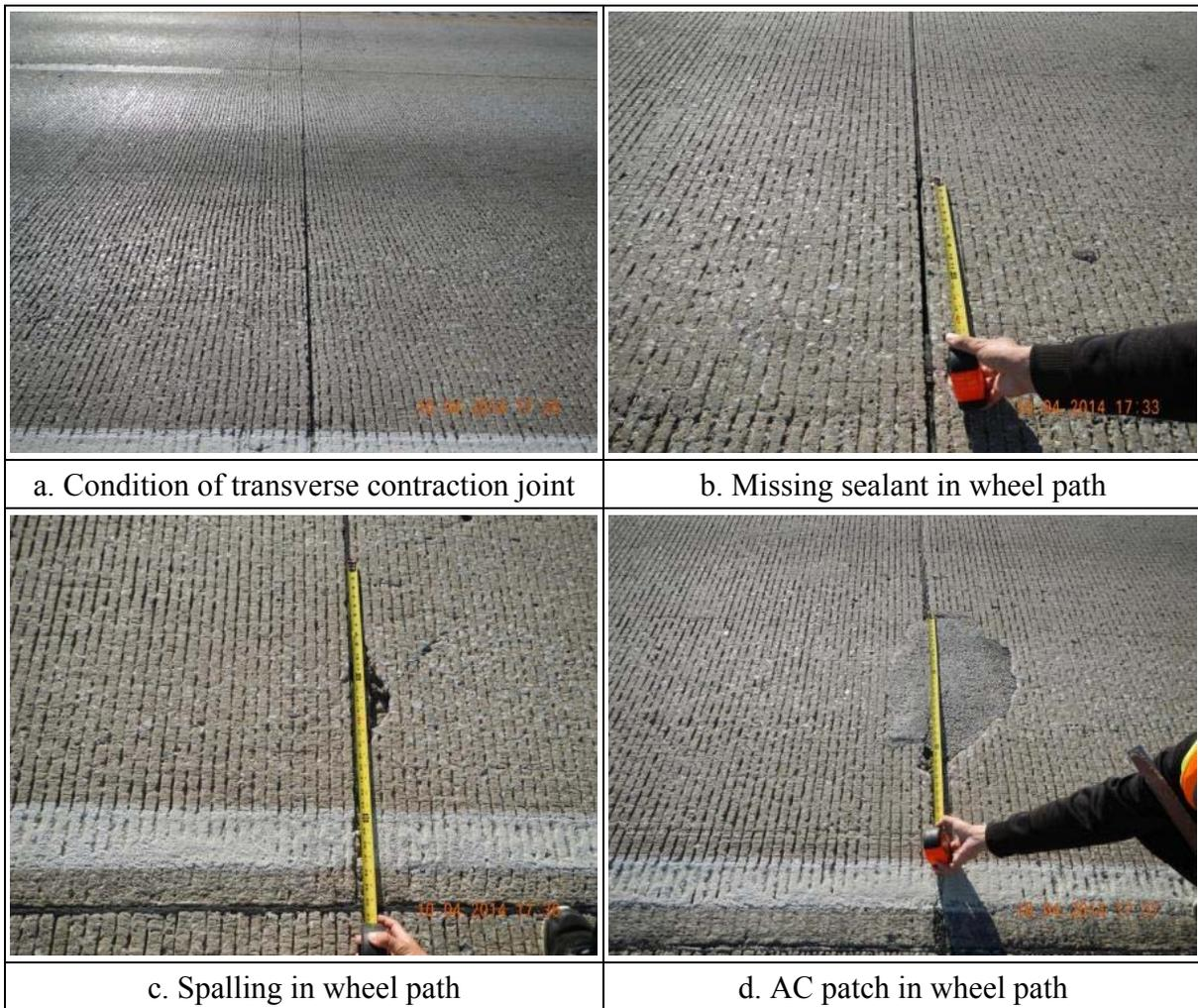
**Figure 3.15 Sealant condition on IH 35-DAL [NO. 45]**
