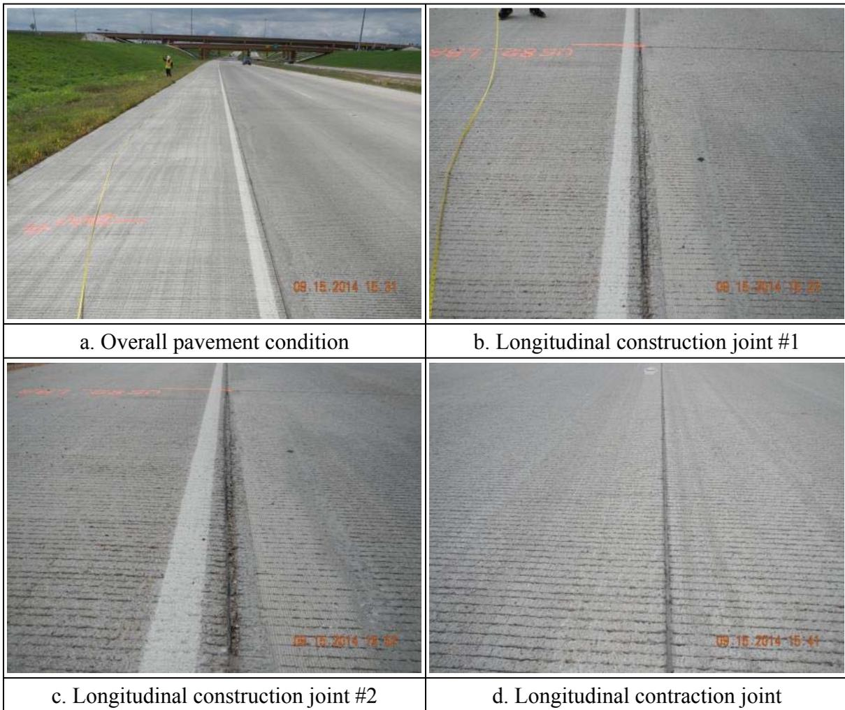
**Figure 3.3 Sealant condition on US 82-LBB [NO. 29]**
