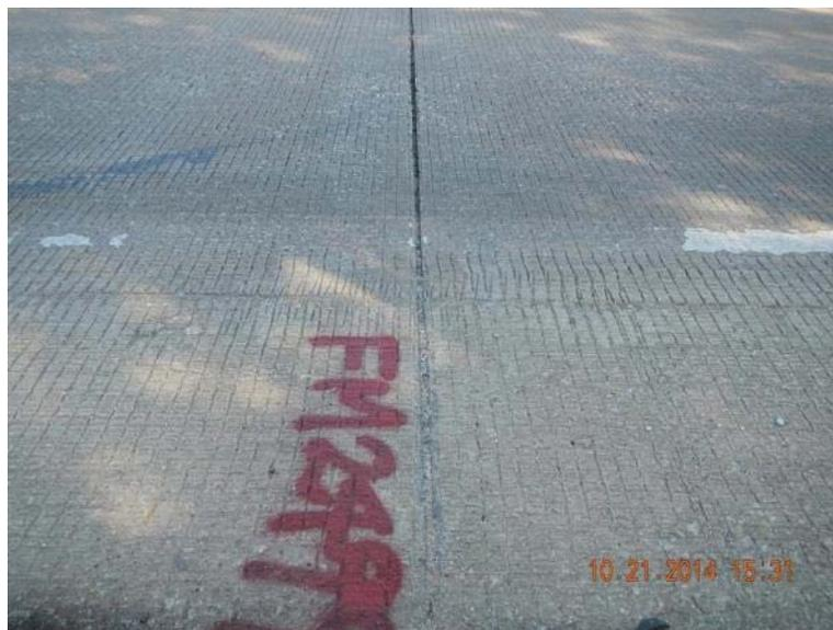
**Figure 2.3 Low level of stone intrusion**
