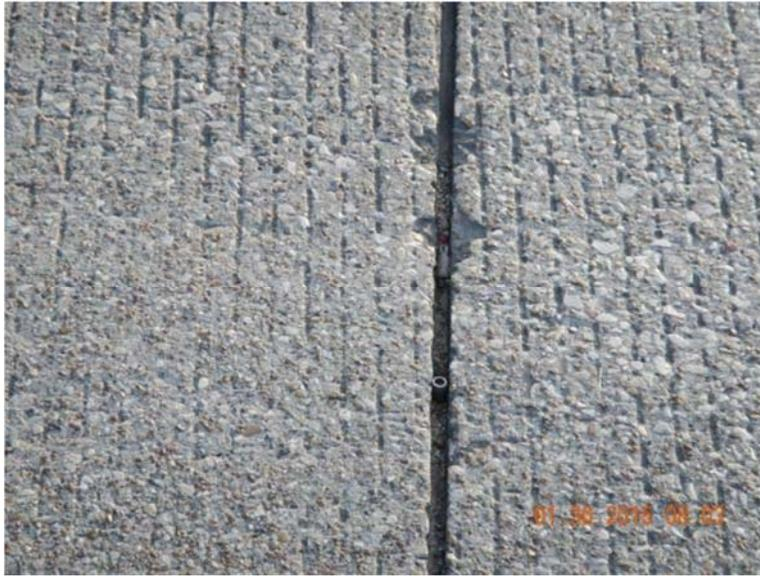
**Figure 2.4 Medium level of stone intrusion**
