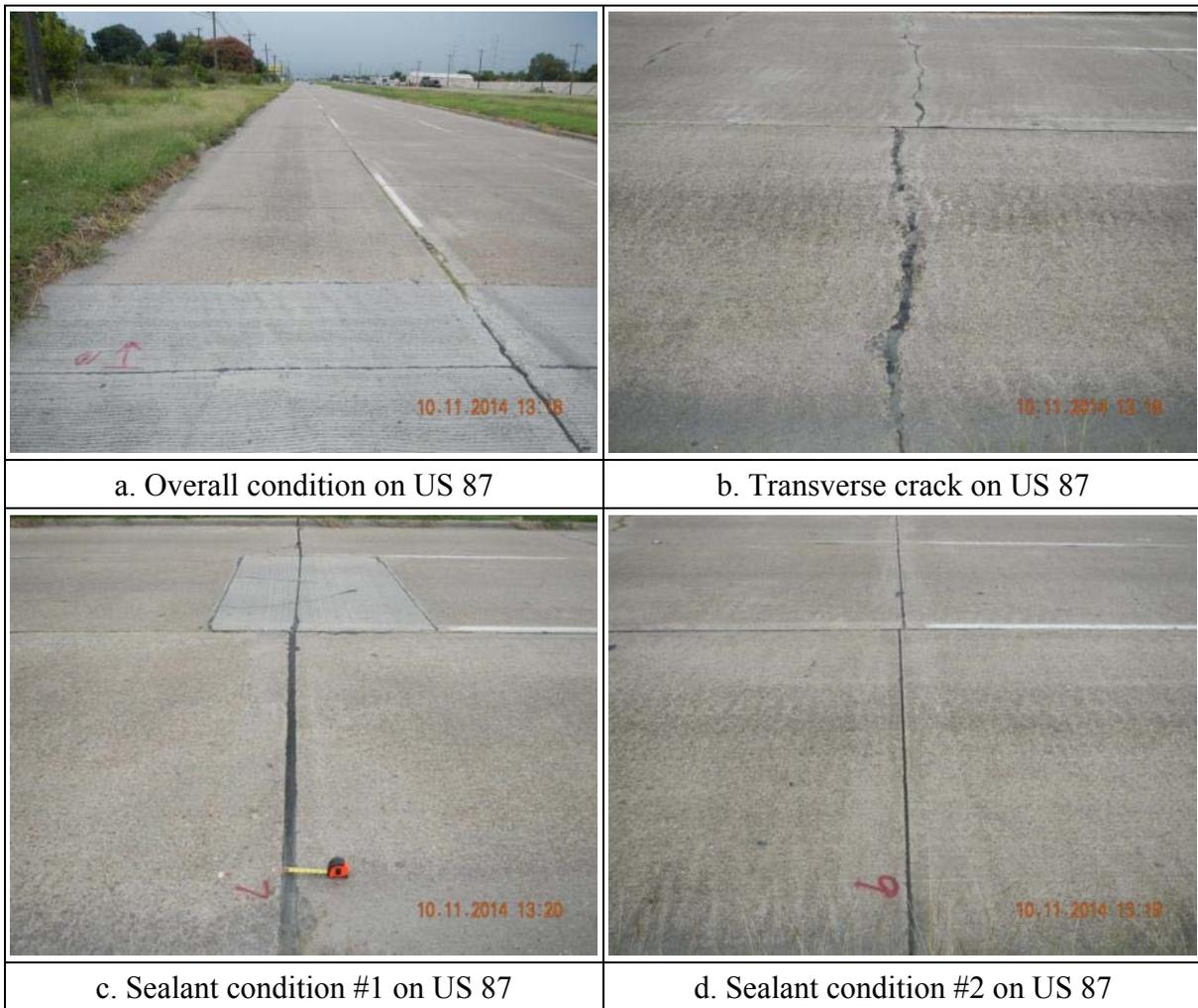
**Figure 3.17 Sealant condition on US 87-BMT [NO. 61]**
