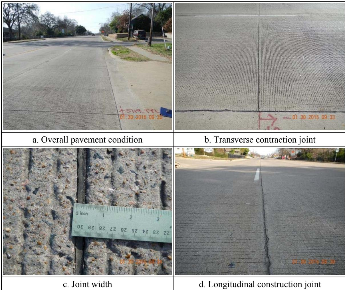
**Figure 3.7 Sealant condition on SH 9-TYL [NO. 40]**
