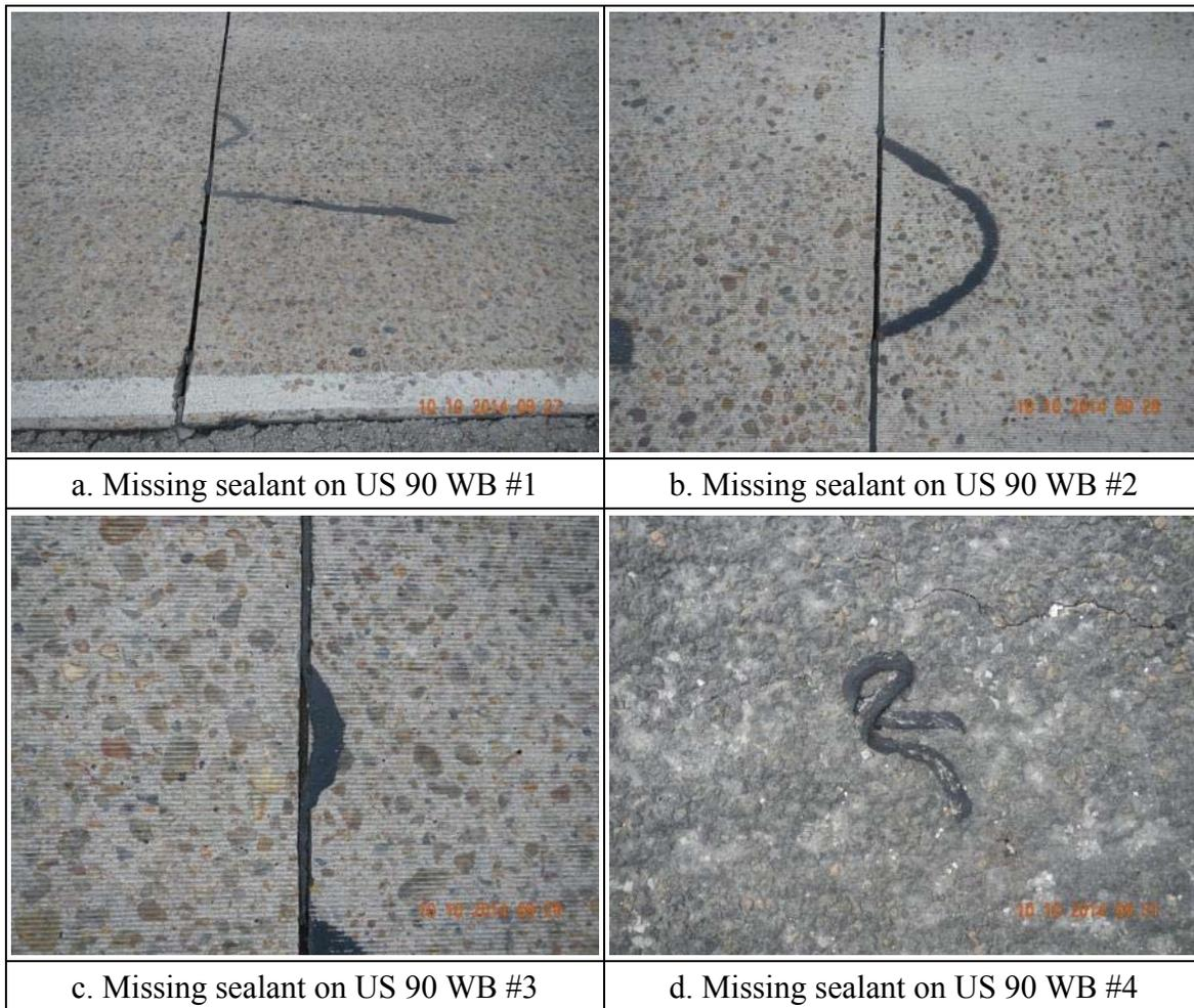
**Figure 3.13 Sealant condition on US 90 WB-BMT [NO. 32]**
