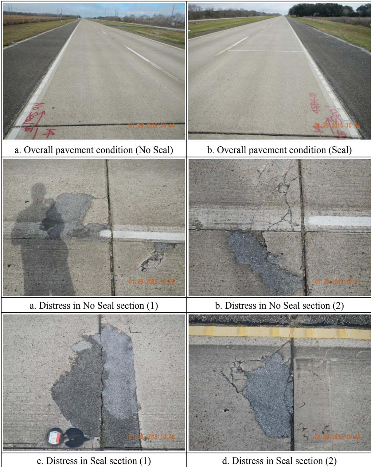
**Figure 5.5 Distresses at Sealed and No Sealed sections**
