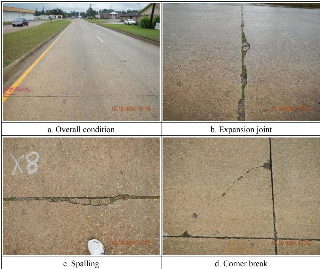
**Figure 3.18 Sealant condition on SH 326-BMT [NO. 55]**
