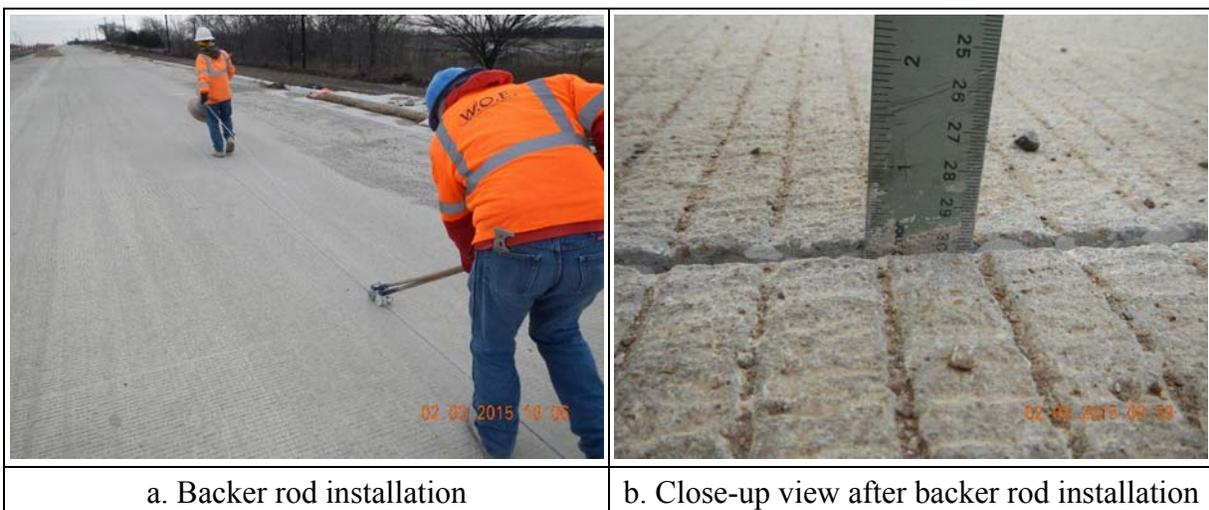
**Figure 2.8 Backer rod installation**
