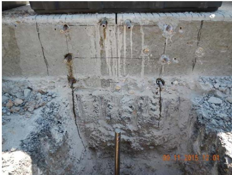
**Figure 4.19 Joint condition before gage installation**
