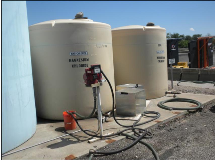
**FIG 4.** MeltDown® Apex is a magnesium chloride brine solution obtained by solarizing natural salt brine from the Great Salt Lake in Utah
