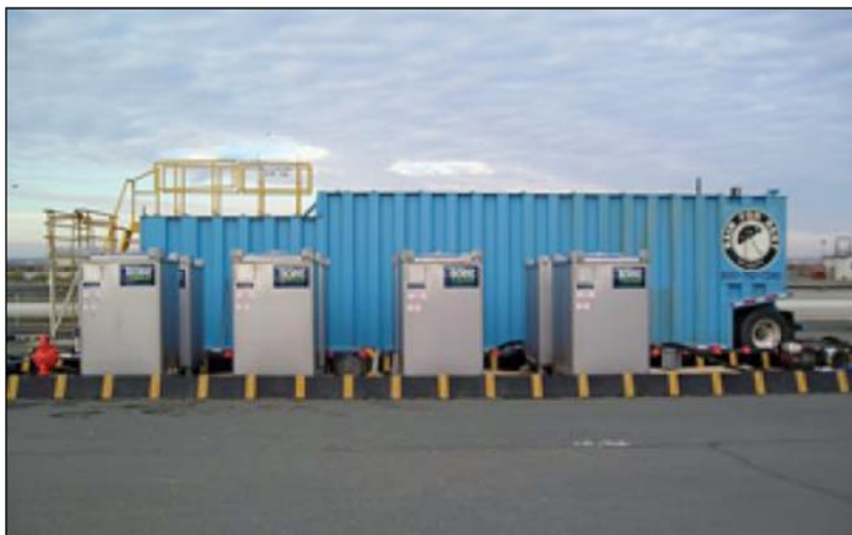
FIG 35. TxDOT districts south of IH20 should use pre-blended brine with temporary storage in frac tanks
