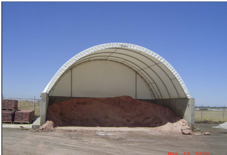
FIG 32. Dedicated salt storage sheds for bulk granular salt are suitable for material storage in Texas' snowy districts
