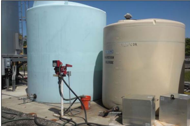
FIG 31. Liquid storage includes adequate tank capacity, proper-sized pumps and hoses for loading and recirculation
