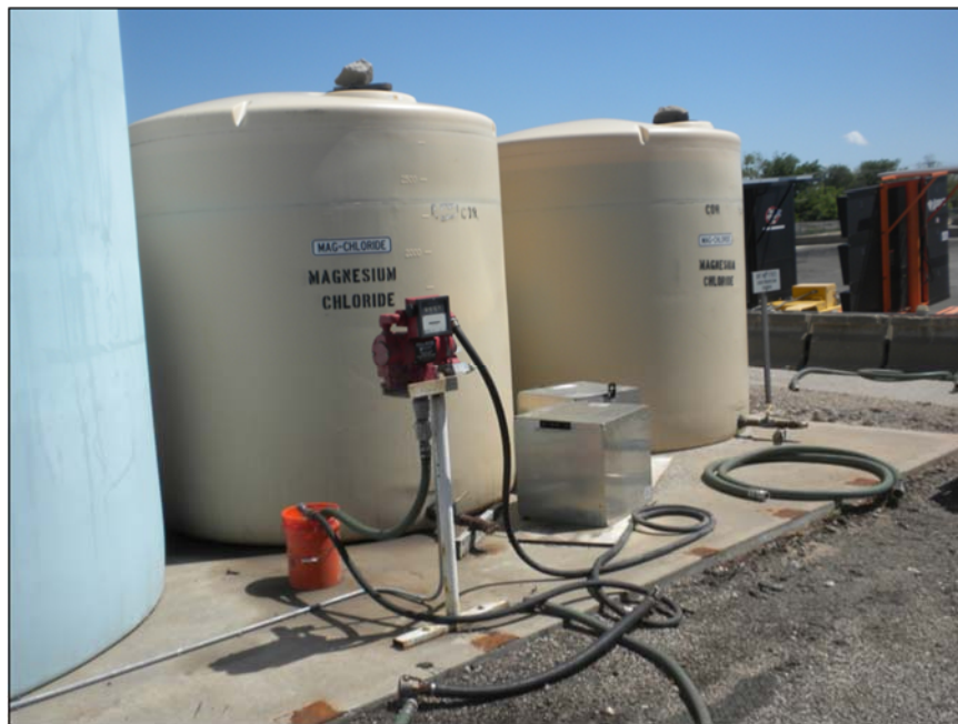
FIG 16. MeltDown® Apex is a magnesium chloride brine solution obtained by solarizing natural salt brine from the Great Salt Lake in Utah
