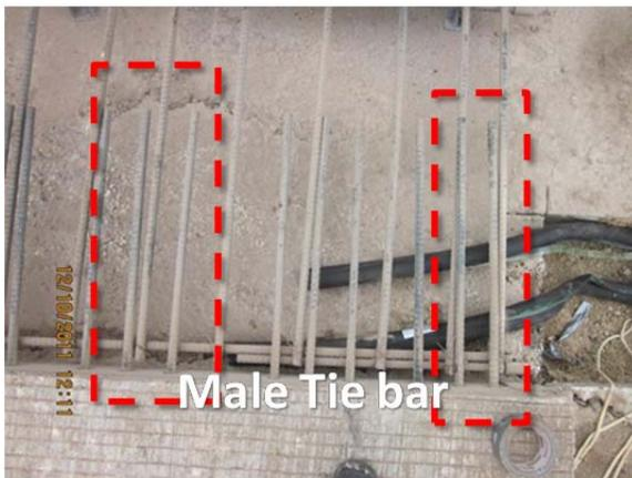
**Figure 3. 6 Male Tie-Bars Inserted After Removing the Headers at Morning construction side at LBB-I**
