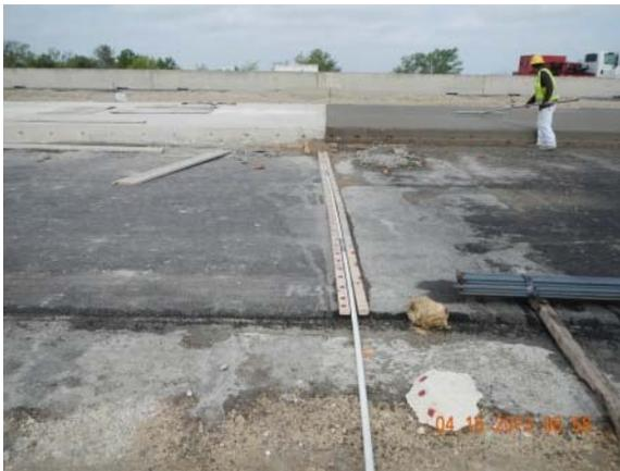
**Figure 3.68 Steel Strain Gage Lead Wire Protected by PVC Pipes and Embedded in the Asphalt Base**
