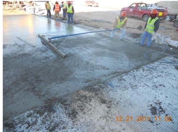
**Figure 3.16 Concrete Finishing at LBB-II Morning Test Section**
