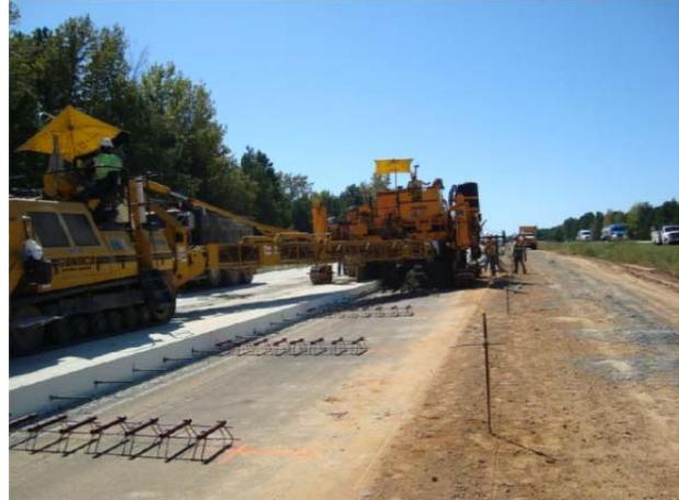
**Figure 2. 42 Construction of CRCP Tied to CRCP on US 59 in the Atlanta District**
