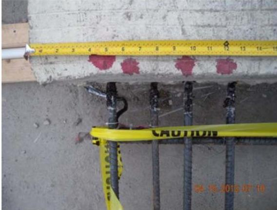
**Figure 3.66 Steel Strain Gage Installation Near Transverse Construction Joint**
