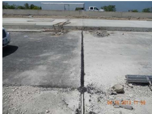
**Figure 3.69 Embedded PVC Pipes Carrying SSG Lead Wires Covered With Cold-Mix Asphalt**
