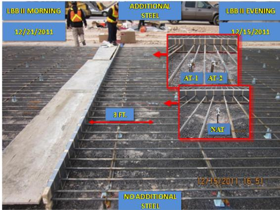
**Figure 3.13 VWSG Installation at LBB-II Evening Test Section**
