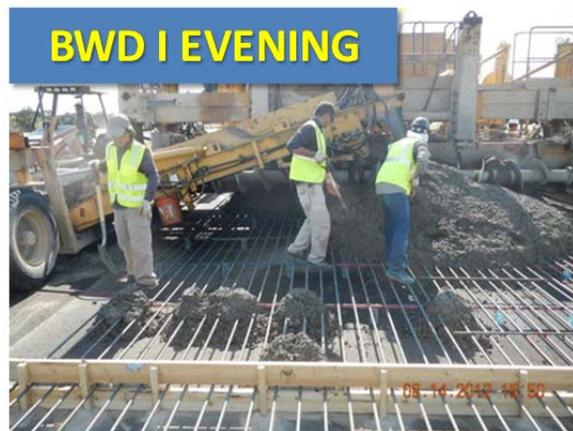
Figure 3.34 Protecting VWSGs at BWD-I Evening Test Section
