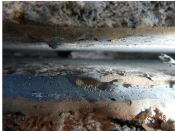
**Figure 2. 31 Debonding Between Steel and Concrete on IH 40 in the Childress District**
