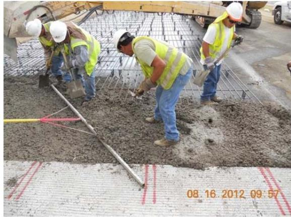
**Figure 4. 31 Manual Placement of Concrete At the Transverse Construction Joint – Morning**
