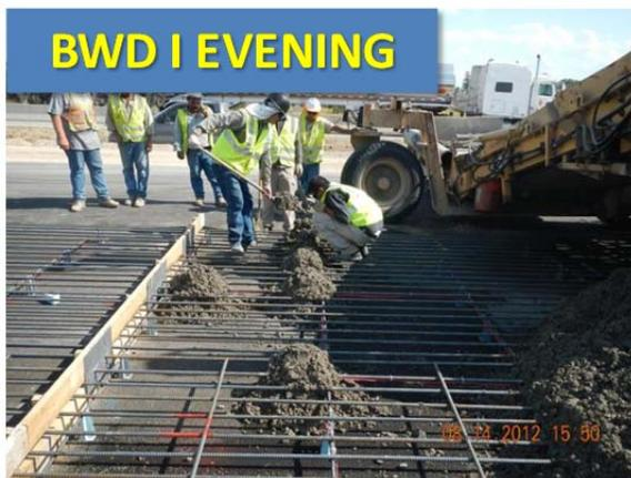
Figure 3.33 Concrete Placement at BWD-I Evening Test Section
