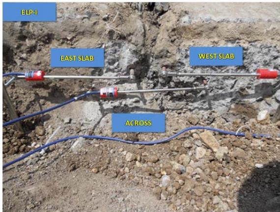
**Figure 4. 7 Crackmeter Installation Across Transverse Construction Joint at ELP-I Test Section**
