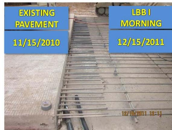
**Figure 3. 7 Steel Placement at LBB-I Test Section**
