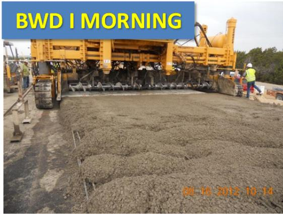
**Figure 3.35 Concrete Placement at BWD-I Morning Test Section**
