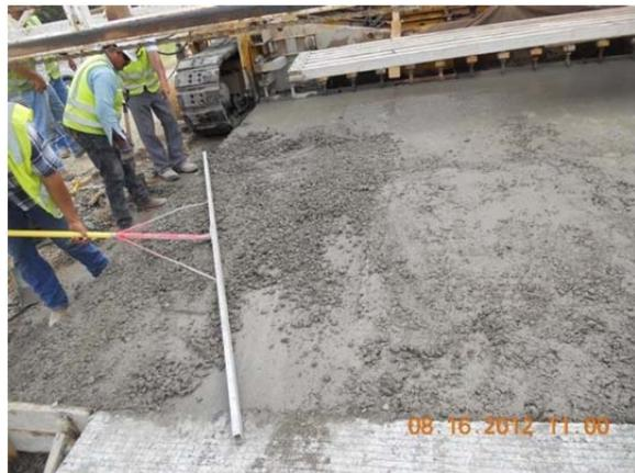
**Figure 4. 33 Manual Finishing of Concrete at BWD-I Test Section**
