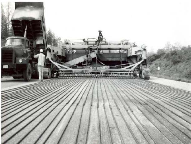
**Figure 2. 45 CRCP Const. With Mechanical Steel Placement**
