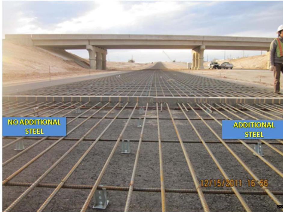
**Figure 3. 11 Steel Placement at LBB-II Test Section**
