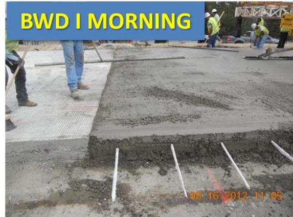
**Figure 3.36 Concrete Finishing at BWD-I Morning Test Section**
