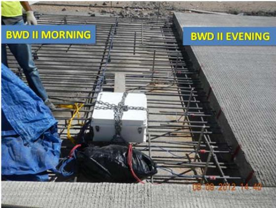
**Figure 3. 48 Crackmeters Installed to Measure Longitudinal Slab Movement at BWD-II Test Section**
