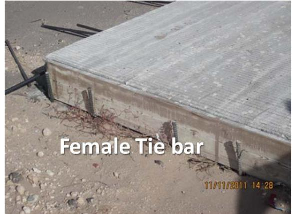
**Figure 3. 5 Header Installed After Placing Female Tie-bars at Existing Slab at LBB-I Test Section**
