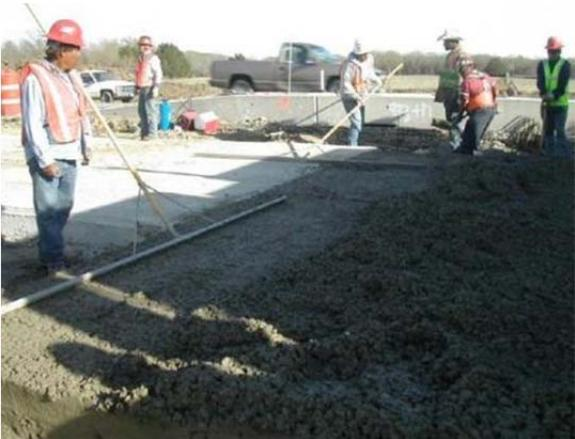
**Figure 2. 15 Concrete Consolidation at TCJ**
