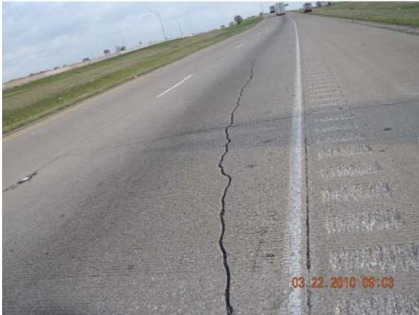
**Figure 5.3 Longitudinal Cracking in CPCD**
