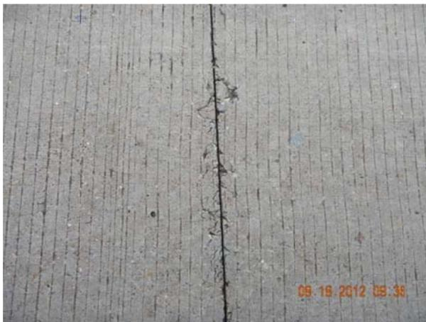
**Figure 5.7 Micro-Damage Due to Early Entry Saw Cut**
