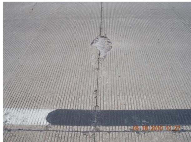
**Figure 5.8 Spalling at Saw Cut Joint Due to Micro-Damage in Concrete**
