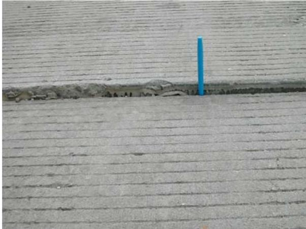
**Figure 5.1 Faulting in Transverse Joint**
