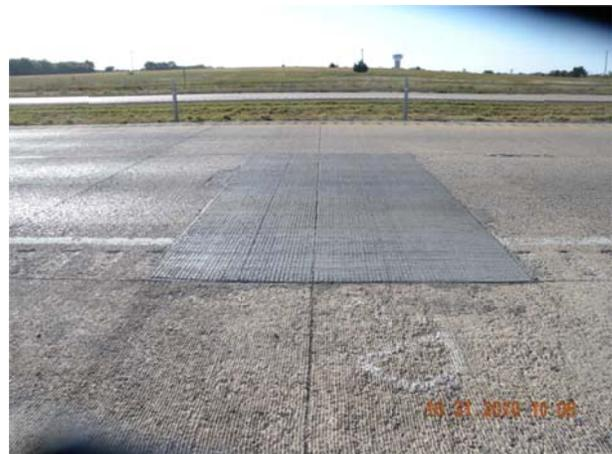
**Figure 5.6 Repair of Distress at TCJ**
