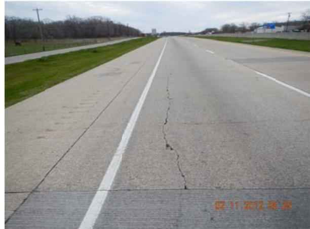
**Figure 5.4 Longitudinal Cracking in CRCP**
