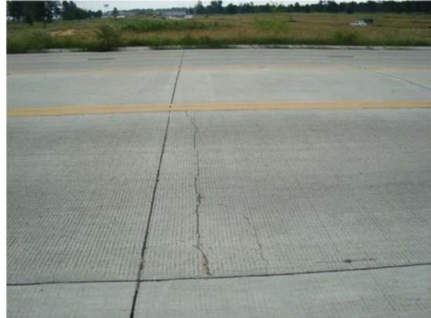
**Figure 5.2 Transverse Cracks Near Joint**
