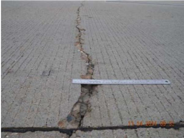
**(a) Typical spalling on SL 151**
