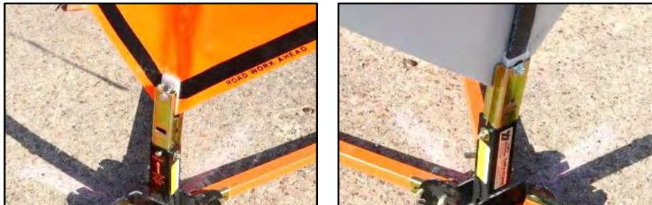
**Figure 5.15. Bolt Added Through Stand Bracket and Vertical Stay.**
