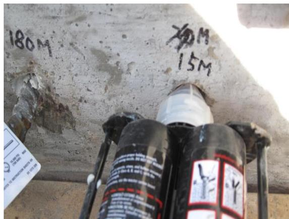
Figure 3.3- (a) Inject epoxy with handgun – Compliance
