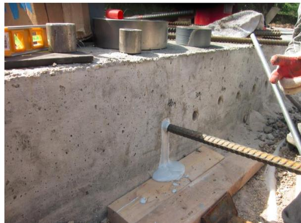
Figure 3.2- (f) Insert a rebar in the hole
