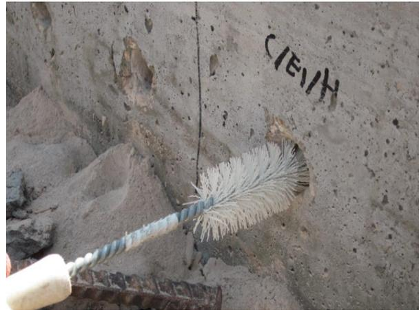
Figure 3.2- (b) Clean hole with brush
