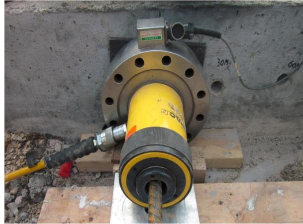
Figure 3.2- (j) Install hydraulic jack
