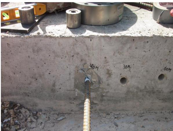
Figure 3.2- (g) Prevent the epoxy leak
