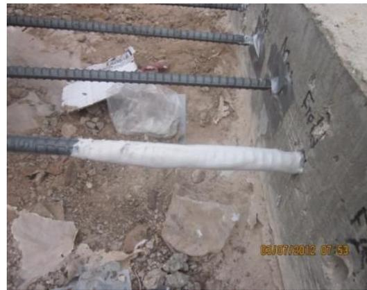
Figure 3.3- (e) Insert the rebar into a hole
