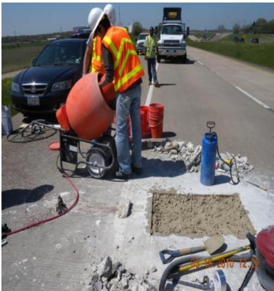
Figure 11 – Mixing of prepared repair materials at the job site
