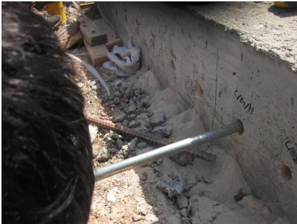
Figure 3.2- (c) Clean hole with air tube
