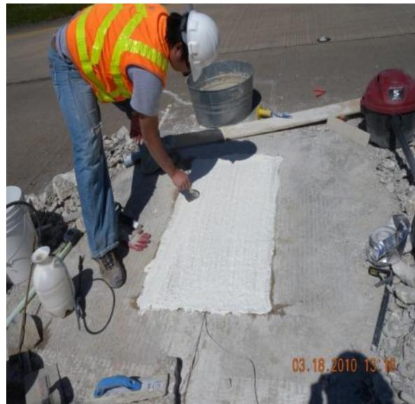
Figure 12 – Application of sufficient curing compound
