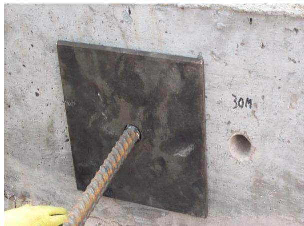
Figure 3.2- (h) Place a steel plate
