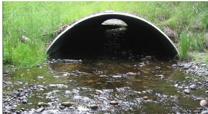
Figure 12: Example of a buried-invert culvert [from Crookston (2008)].
