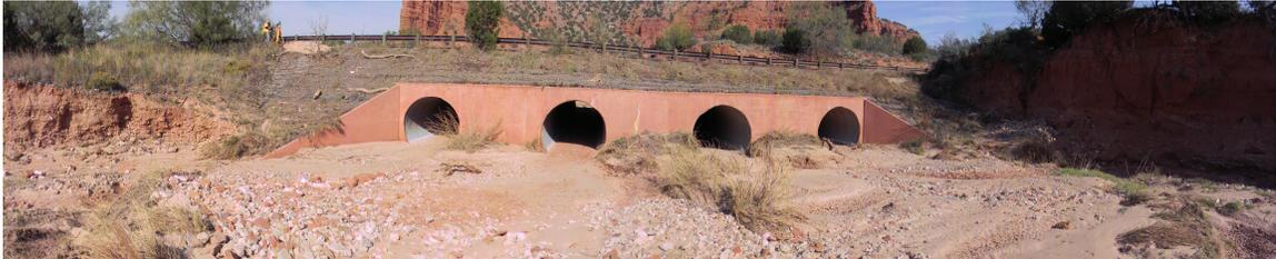
Figure 1: 4-Barrel Culvert System at Caprock Canyons State Park (G.R. Herrmann)
