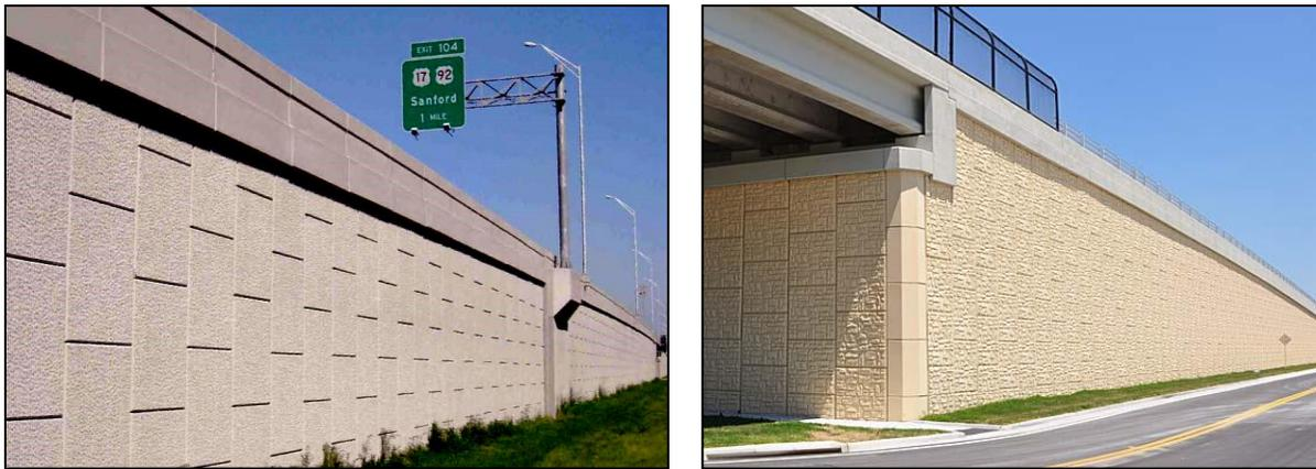
**Figure 1.2** MSE Retaining Walls Used in Transportation Applications
