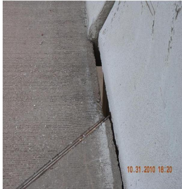
Figure 2.14 Misalignment of traffic rail (2)
