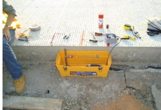
Figure 4.25 Installation of the crackmeter with protection box
