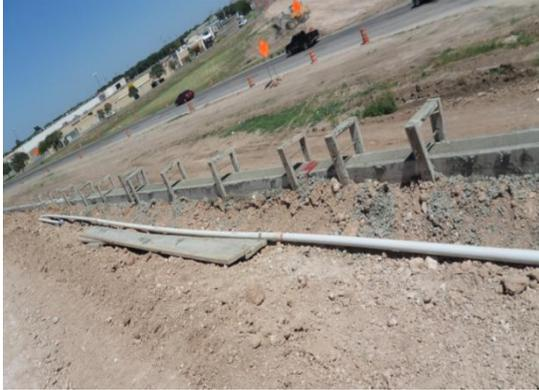
Figure 4.44 Pipes to protect gage cables
