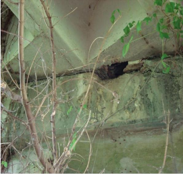
Figure 2.11 Damage in bent cap
