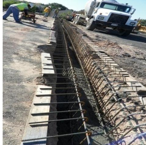
Figure 4.51 Concrete pouring in the lugs cell
