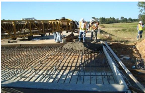
Figure 4.22 Pouring of concrete at the section
