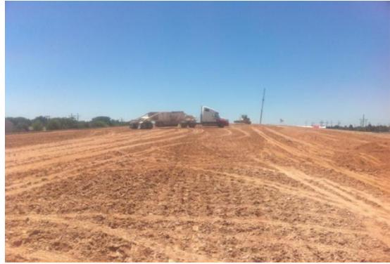
Figure 4.41 Subbase type 6 inches CSB
