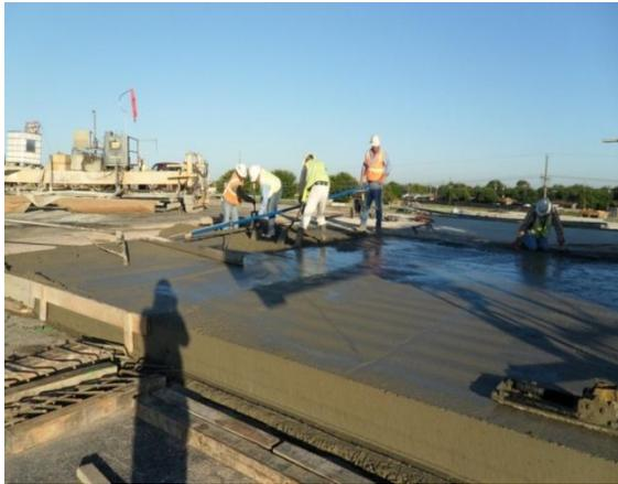
Figure 4.53 Concrete placement on the AL
