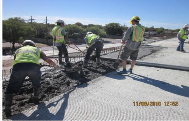
Figure 4.55 Concrete placement in the shoulder area
