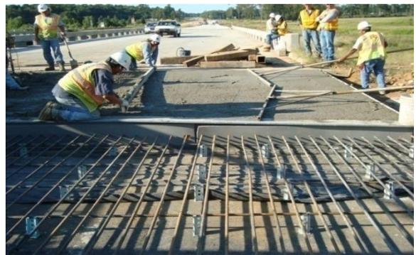
Figure 4.23 Finishing of the concrete
