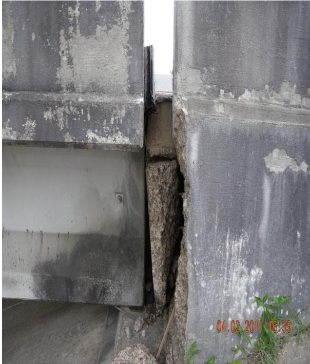
Figure 2.1 Damage in the abutment
