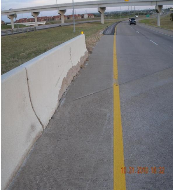
Figure 2.15 Damage in traffic rail
