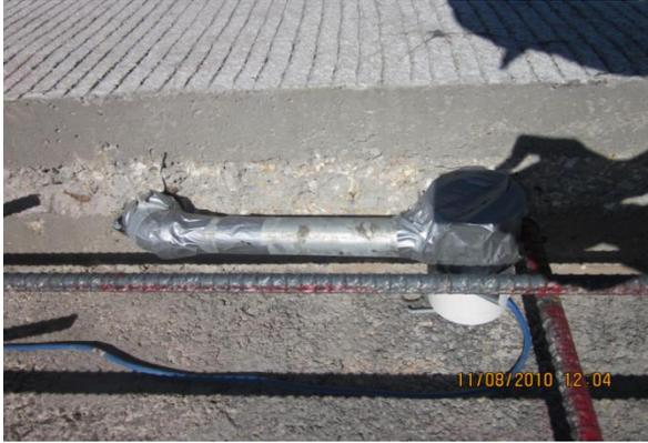
Figure 4.54 Crackmeter installation with protection
