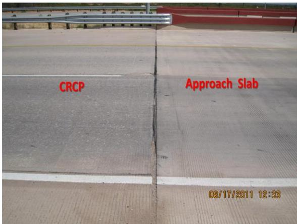
Figure 5.8 Expansion joint at the east end of the CRCP
