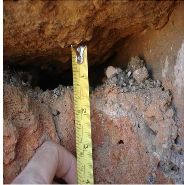
Figure 2.20 Void under bridge approach slab
