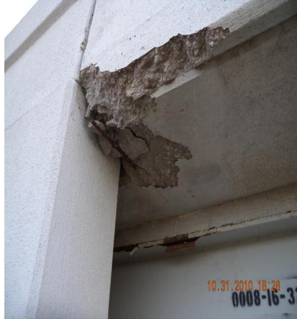
Figure 2.16 Damage in the bridge superstructure
