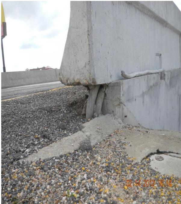
Figure 2.7 Subsidence of embankment material (2)
