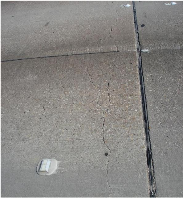
Figure 2.22 Transverse cracks due to voids
