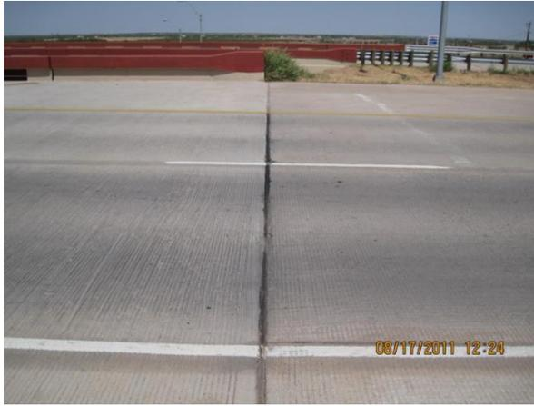
Figure 5.6 Expansion joint at the west end of the CRCP
