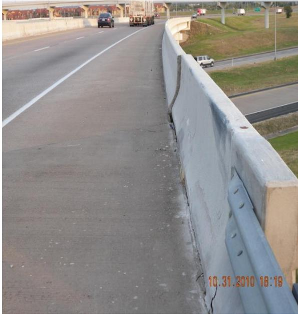
Figure 2.13 Misalignment of traffic rail (1)
