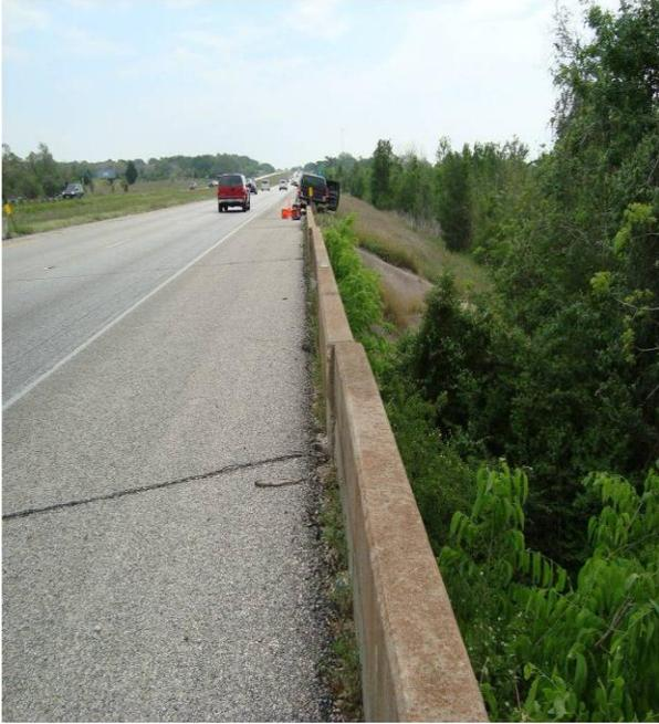
Figure 2.9 Misalignment of the traffic rails
