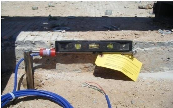
Figure 4.14 Installation of the crackmeter
