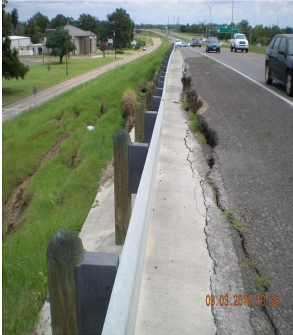
Figure 2.3 Slope failure in the embankment area
