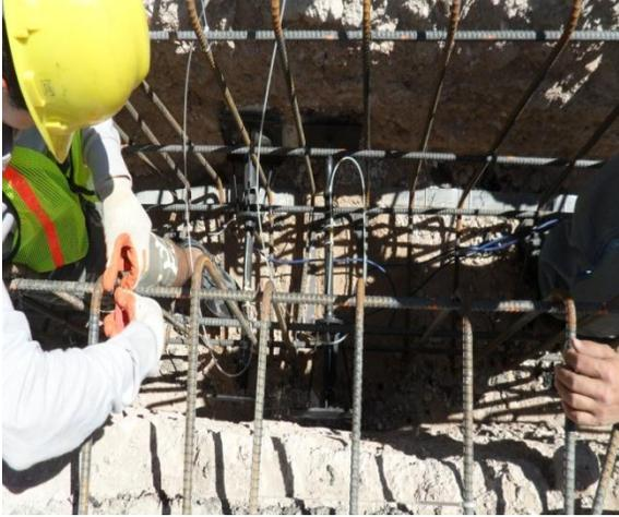
Figure 4.50 Installation of jackout pressure cells
