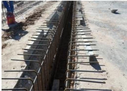
Figure 4.46 Cage tied and placed in the excavated area
