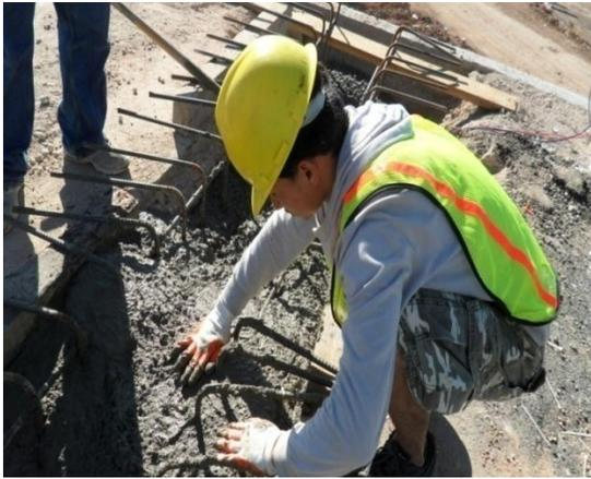
Figure 4.52 Covering the gages with concrete
