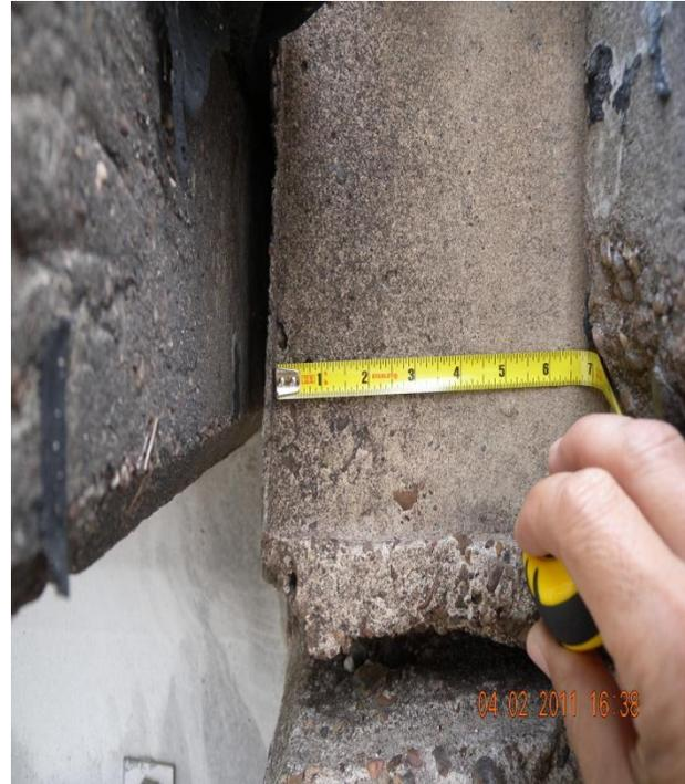
Figure 2.2 Approach slab pushing bridge seven inches
