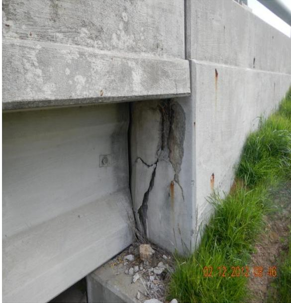
Figure 2.17 Damages in abutment
