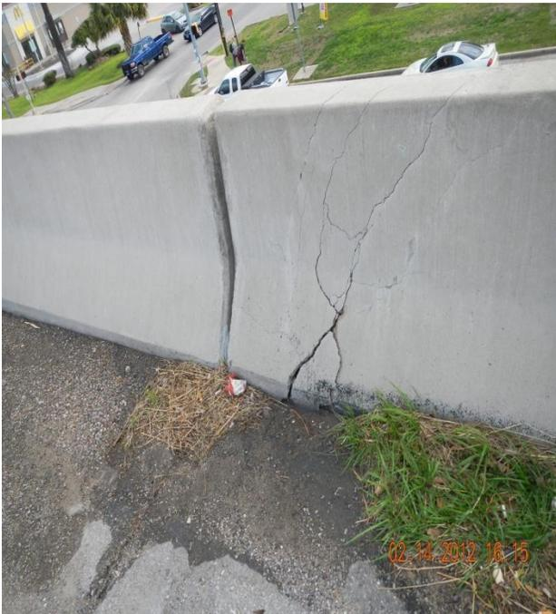
Figure 2.8 Damage in traffic rail
