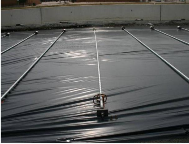
Figure 4.56 Polyethylene sheet placed between subbase and CRCP
