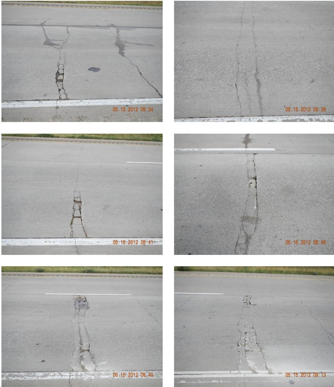
**Figure D.6 IH 35 Pavement Evaluation in the Laredo District – Pavement Condition (05/15/2012)**
