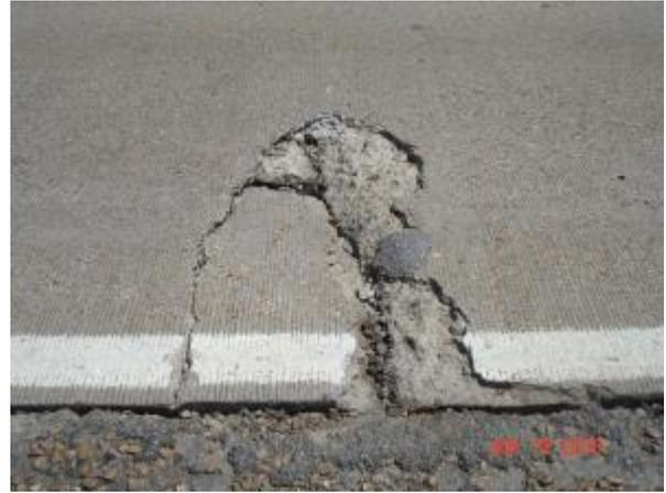
b. Distress in post-tensioned pavement
