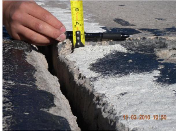
b. Joint separation and slab settlement
