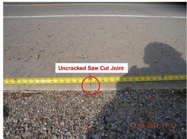
**Figure 5.34 Cracked and Uncracked Saw Cut Joints in Abilene Whitetopping Section (SH 226 at SH 279)**
