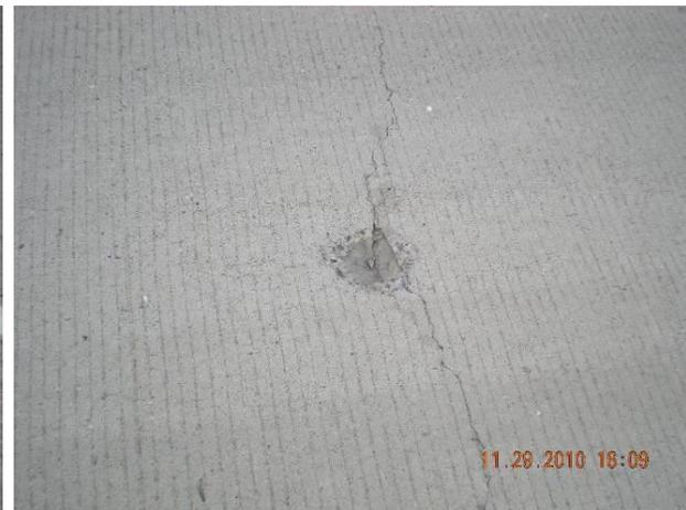
**Figure 4.34 Spalling Distress in Van Horn IH 10**
