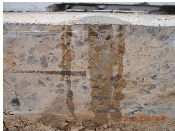
b. Tight crack width below the surface
