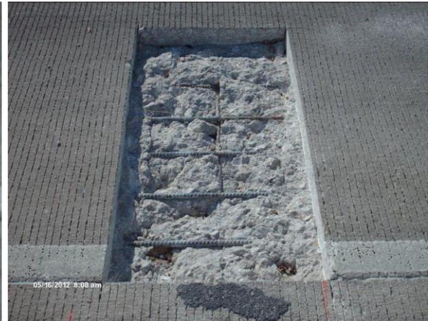
**Figure 5.24 Concrete after Removal of Distressed Concrete**
