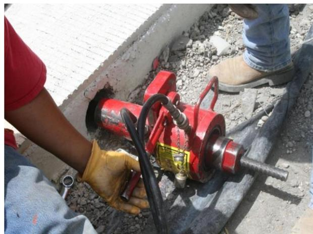
**Figure 5.9 Post-Tension (transverse)**
