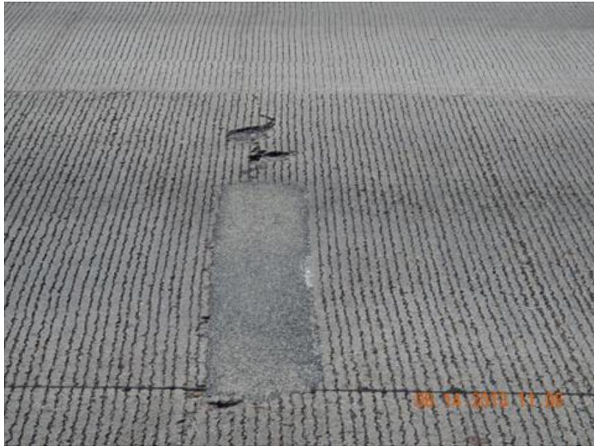
**Figure 4.8 Close-Up View of Spall Repairs**
