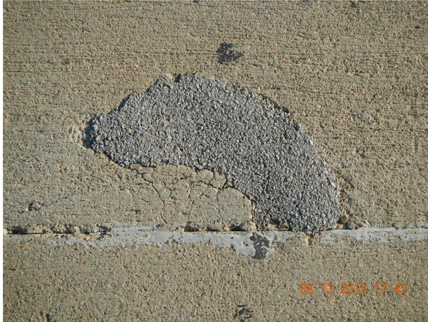
**Figure 5.14 Asphalt Concrete Patch at Joint (North)**
