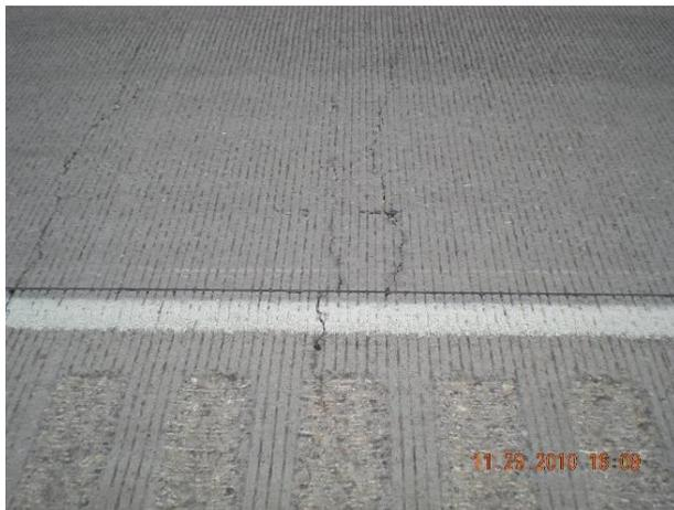
**Figure 4.33 Transverse Cracks in Van Horn IH 10**
