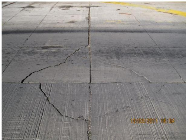
**Figure 5.31 Diagonal Failures in Abilene Whitetopping Section (SH 36 at FM 1750)**
