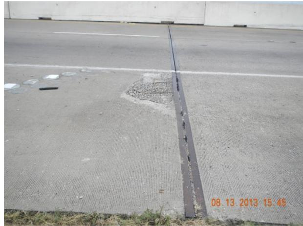
**Figure 5.6 Longitudinal Cracks (built in 1985) Figure 5.7 Joint Failure in Shoulder (built in 1985)**
