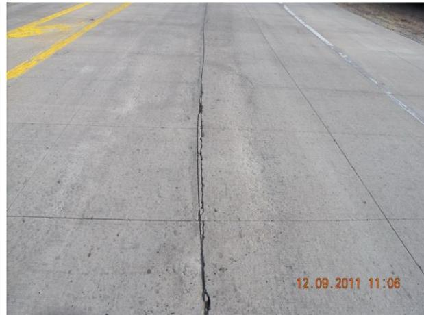
**Figure 5.33 Cracking along the Joints in Abilene Whitetopping Section (SH 226 at SH 279)**
