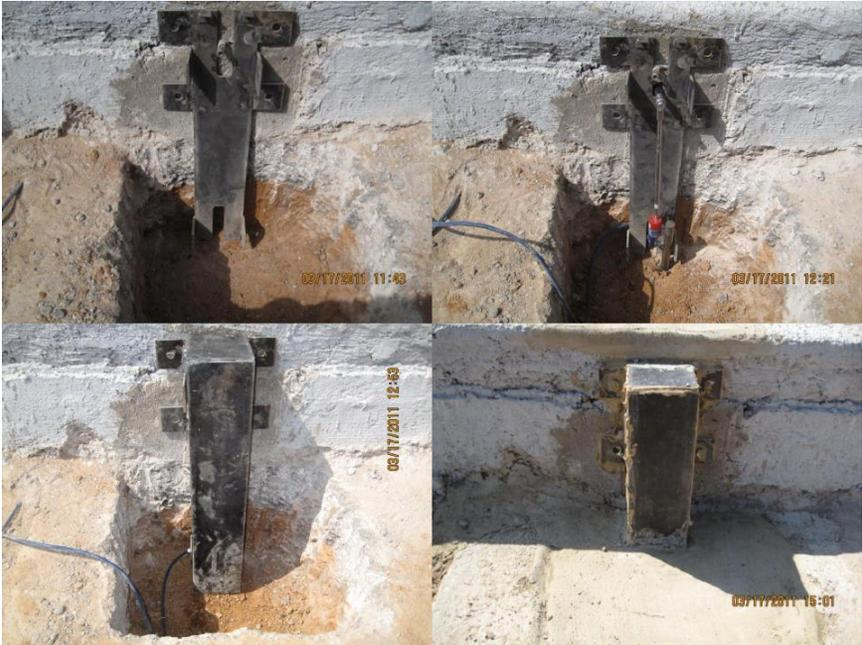
**Figure 3.1 Crackmeter Installation**
