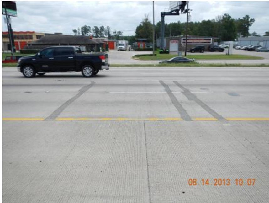
**Figure 4.14 Spalling Repairs in SRG Section**
