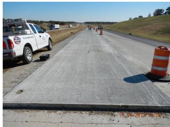
b. 4-in. bonded concrete overlay
