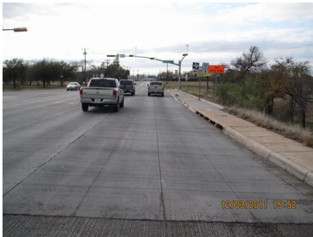
**Figure 5.30 Whitetopping in Abilene (SH 36 at FM 1750)**
