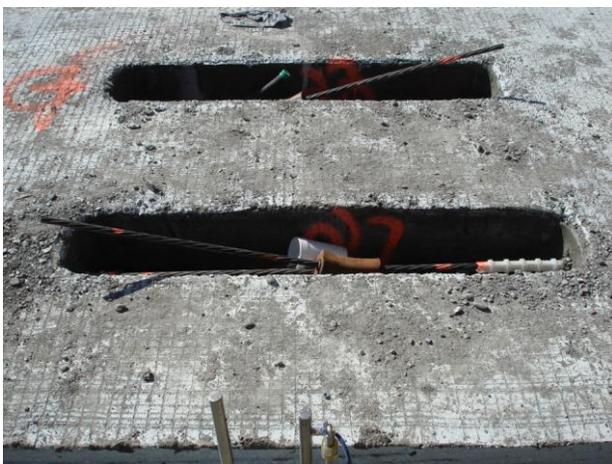
**Figure 5.8 Post-Tension (longitudinal)**
