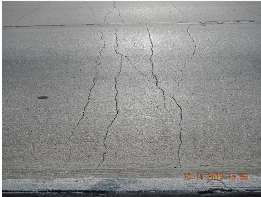
**Figure 2.18 Y-Crack and Narrow Crack on US 81 in the Wichita Falls District**
