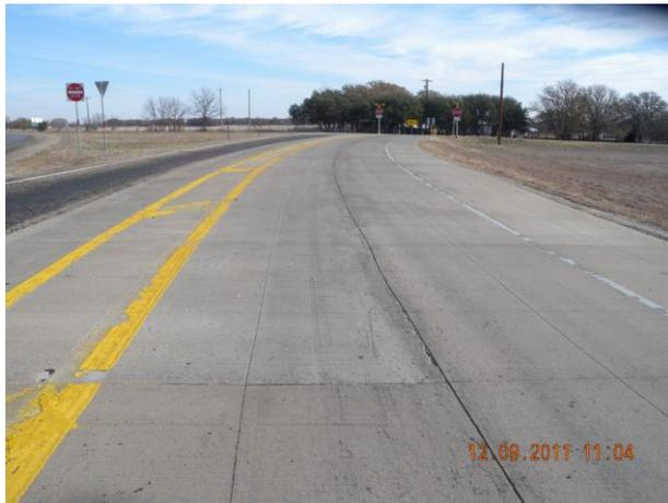
**Figure 5.32 Whitetopping in Abilene (SH 226 at SH 279)**
