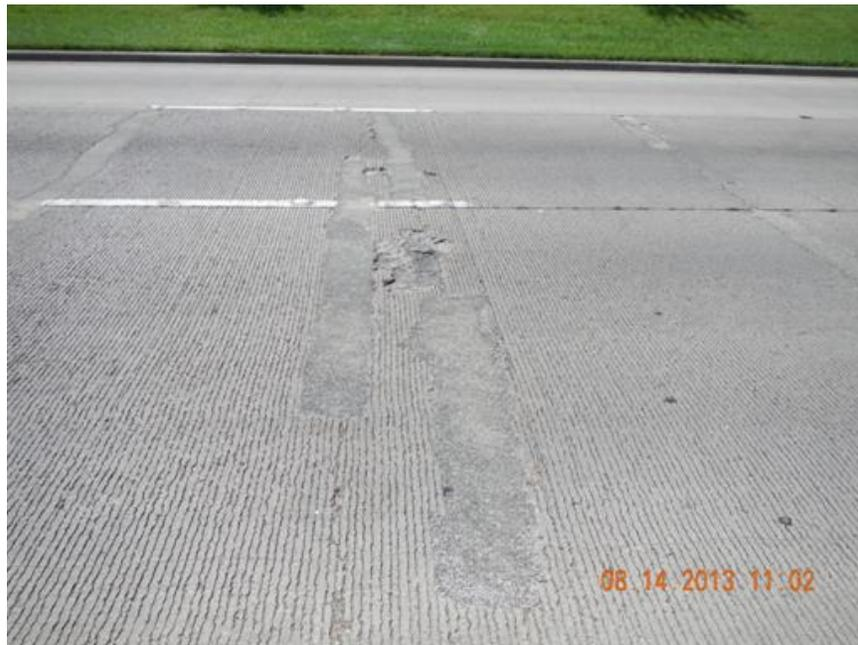
**Figure 4.7 Deep Spalling in SRG Section**
