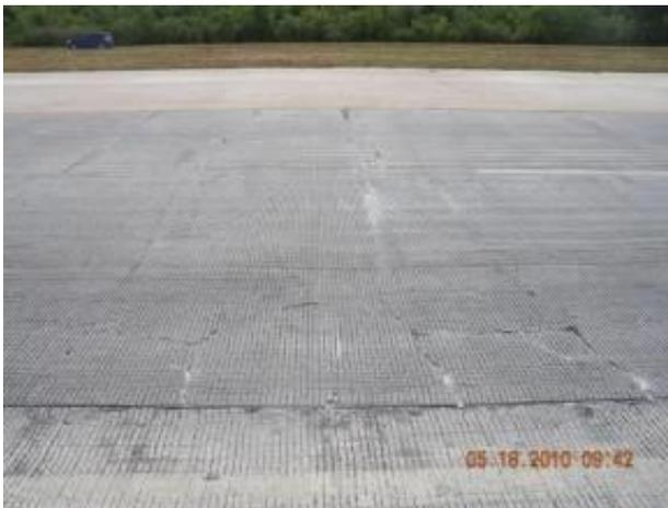
**Figure 5.25 Delaminations in BCO**
