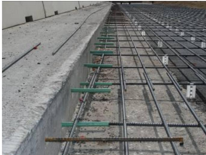
*Figure 2.2: Tied and doweled sections*
