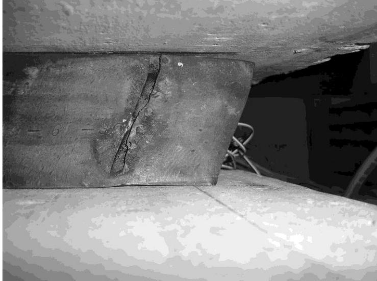
Figure 5.67 – Example of Observed Transverse Top Uplift
