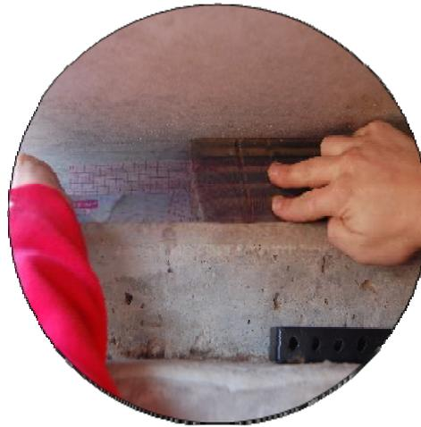
**Figure 1.1** – Typical Transverse Displacement on a Standard U-Beam Bearing
