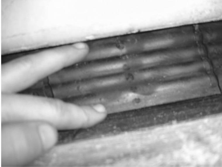
Figure 5.75 – Tension Debonding at Shims
