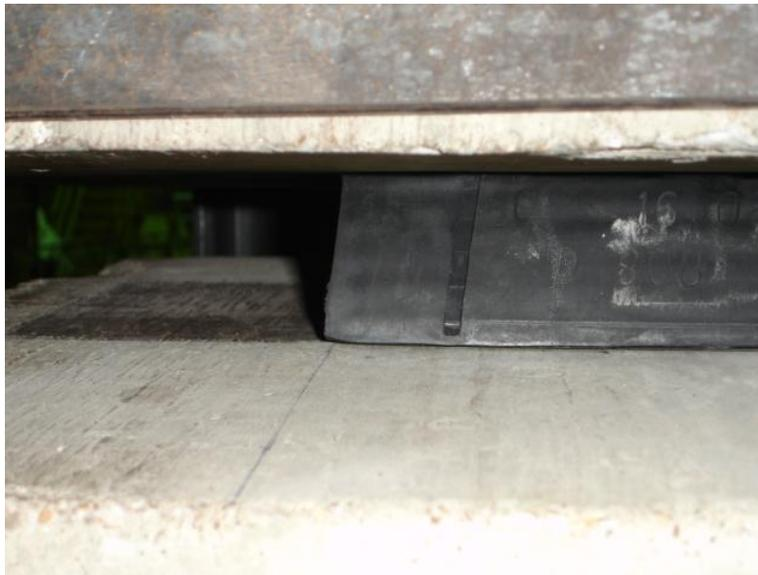
Figure 5.51 – Illustration of Slip, Transverse Front
