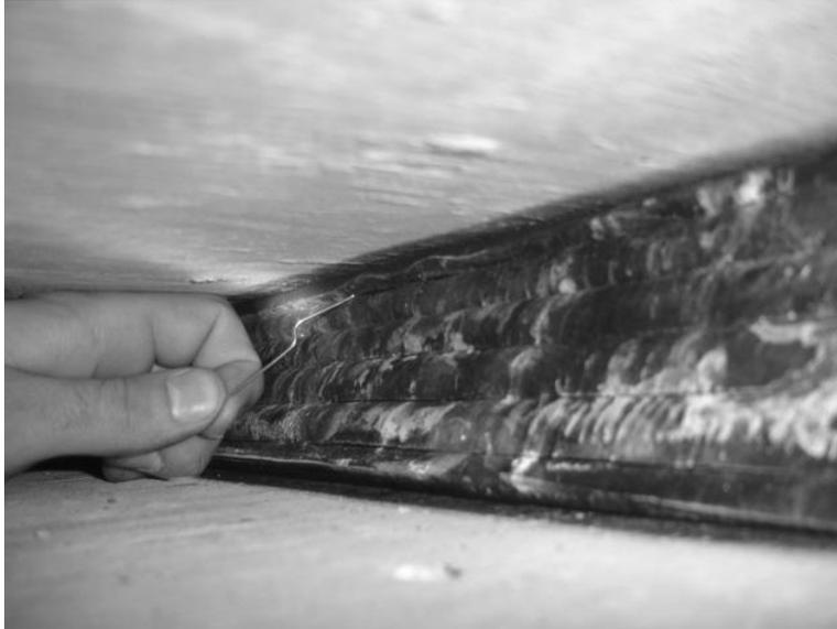
Figure 5.76 – Delamination of Elastomer
