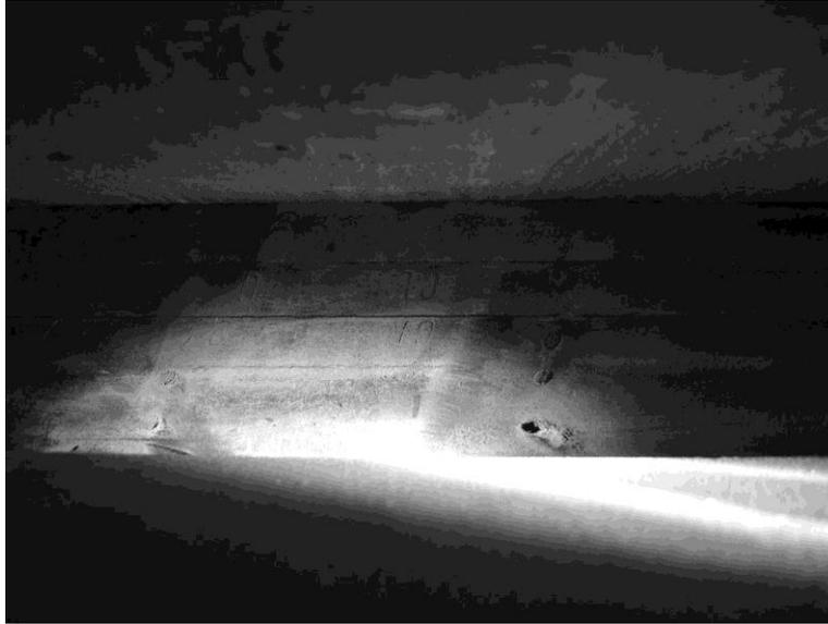
Figure 5.73 – Hairline Surface Cracks on Elastomeric Bearing
