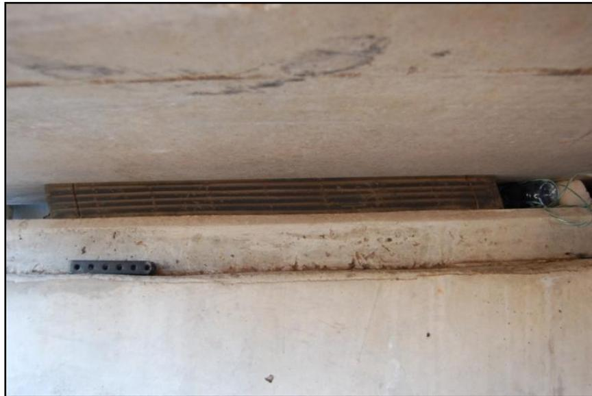
Figure 4.2 – Elevation of Bearing A
