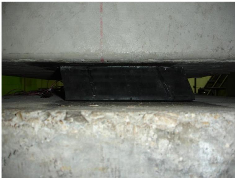
Figure 5.54 – Bearing Corner Undergoing Curling
