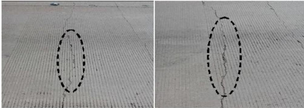
Figure 5.3 Low and Medium Severity Chipping, on US 290, Cypress
