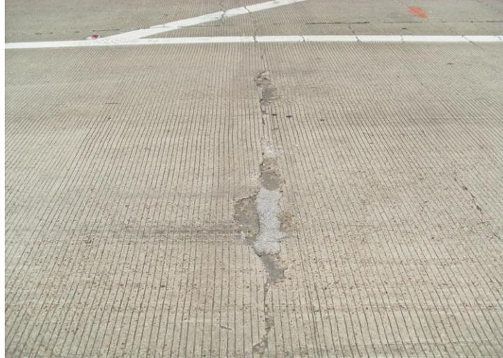
Figure 5.32 Medium Severity Spalling, SH 225
