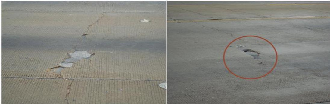
Figure 5.40 High Severity Spalling, FM 1960
