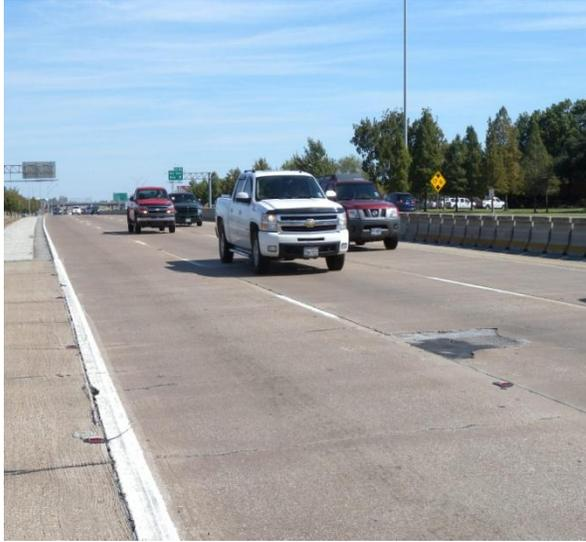
Figure 2.11-(a) Distress due to poor load transfer at longitudinal joint
