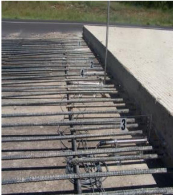
Figure 2.3-(a) Slab displacement measurement at transverse construction joint
