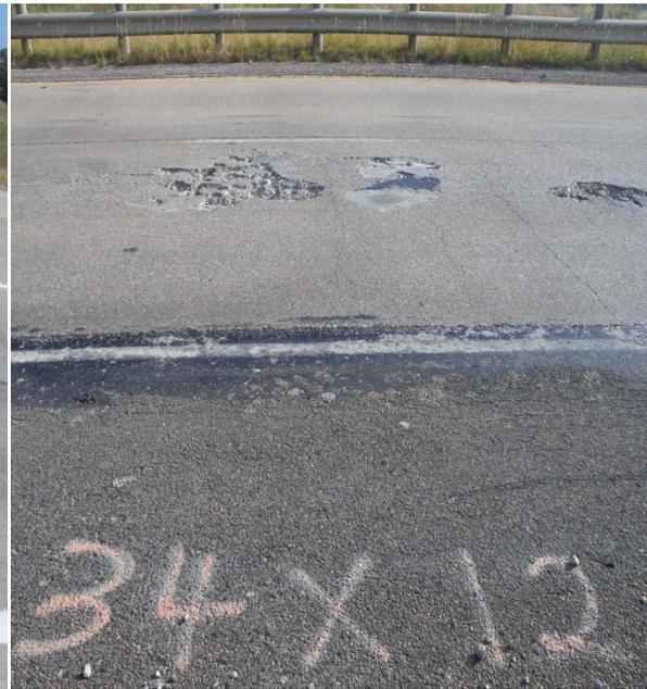
Figure 2.9-(b) CRCP distress due to construction quality issue
