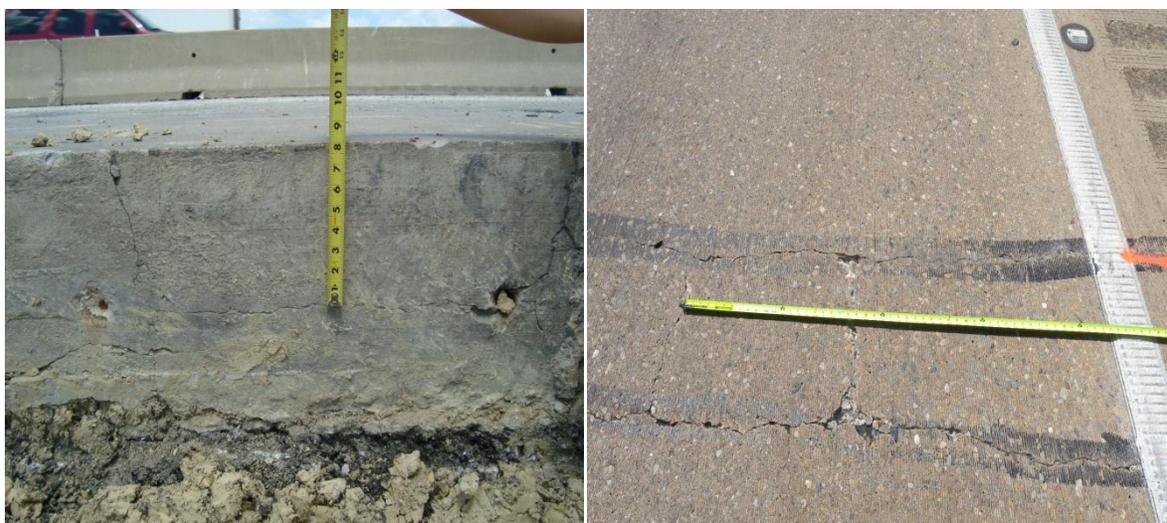
Figure 2.5-(a) Horizontal cracking on IH35 observed in 2010      Figure 2.5-(b) Distress due to horizontal cracking
