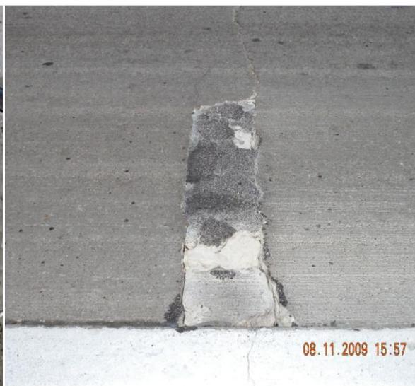
Figure 2.4-(b) Distress resulting from early age horizontal cracking
