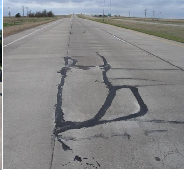
Figure 2.11-(b) Distress due to poor load transfer at longitudinal joint
