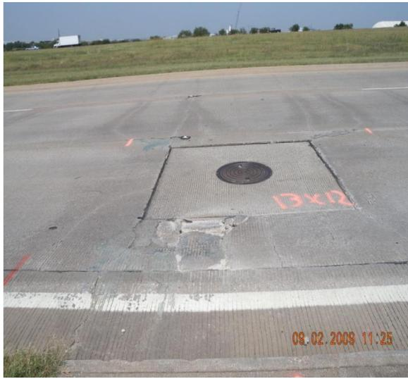
Figure 2.10-(a) Distress due to consolidation of subgrade/subbase
