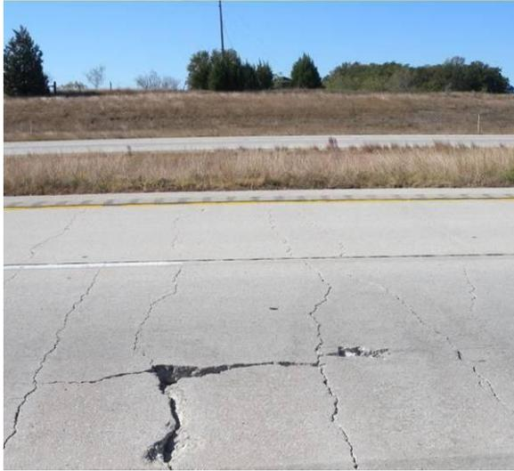
Figure 2.15-(a) Longitudinal crack due to poor slab support
