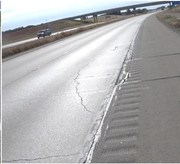
Figure 2.10-(b) Distress due to consolidation of subgrade/subbase
