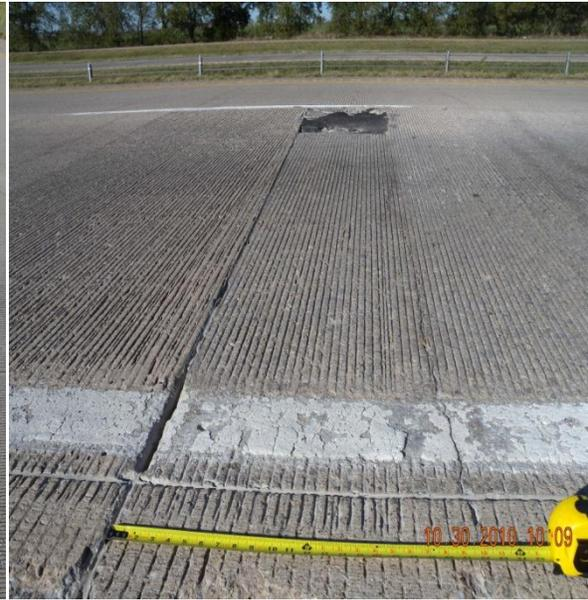
Figure 2.2-(b) Distress at transverse construction joint
