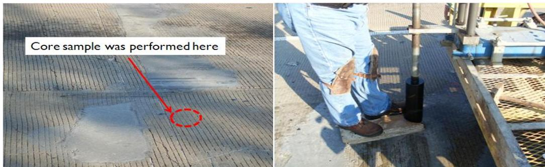
Figure C.1 Coring Site and Coring Equipment Setup in SH 1960
