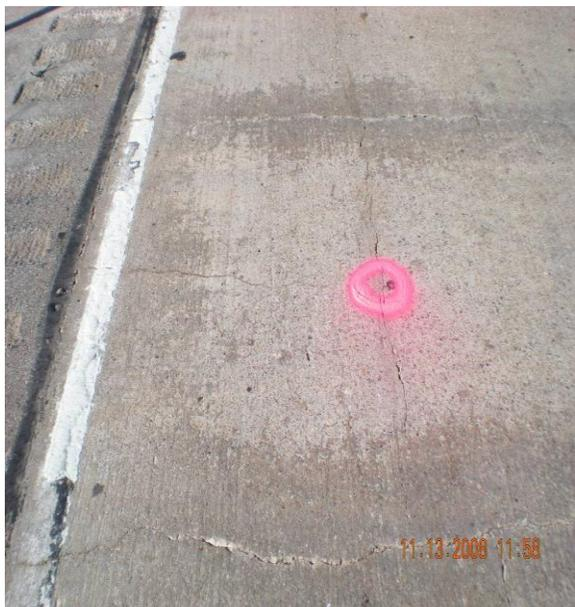
Figure 2.14-(a) Longitudinal cracking in the wheel path
