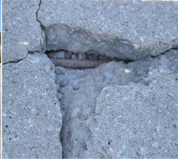
Figure 2.15-(b) Close-up view of longitudinal crack, showing steel
