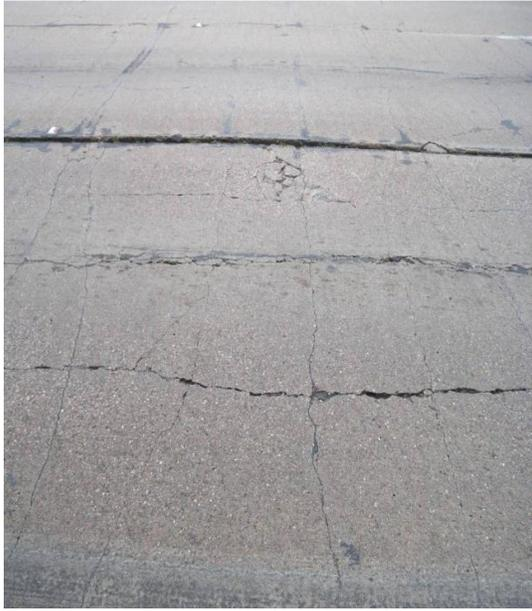
Figure 2.8-(a) Close-up view of distress in 6-in CRCP in Dallas
