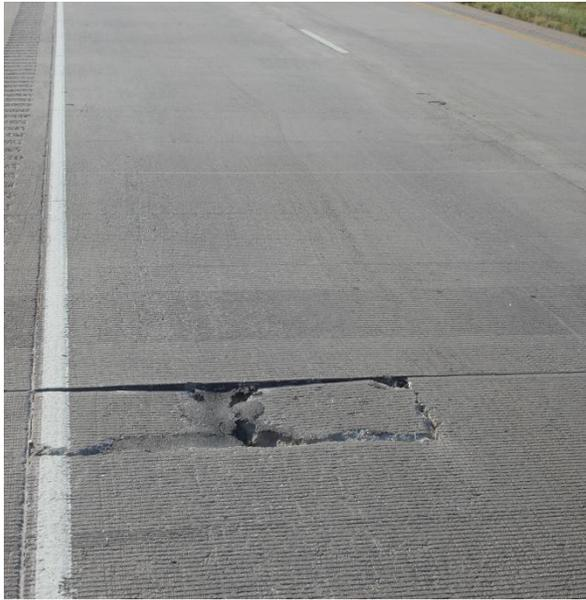
Figure 2.2-(a) Distress at transverse construction joint
