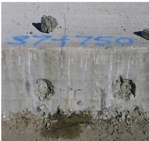
Figure 2.4-(a) Horizontal cracking observed on IH35 in 1999
