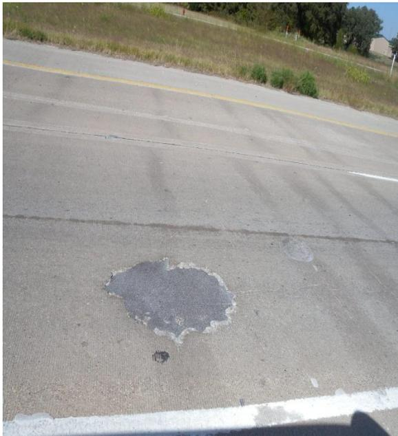
Figure 2.9-(a) CRCP distress due to construction quality issue
