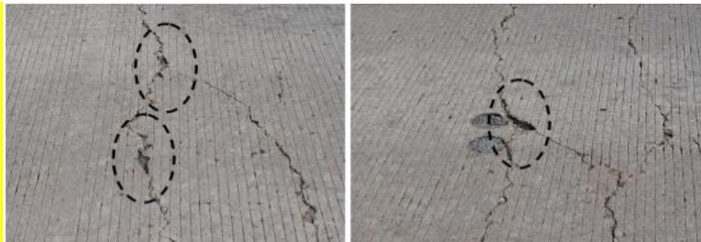
Figure 5.4 Low and Medium Severity Shallow Spalling, on US 290, Hempstead
