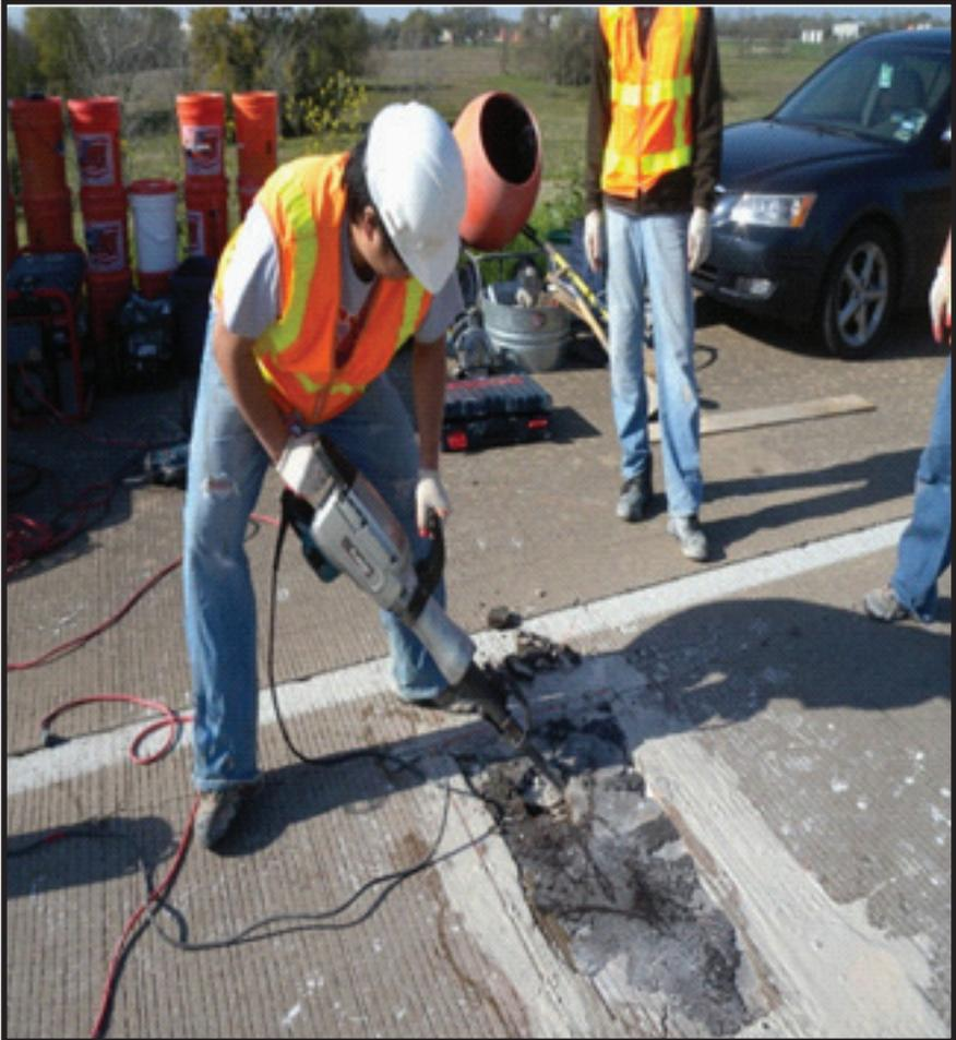
**Figure 9.** Removing concrete using a jackhammer
