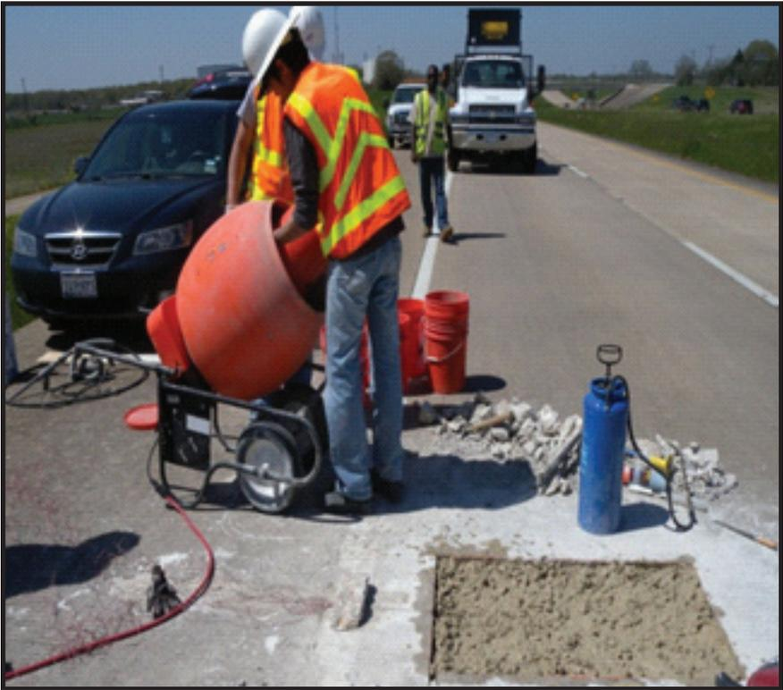
**Figure 11.** Mixing of prepared repair materials at the job site
