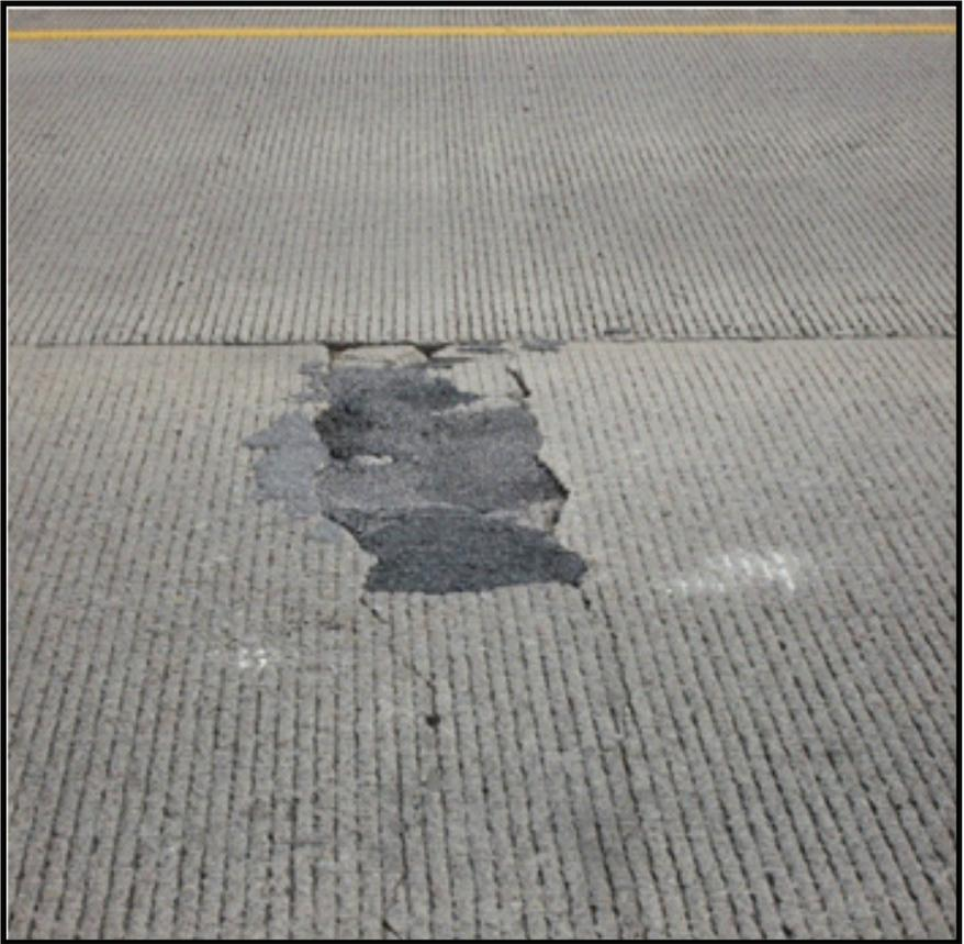
**Figure 1.** Partial depth distress near longitudinal construction joint
