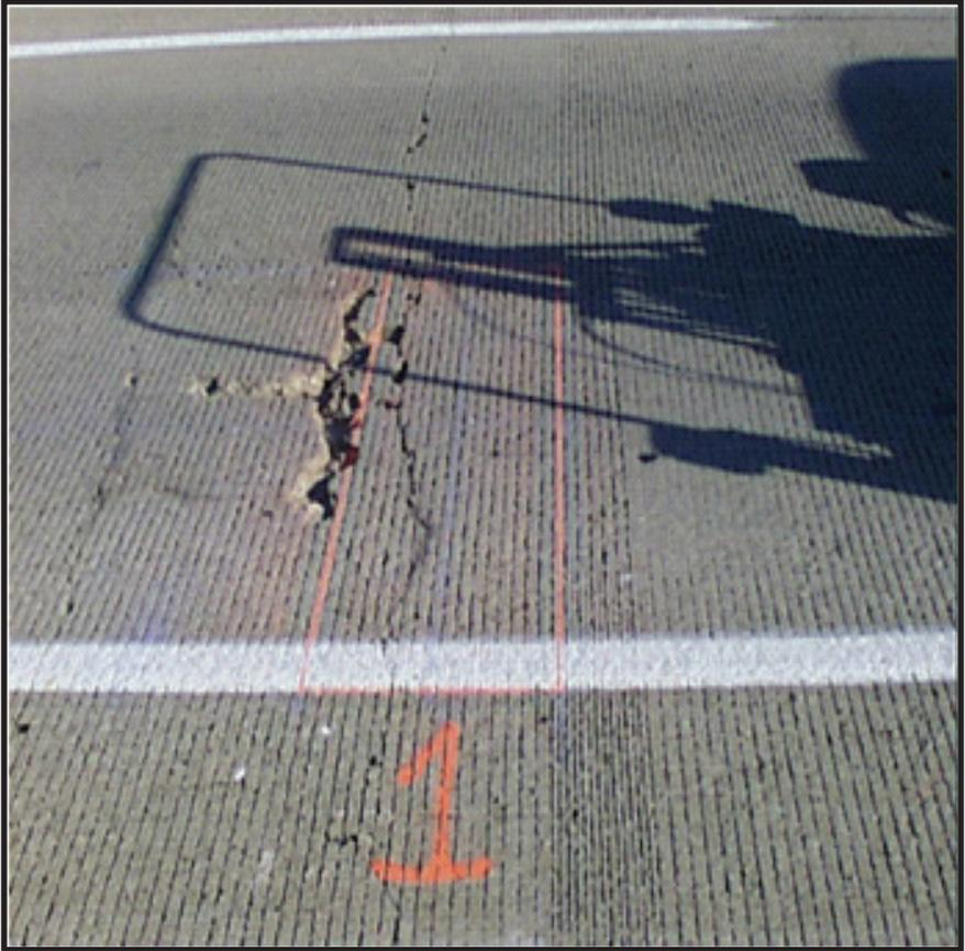
**Figure 6.** Partial depth distress under wheel path
