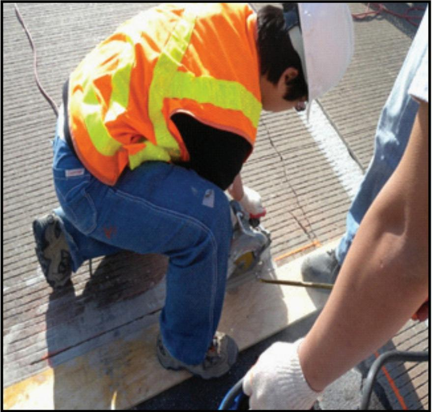
**Figure 8.** Saw cut operation
