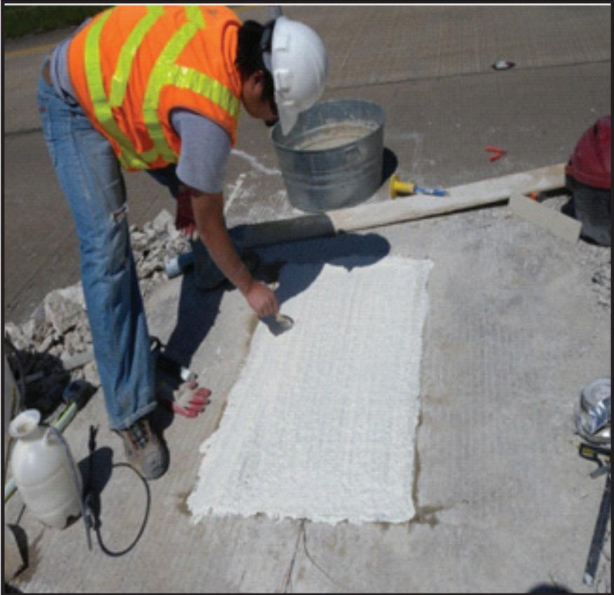
**Figure 12.** Application of sufficient curing compound
