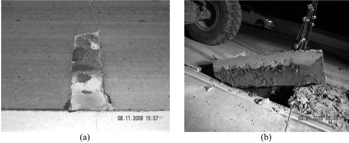
*Figure 2.2: CRCP distress caused by horizontal cracking*
