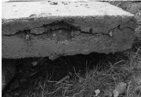
*Figure 2.4: Horizontal cracking in CRCP*
