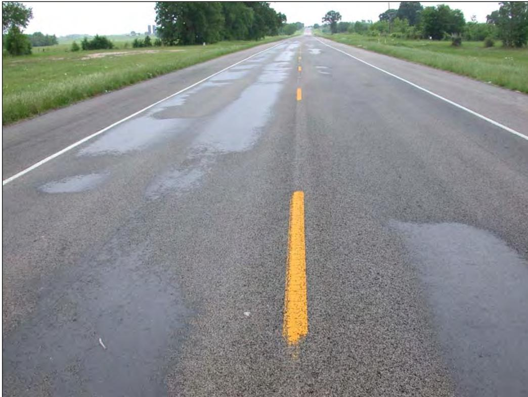
**Figure 3.4** Flushed Pavement
