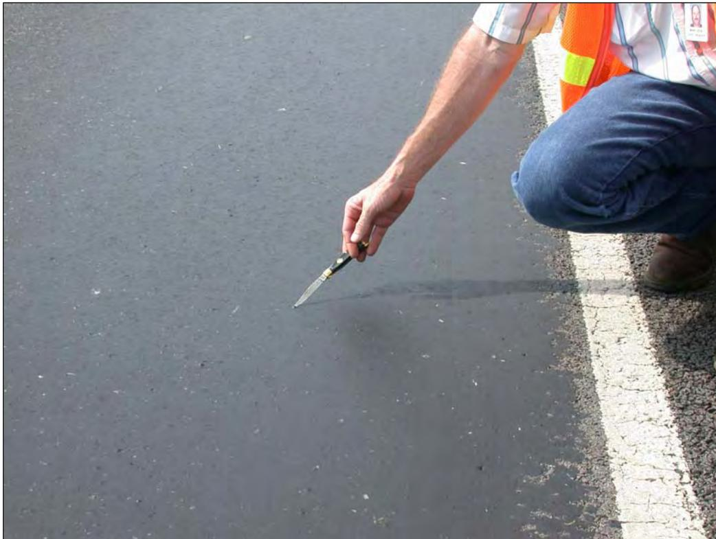
**Figure 3.5** Heavily Flushed Pavement
