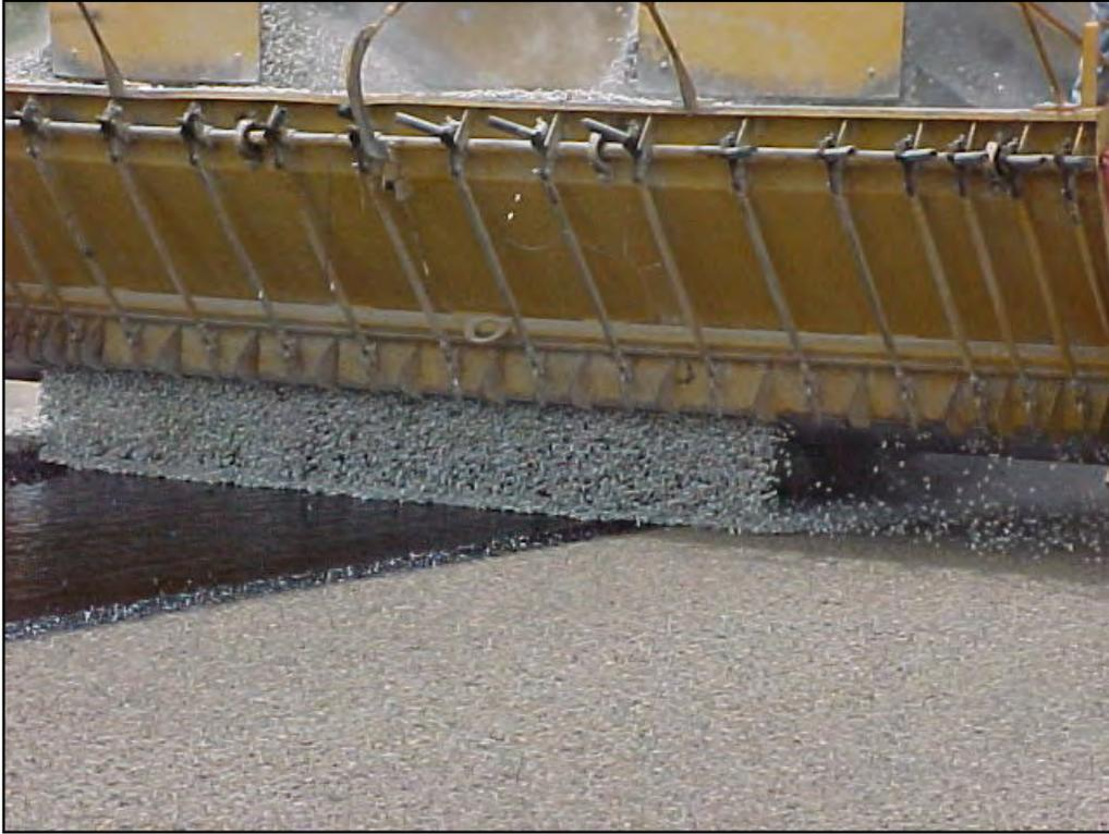
**Figure 6.5** Application of Grade 3 Seal Coat Aggregate
