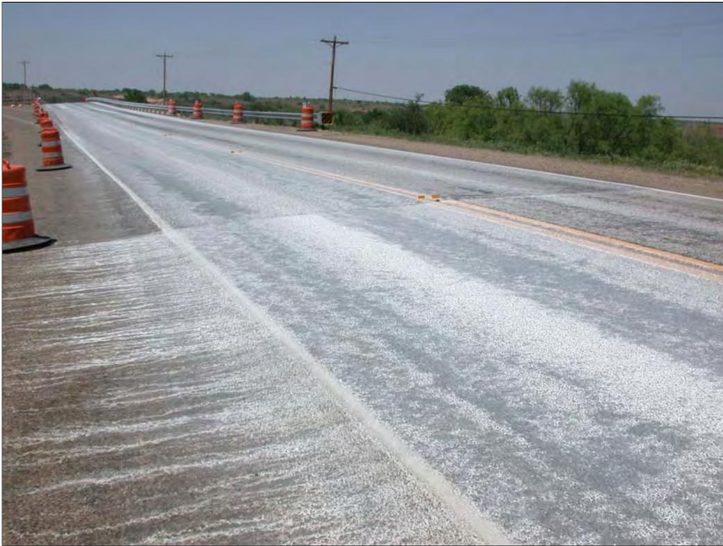
**Figure 6.12** The Lime Application Rate Should Achieve Good Splatter (Dosage) of Lime Water Solution on the Affected Pavement Surface
