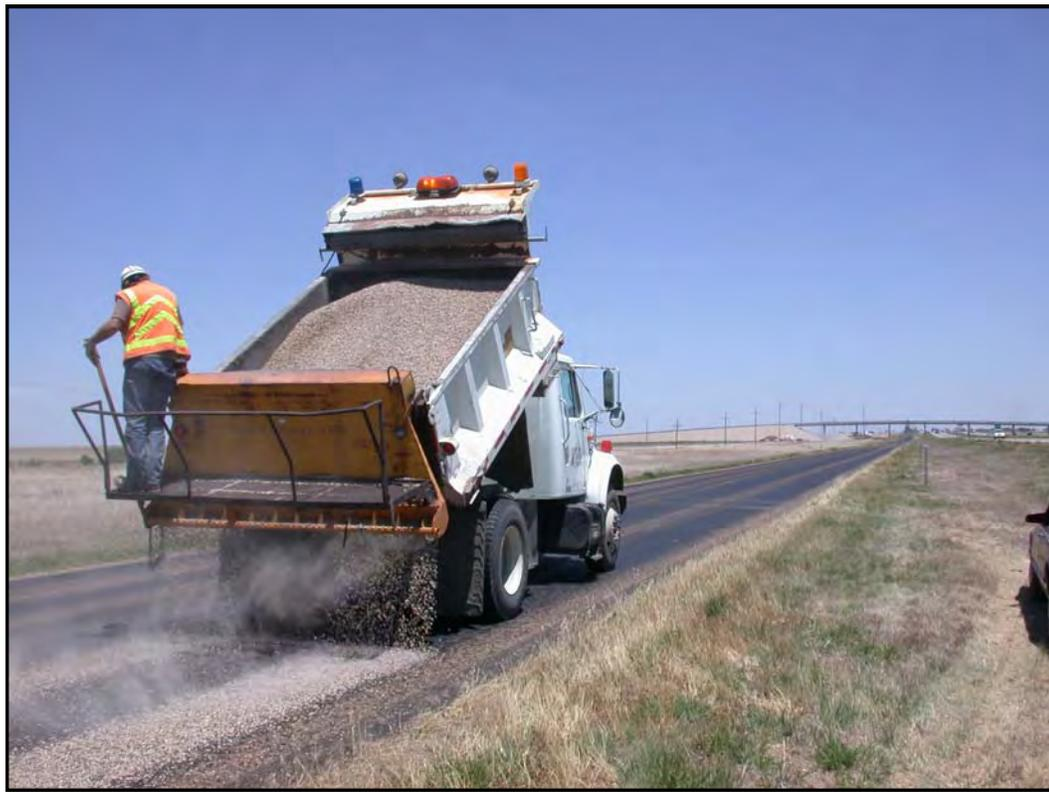
**Figure 6.1** Applying Small-Size Aggregate to Treat Bleeding Pavement
