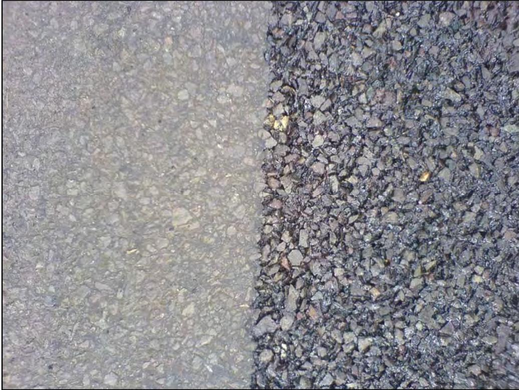
**Figure 7.9** Ultra High Pressure Watercutting Allows Effective Removal of Excess Asphalt Binder *Source:* Fulton Hogan, Ltd. [[www.fh.co.nz](http://www.fh.co.nz)]
