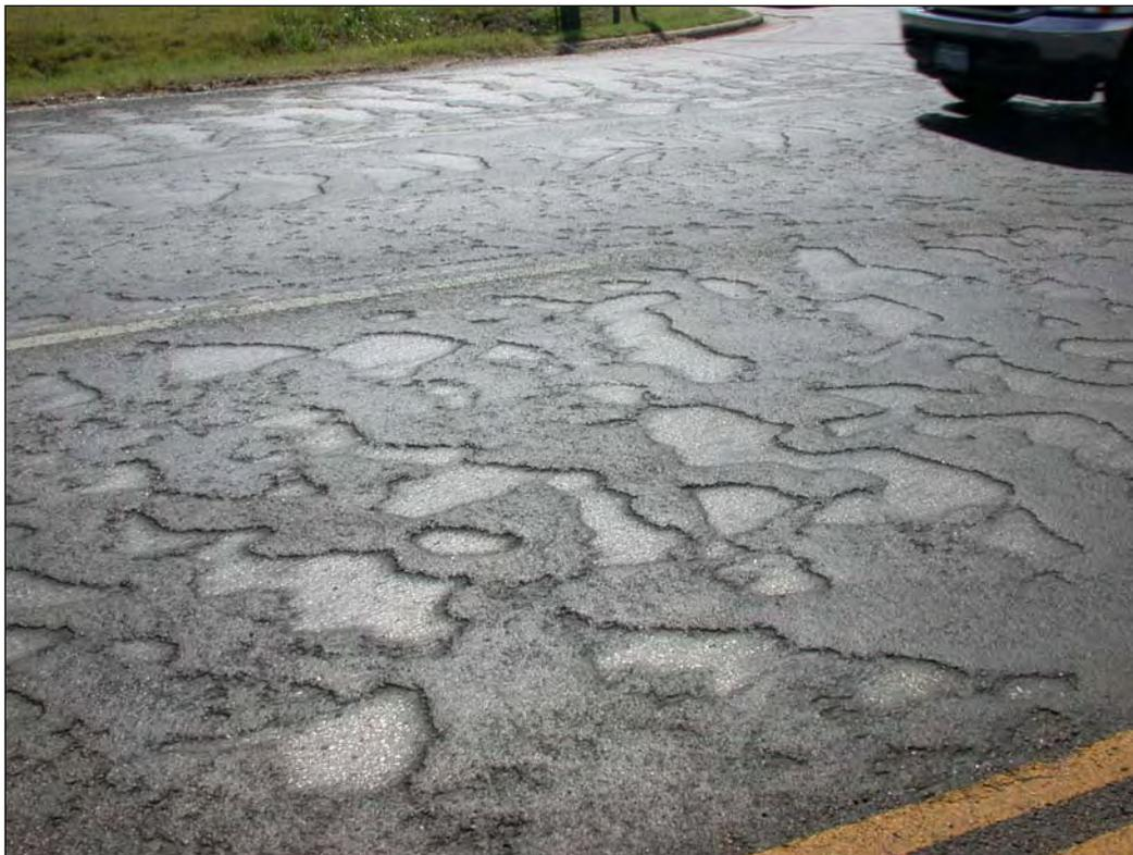
**Figure 4.3** Pavement Distress Caused by Starting/Stopping and Turning Maneuvers
