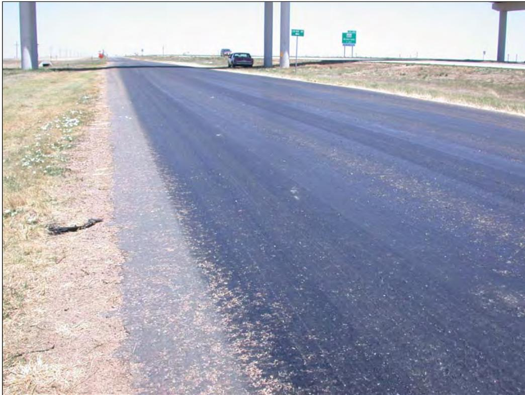
**Figure 3.2** Bleeding Asphalt Caused by Excessive, Heavy Truck Traffic and Hot Weather
