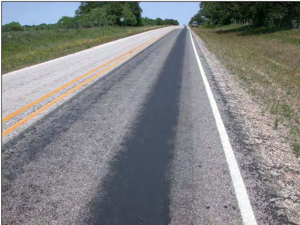
**Figure 4.1** Flushing in Wheel Paths
