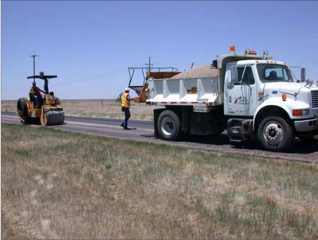
**Figure 6.3** Application of Grade 5 Aggregate to Treat Bleeding
