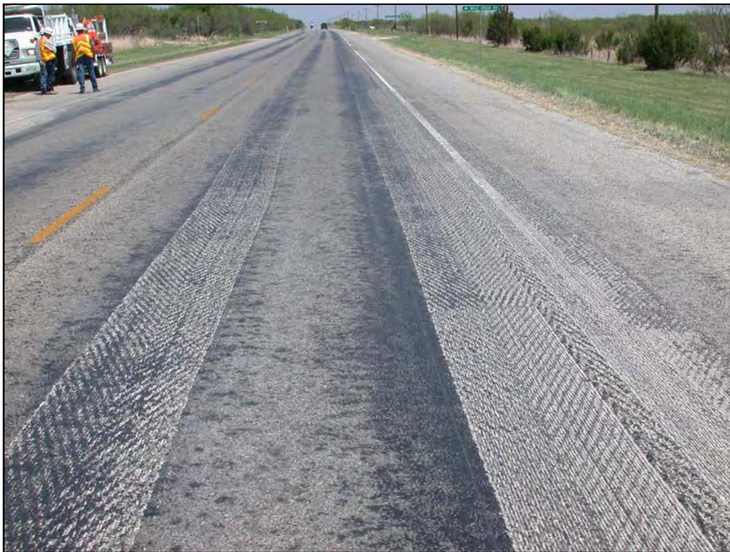
**Figure 7.2** Cold Milling Yields a Grooved Surface Texture Along the Longitudinal Axis of the Roadway
