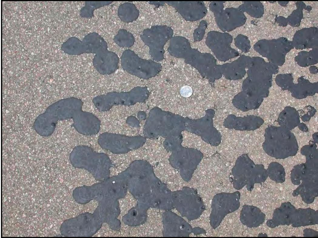
**Figure 7.5** Excess Asphalt from Flushed Pavement Can Work Its Way Through Microsurfacing
