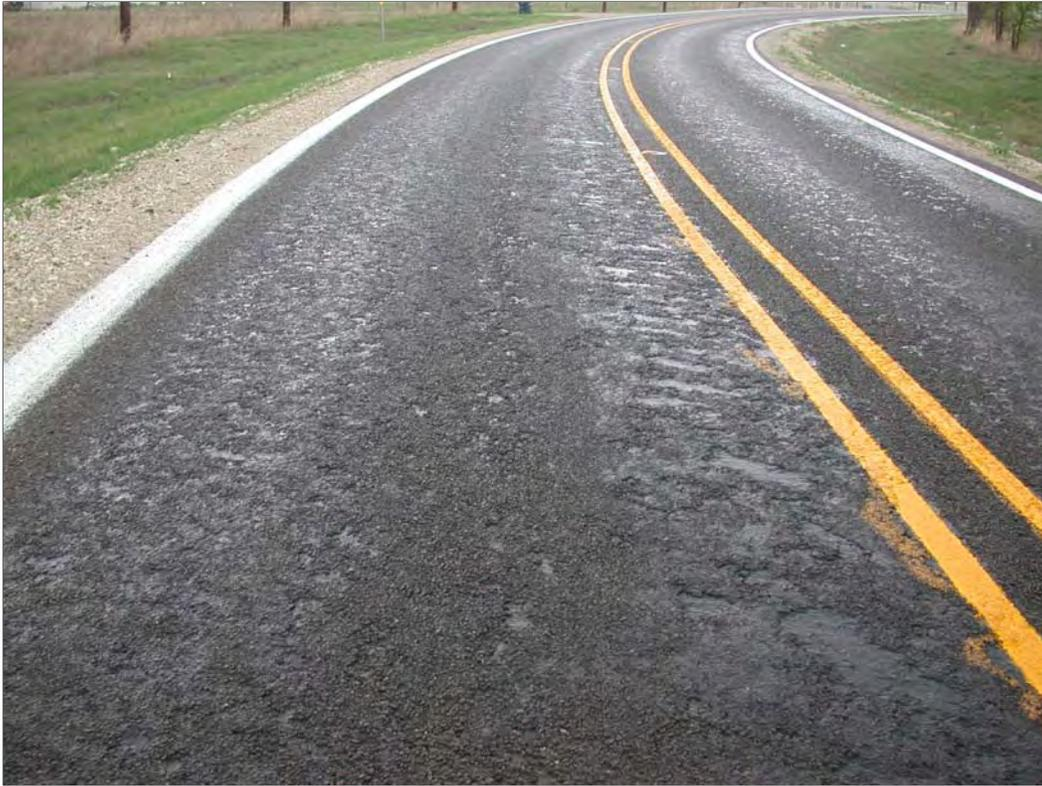
**Figure 6.15** Removal and Replacement May Be Necessary When a Fresh Seal Coat Totally Fails
