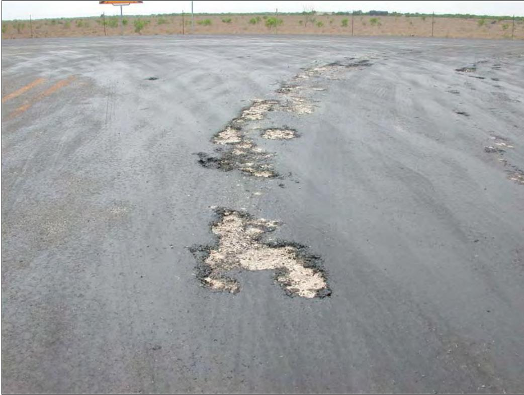
**Figure 3.3** Pavement Damage – Picking Up of Seal Coat – Caused by Bleeding
