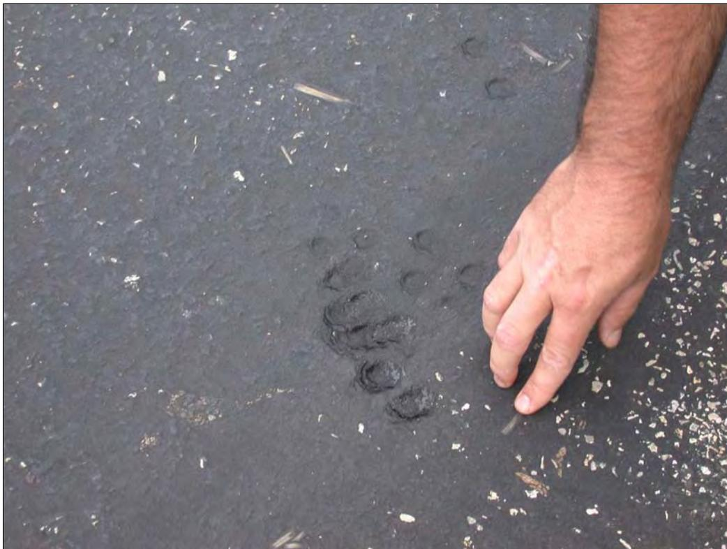
**Figure 4.4** Soft Pavement (Flushing) Resulting From High Temperature/Humidity
