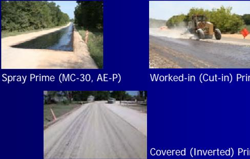
Spray Prime (MC-30, AE-P)      Worked-in (Cut-in) Prime
