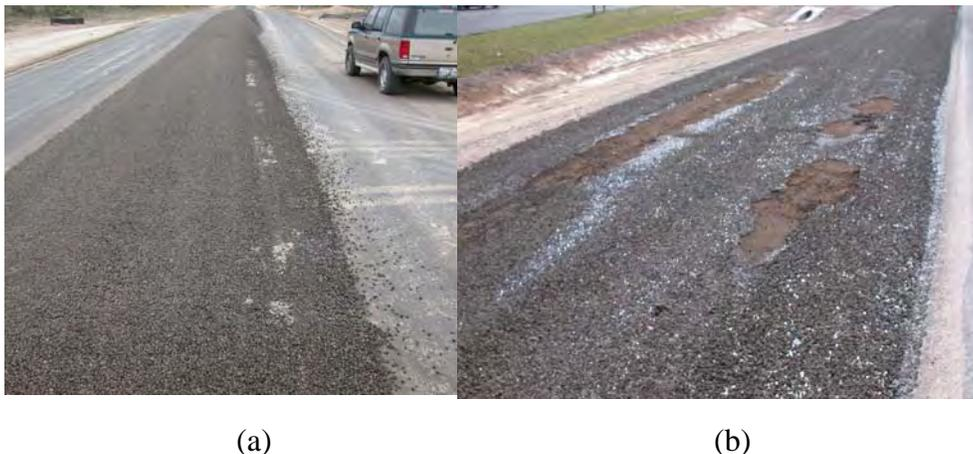
**Figure 4.14** Peeling of Surface Treatment During Construction
