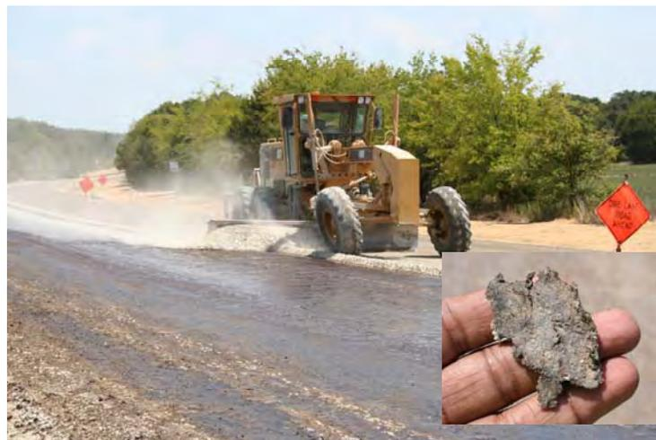
**Figure 4.7** Application of Worked-In (Cut-In) Prime on Limestone Base
