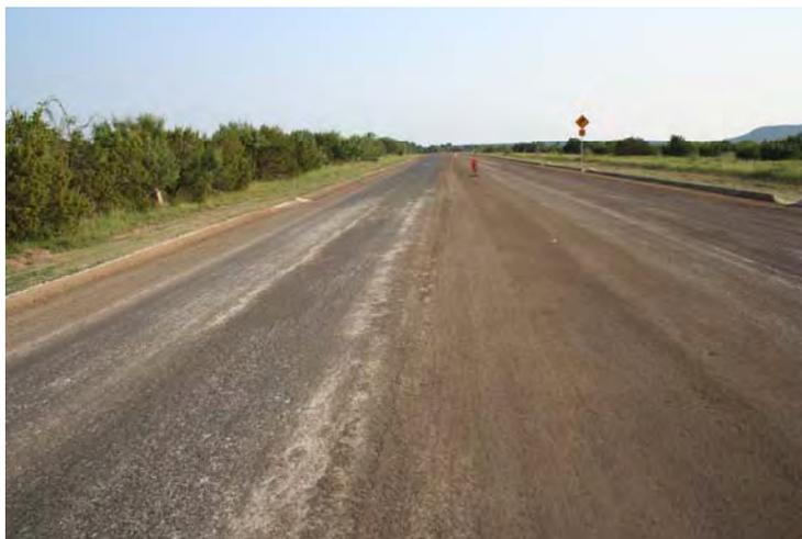
**Figure 4.12** Damaged Prime Coat Due To Water-Logging
