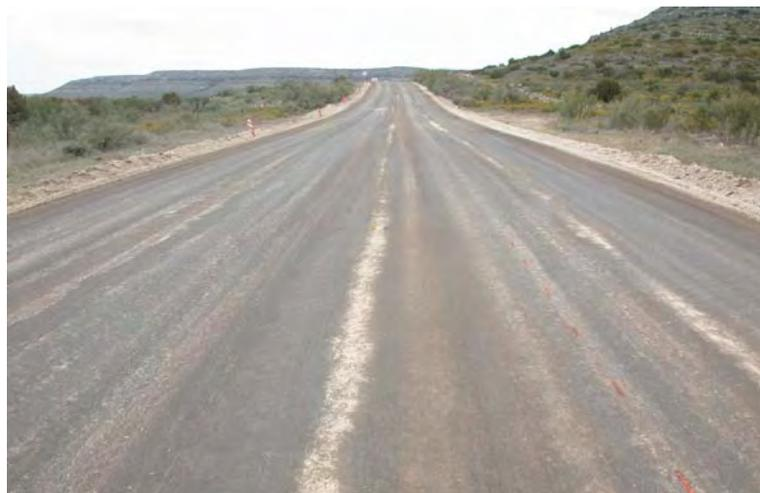
**Figure 4.11** A Prime Coat Worn Out Due To Excessive Exposure To Traffic
