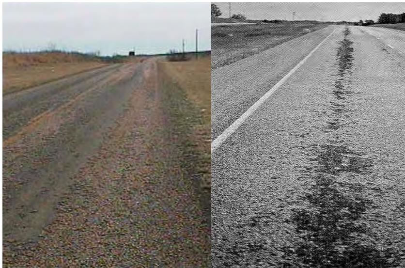
**Figure 4.16** Raveling (rock loss in surface treatments)
