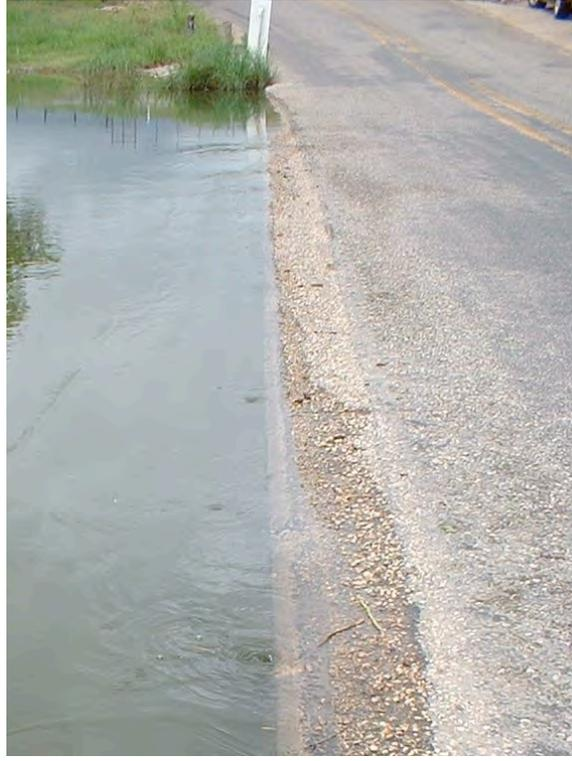
Figure 2.4: US 374 Northwest from Telegraph, Texas (between Junction and Rocksprings, Texas). Image is on a tributary of the South Llano River. Notice the vortices near the front left of the image at the water-roadway interface.
