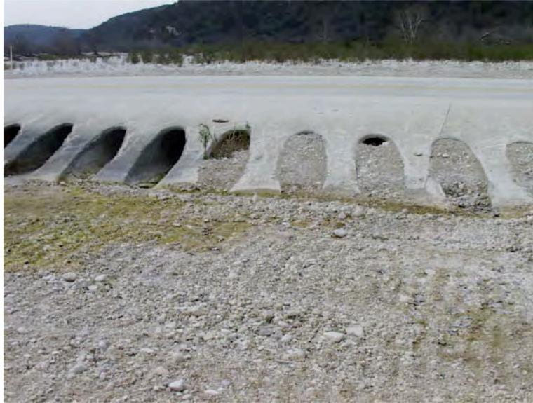
Figure 2.2: RR 335 at Ben Williams Ranch crossing Nueces River about 12 miles northeast from Barksdale, Edwards County, Texas. (Near the Real County line). Upstream side near river. All culverts have gravel deposit except for the southern four culverts which currently (03-09-2003) are passing flow. The other culverts also pass some flow, but behave as porous medium.
