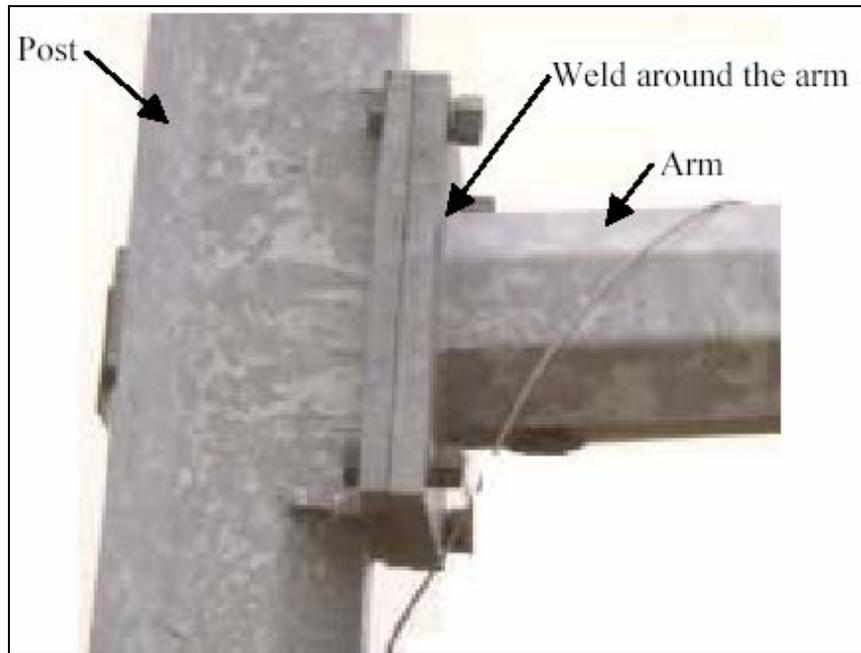
Figure 2.12. Typical Arm-Post Connection used by MoDOT (Chen et al. 2001)
