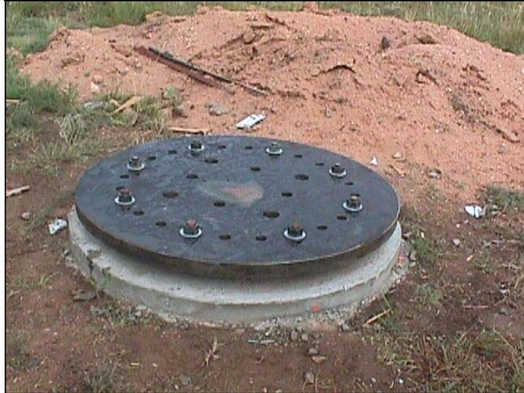
Figure 3.5 Foundation with Steel Plate
