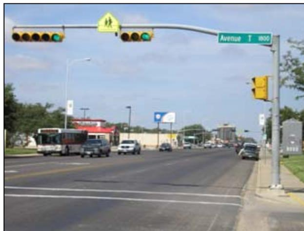
Figure 1.2 Cantilever Traffic Signal Structure with Bent Mast Arm
