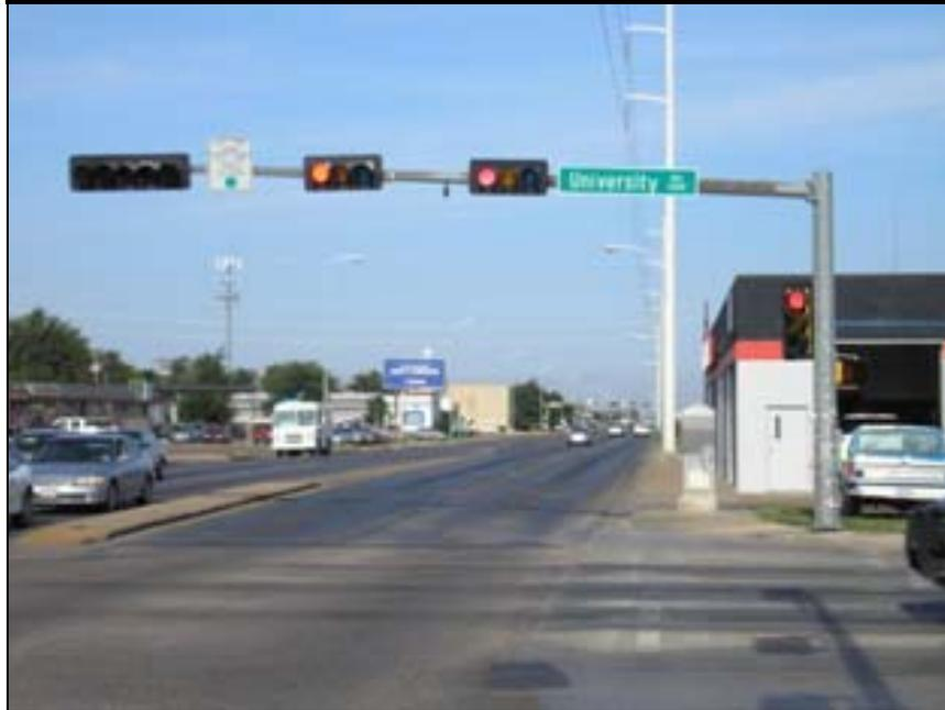
Figure 1.1 Cantilever Traffic Signal Structure with Straight Mast Arm
