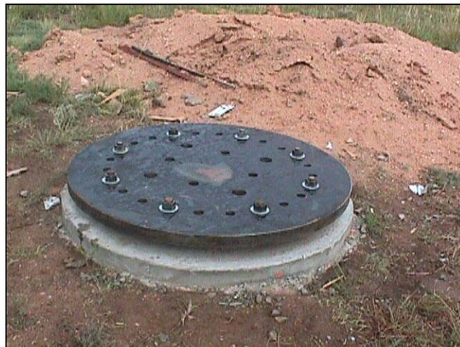
**Figure 2.** Foundation of Steel Plate Allowing Rotation of Mast/Arm Assembly
