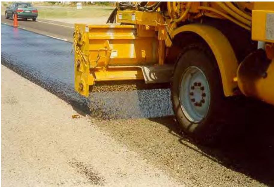
**Figure 2-1** Typical Seal Coat Operation
