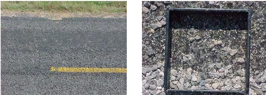
**Figure 3-5** Illustration of Rock Loss due to Aggregate-Binder Incompatibility
