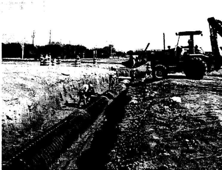
**Figure 5.17** Backfill Placement and Compaction.
