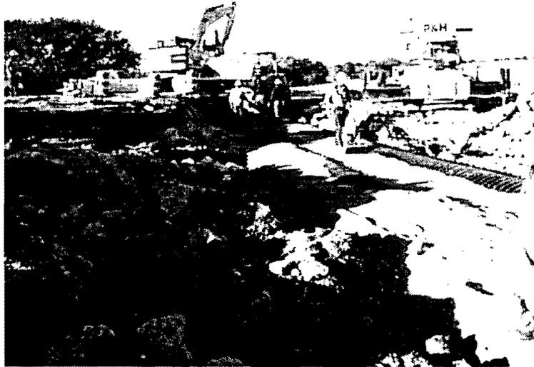
**Figure 5.6** Pipe with Backfill up to the Crown.
