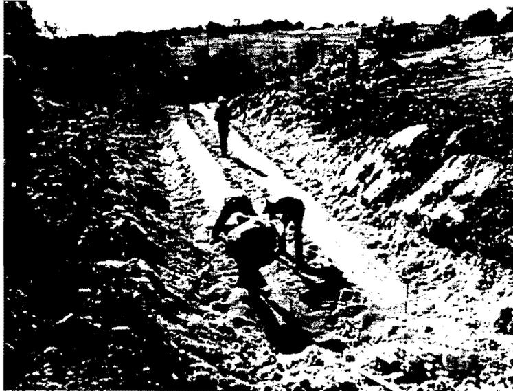
**Figure 5.4. Shaping of the Bedding.**
