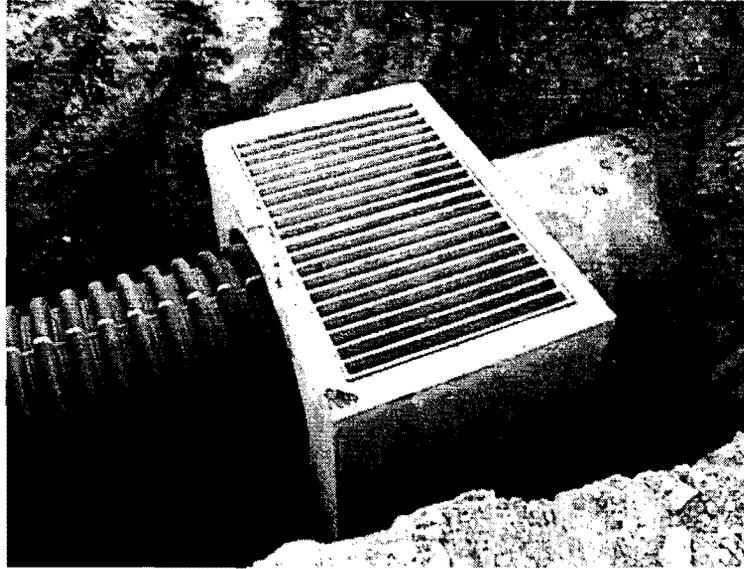
**Figure 5.16** Existing Concrete Catch Basin and HDPE Pipe.
