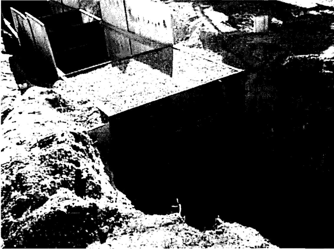
**Figure 4.13.** A Pipe Section Backfilled and Ready for Loading.
