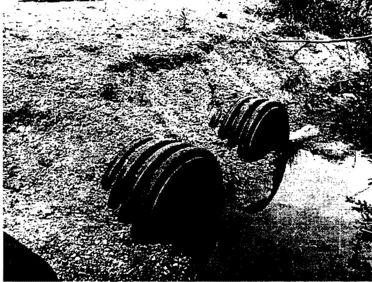
**Figure 5.32** Erosion in Installation A1 in Atlanta District.
