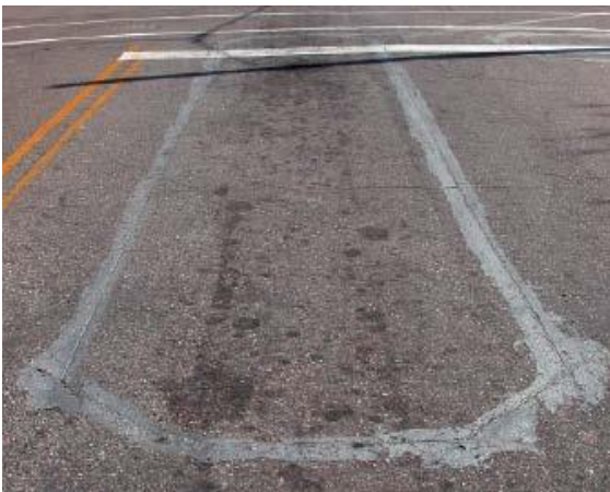
Figure 1.2.1 An example of inductive loop detector
