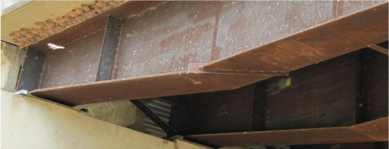
**Figure 4.2. Tapered End Section.**
