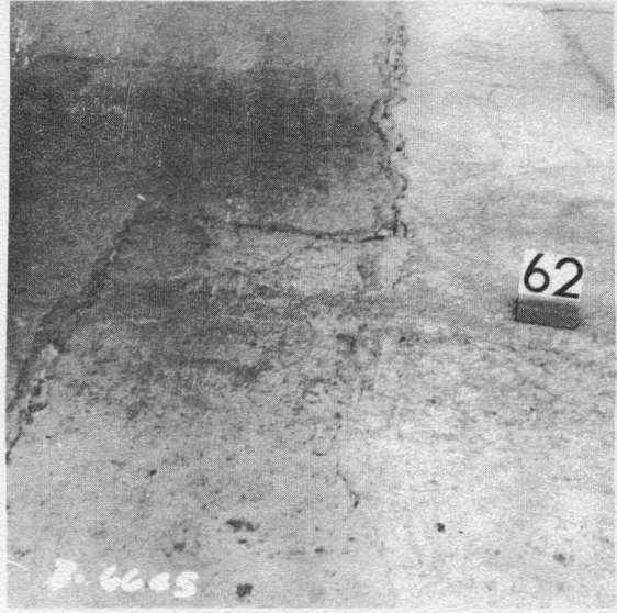
Figure A-14. Repair Area. SBL Station 331+
