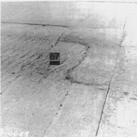
Figure A-19. Repair Area at Construction Joint. NBL Station 310+
