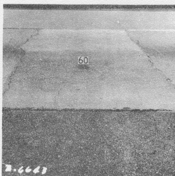
Figure A-12. Repair Area. SBL Station 405+
