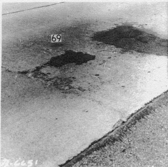
Figure A-21. Repair Area with Cold Mix and Concrete. NBL Station 353+
