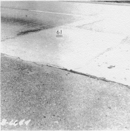
Figure A-13. Repair Area. SBL Station 387+
