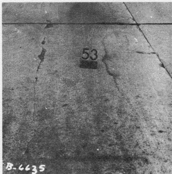
Figure A-4. Failure Near Construction Joint. SBL Station 511+
