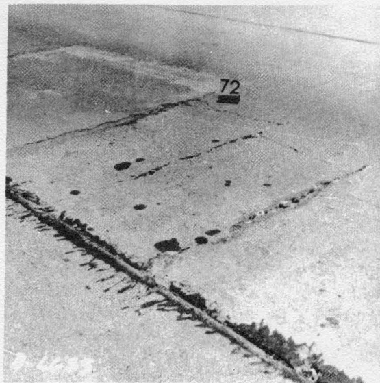
Figure A-24. Repair Area and Failure due to Honeycombing. NBL Station 425+
