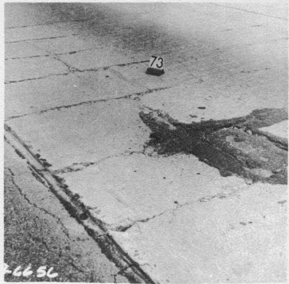
Figure A-26. Repair Area and Failure due to Honey-combing. NBL Station 520+
