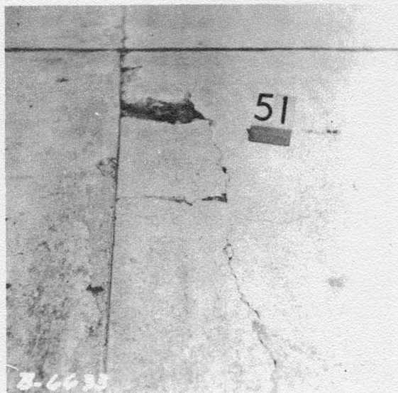
Figure A-2. Failure at Con- struction Joint SBL Station 530+
