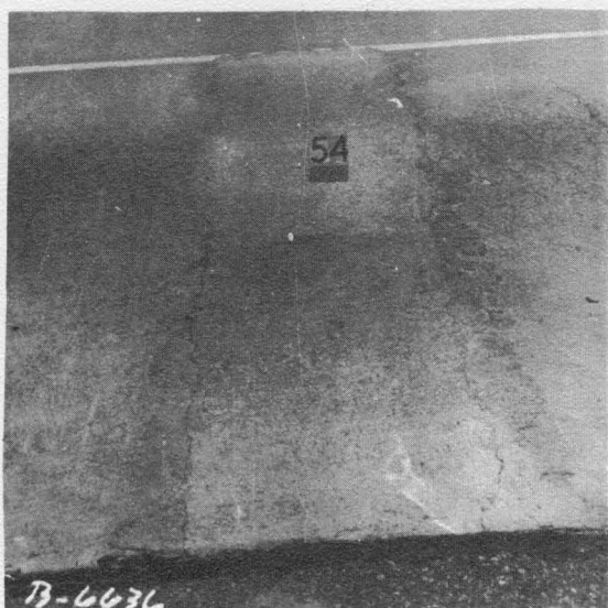
Figure A-5. Repair Area. SBL Station 508+
