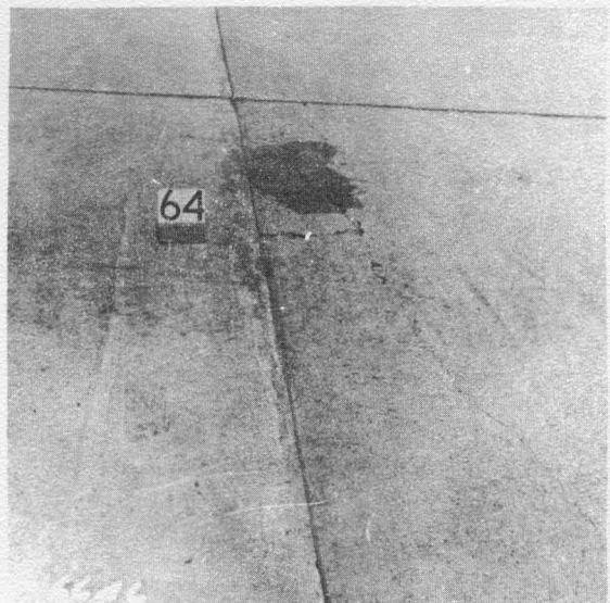
Figure A-16. Repair Area with Cold Mix Construction Joint SBL Station 98+
