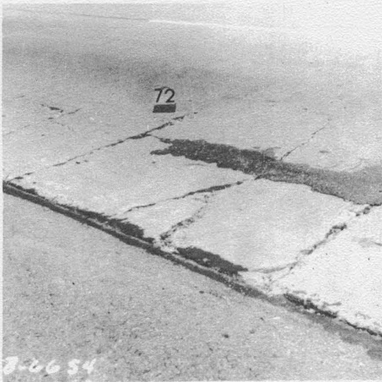
Figure A-25. Repair Area and Failure due to Honey-combing. NBL Station 425+
