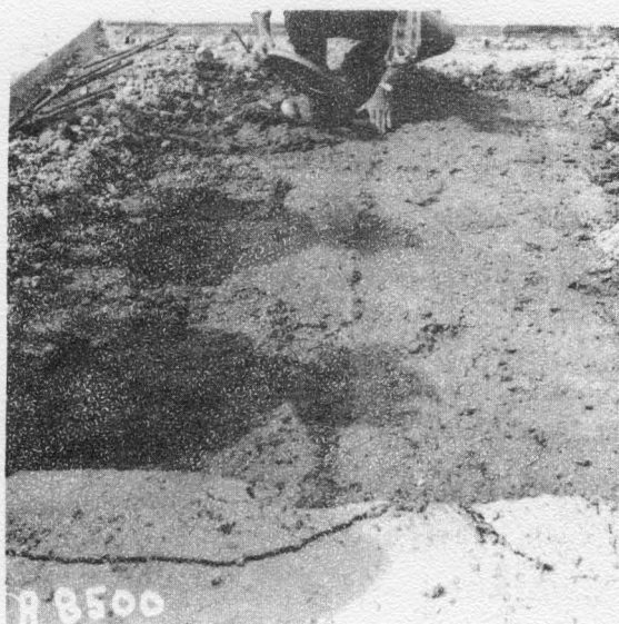
FIGURE B-5 Base Immediately after Re- moving Slab
