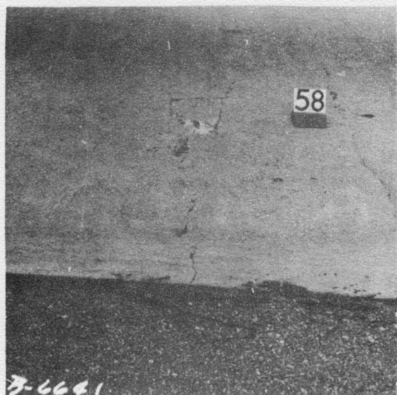
Figure A-9. Failure. SBL Station 441+
