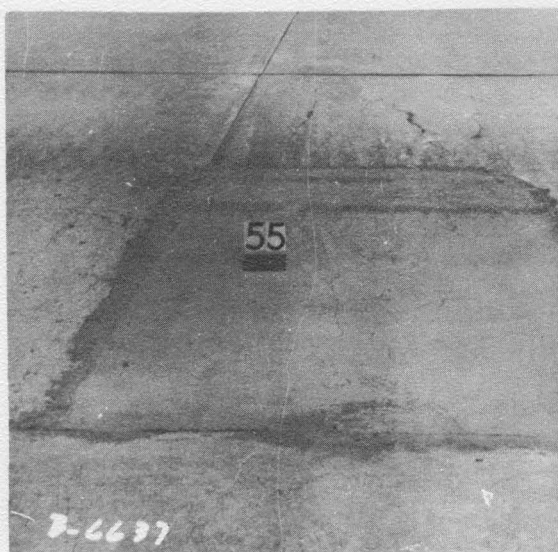
Figure A-6. Repair at Construction Joint. SBL Station 495+
