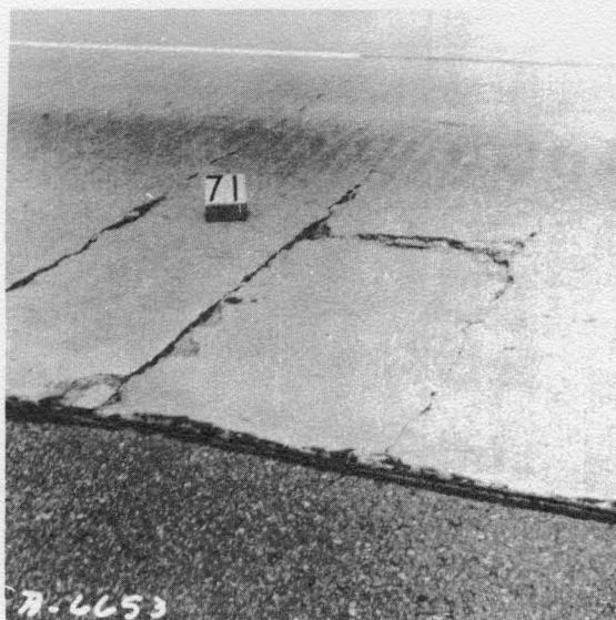
Figure A-23. Failure. NBL Station 419+
