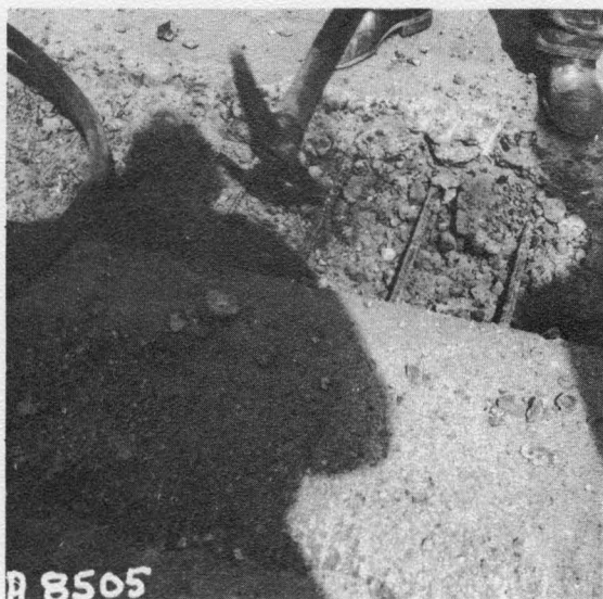
FIGURE B-3 Dry, Sandy Batch of Concrete Below Steel
