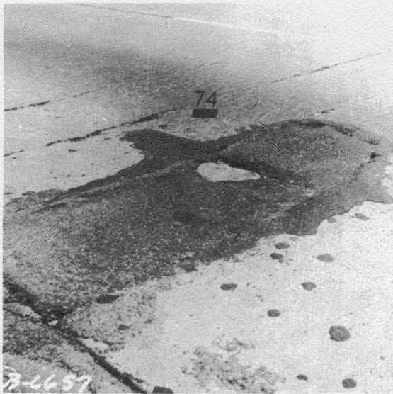
Figure A-27. Repair Area and Failure due to Honey-combing. NBL Station 521+
