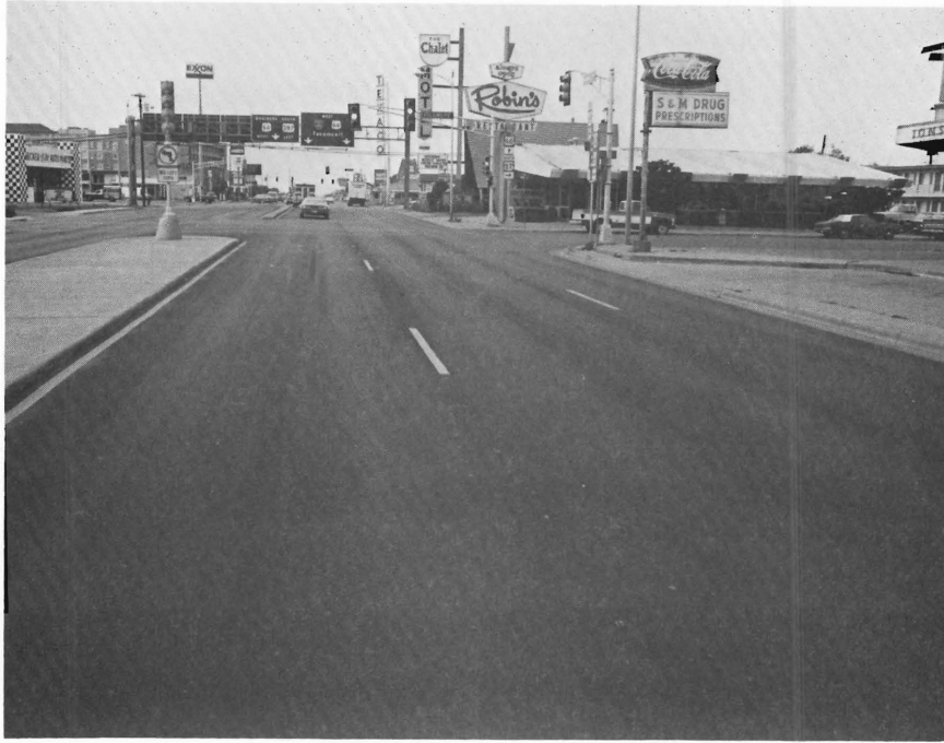
Fillmore Street Without Stabilizing Additive October 1982
