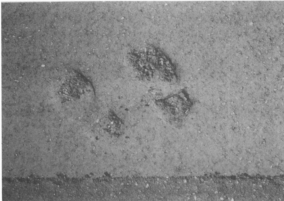
Photograph 8. The uncompacted bottom ash mix displayed a tendency to stick and pull apart when placed in contact with cold, dry objects. A flat wheel roller was used for breakdown rolling. A light coat of diesel prevented the asphaltic concrete pavement from sticking to the roller drum.
