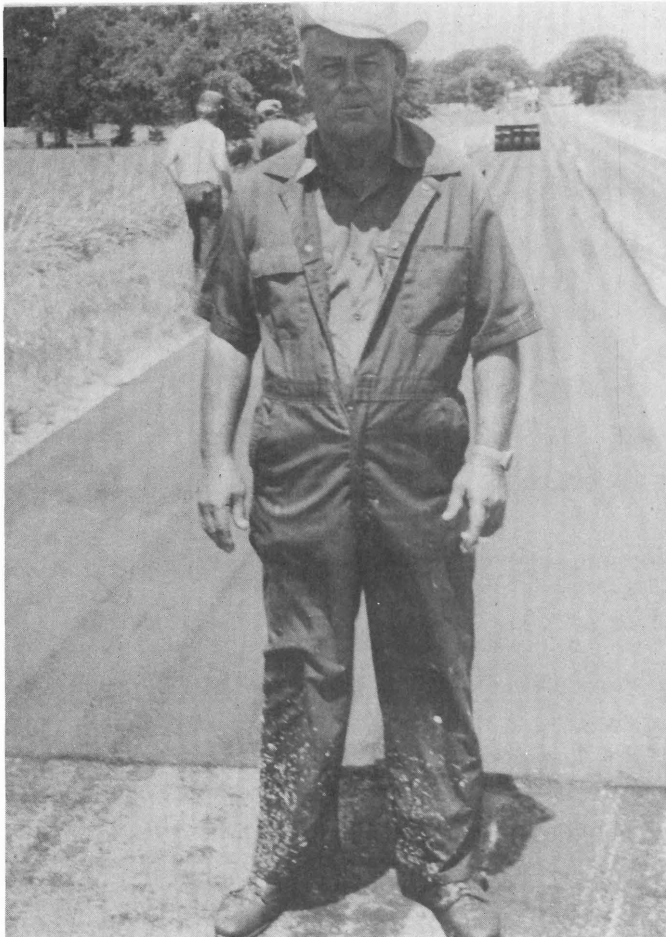
Photograph 20. This RC-2 asphalt is both tacky and sticky, as evidenced by Mr. Bobby Stone's coveralls. The tack coat in the WBL was greatly reduced. To date, there is no noticeable difference in the performance of the two lanes.
