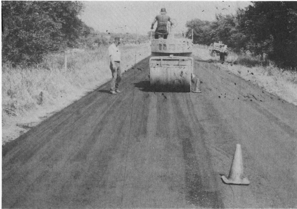
Photograph 9. The bottom ash mix cooled fast and required immediate rolling for proper densification. There was no lateral displacement normally associated with smooth gravel mixes. Mr. Charles Wingfield is monitoring the breakdown rolling for mix pickup.
