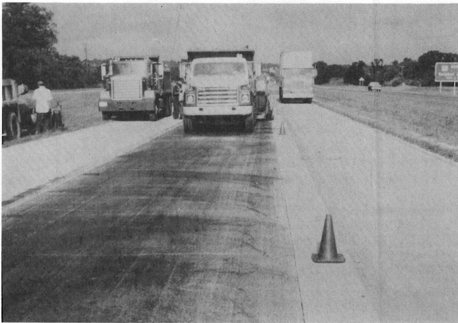
Photograph 22. An 11 percent optimum asphalt content and lighter tack was utilized in this bottom ash test section. There has been no slippage or rutting after 1.5 years service.
