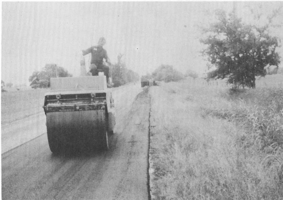
Photograph 18. Flat-wheel breakdown rolling of the bottom ash mix on SH 11.
