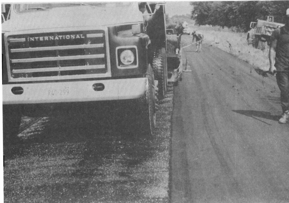
Photograph 7. A heavy tack coat was applied to insure bonding between the existing seal coat and the new bottom ash HMAC. Optimum asphalt content was 10 percent but there was no apprehension about the tack flushing up through the asphalt.
