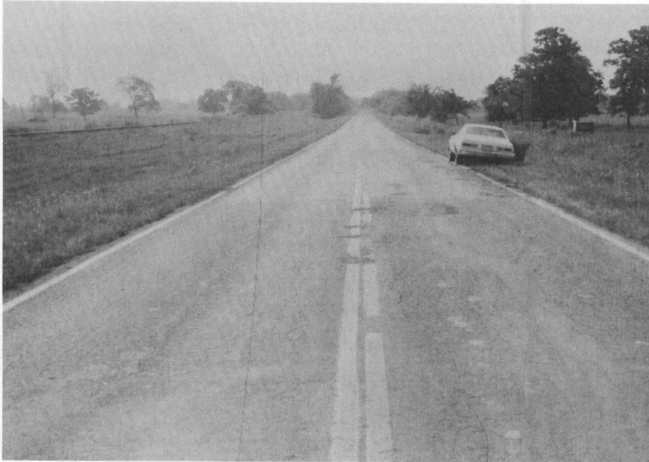
Photograph 13. Overall view of the test section site on SH 11 before overlaying with the bottom ash mix.
