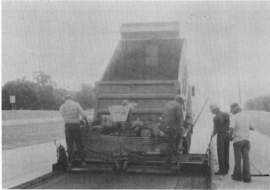
Photograph 23. Laying operations on IH 30 at Sulphur Springs. Maintenance Forces rented the equipment shown.
