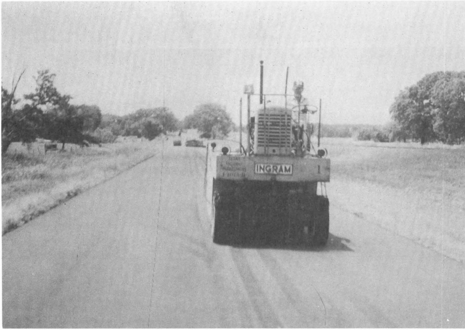
Photograph 19. Mr. Charles Wingfield, Sulphur Springs' Maintenance Forces, operating the pneumatic-tired roller to complete the overlay operation.
