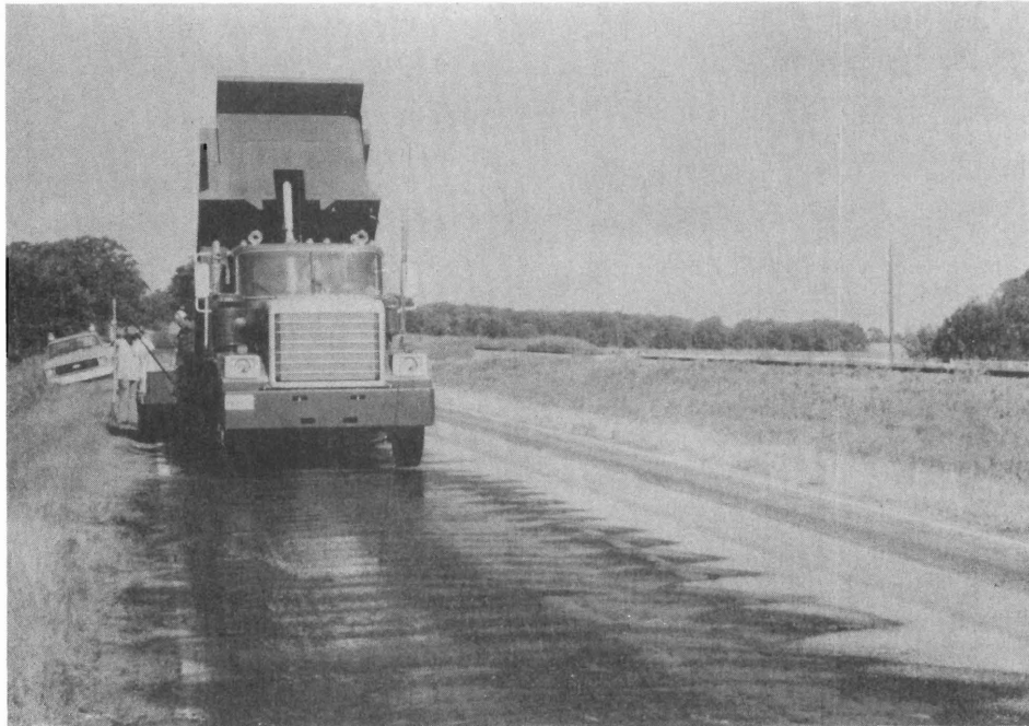
Photograph 15. A heavy hand-sprayed RC-2 tack was used in the EBL of SH 11. Since an optimum asphalt content of 12 percent was selected to hedge against deflection cracking, there was some apprehension about this tack flushing through the compacted bottom ash mat. This has not occurred to date.
