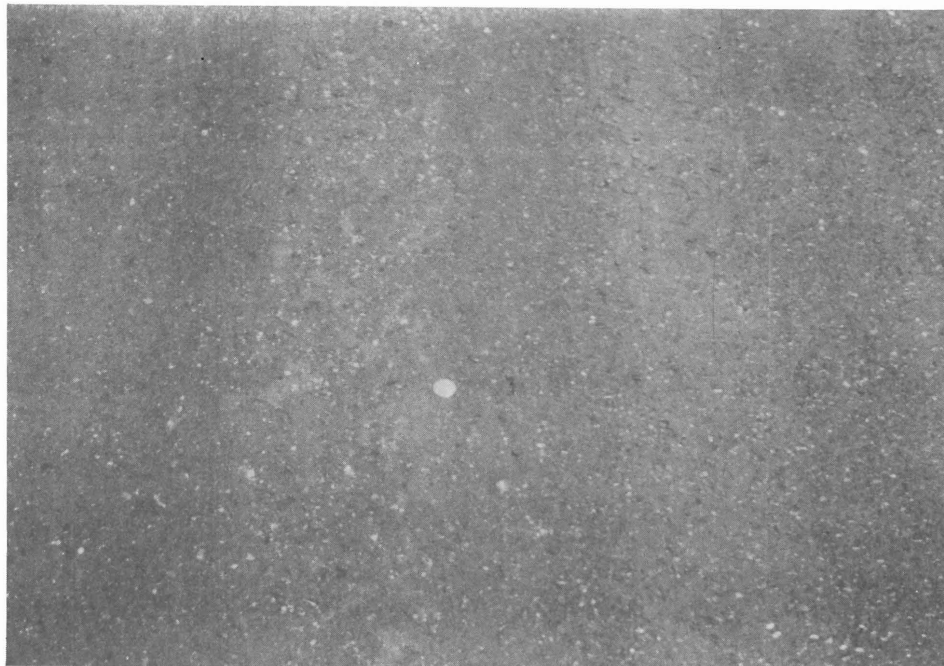
Photograph 28. Close-up view of the compacted bottom ash-gravel mat.
