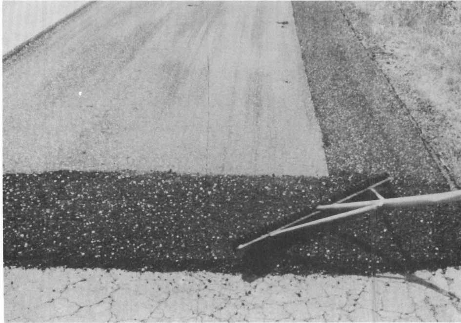
Photograph 17. There was some concern about being able to rake this high-friction bottom ash mixture. This tapered start was hand-constructed without difficulty.
