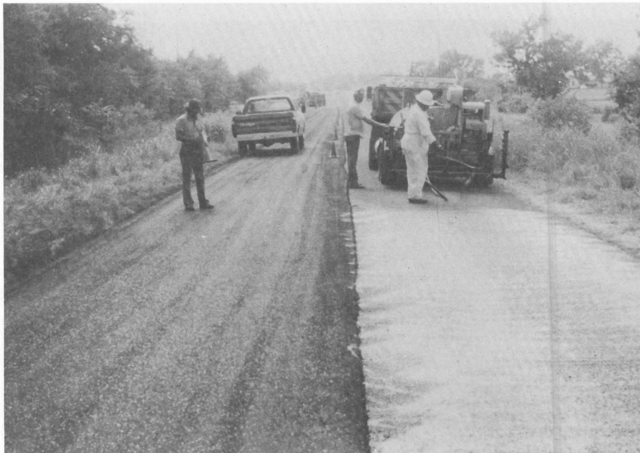
Photograph 6. An RC-2 tack coat was applied by the Sulphur Springs' Maintenance Forces, who are under the immediate supervision of Mr. Walter B. Darling.
