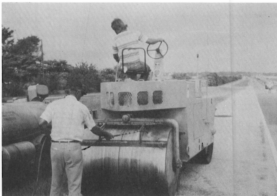
Photograph 26. A light coat of diesel being applied to the flat-wheel roller by Mr. Charles Wingfield prior to the breakdown rolling. This prevents pickup of the bottom ash-gravel asphaltic concrete pavement.
