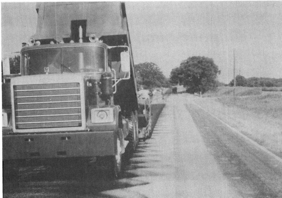
Photograph 16. Depicts the ability of the bottom ash mix to be placed in neat lines.
