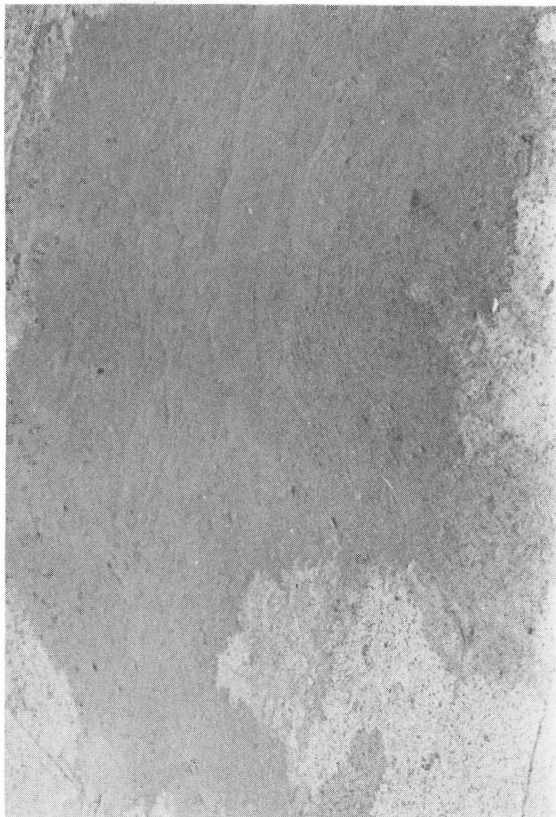
Figure 2 - Cracks Repaired by Brooming (Area No. 5)
