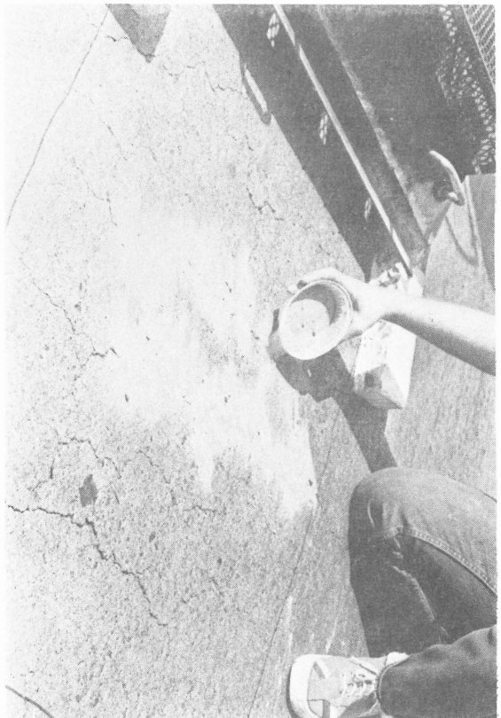
Figure 1 - Cracks Being Repaired Individually (Area No. 1)
