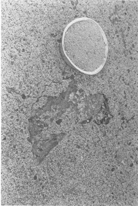
a) Before Patching
