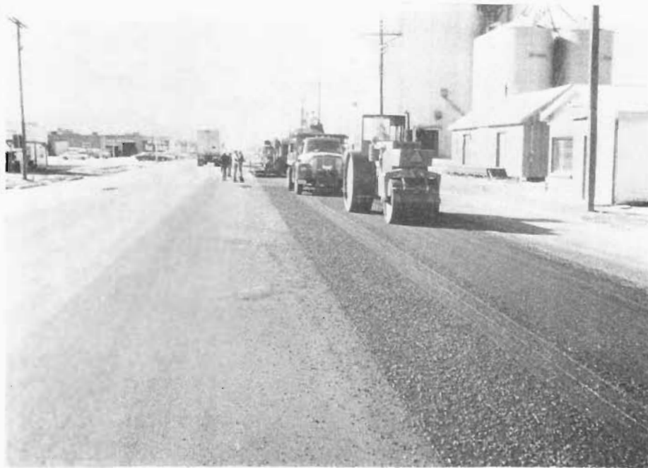
Knockdown Rolling With Steel Wheel And Sealing with Pneumatic Tire Roller
