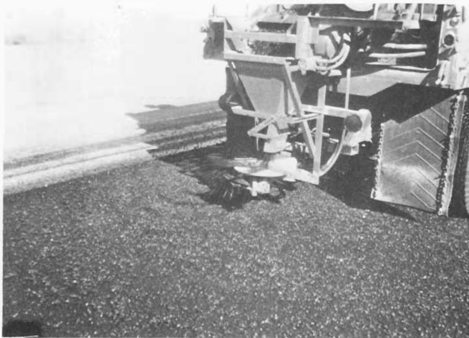
Placing Sprinkle Aggregate
